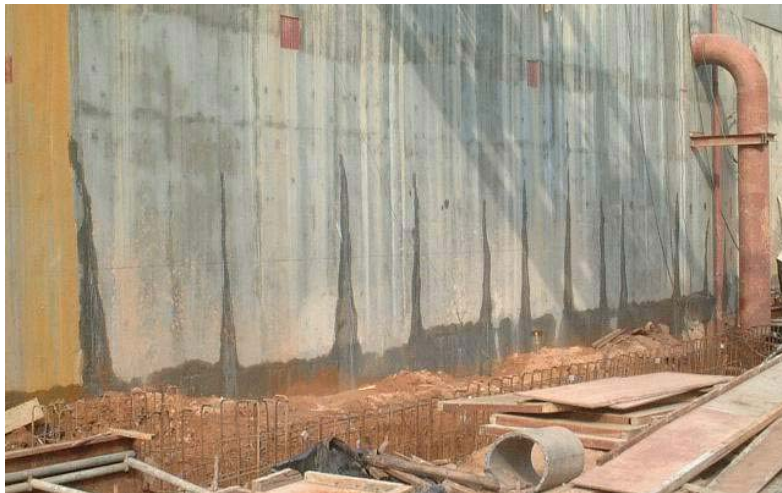
Fig. 10.23 Typical thermal and shrinkage cracks in a large reservoir structure
