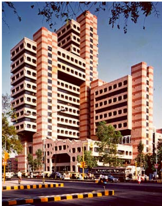
Fig. 1.2 A modern reinforced concrete multi-storeyed building — one of the tallest in New Delhi (102 m) : Jawahar Vyapar Bhavan [Architects : Raj Rewal and Kuldip Singh , Project Consultants : Engineers India Limited ]. Structural concept : joist floor supported on Vierendeel girders (arranged in a ‘plug on’ fashion), cantilevered from core walls.
