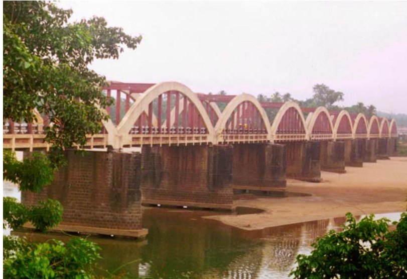
Fig. 1.5 A reinforced concrete bow-string girder bridge spanning across the Bharathapuzha River at Kuttippuram, Kerala
