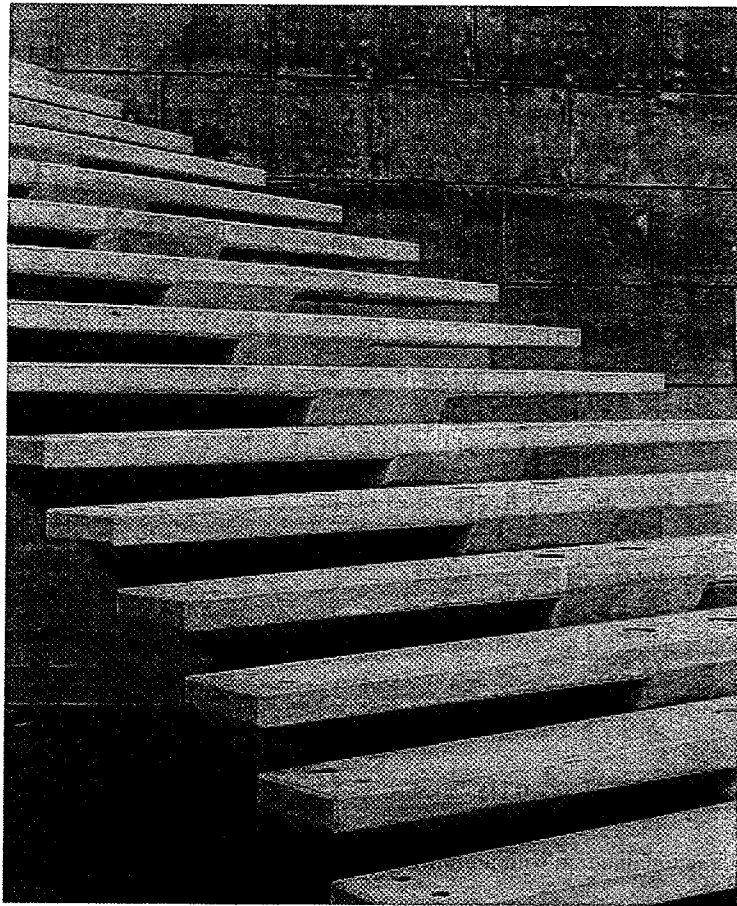
Photo 5.6 Cantilever stairs from a middle beam
