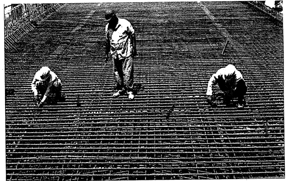
Photo 1.3 Preparation of reinforcement of solid slabs
