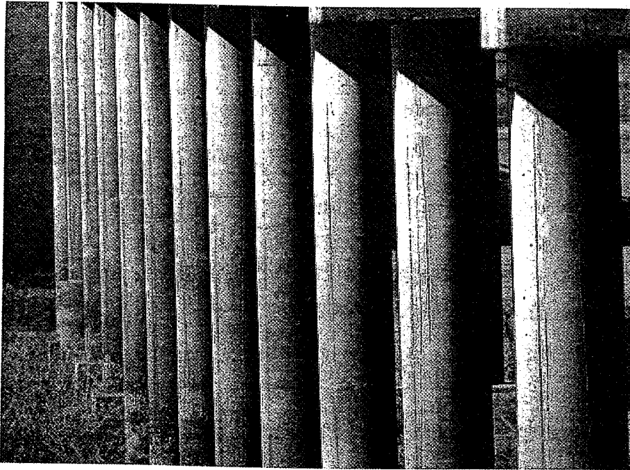
Photo 6.5 Circular reinforced concrete columns supporting a bridge
