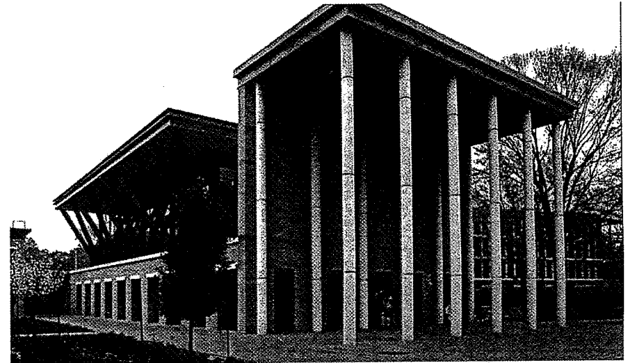
Photo 8.1 Unbraced slender columns at Rice University, USA.
