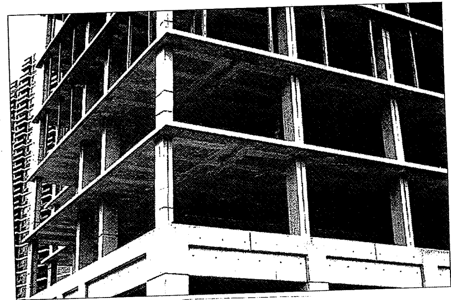
Photo 4.1 Flat slab system
