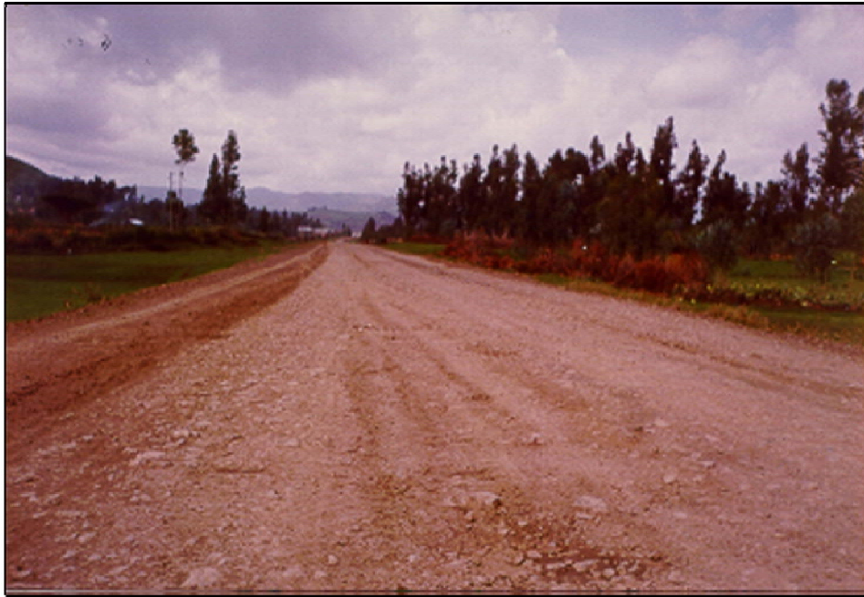
Figure 5-4: Flat Terrain; Flat Roadway Alignment
