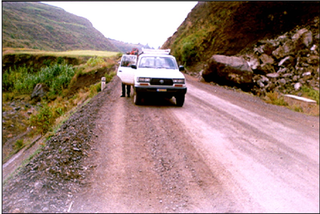
Figure 5-8: Mountainous Terrain; Flat Roadway Alignment
