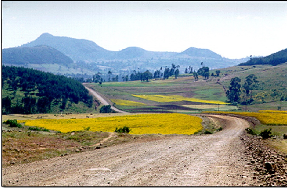
Figure 5-6: Rolling Terrain; Flat to Rolling Roadway Alignment
