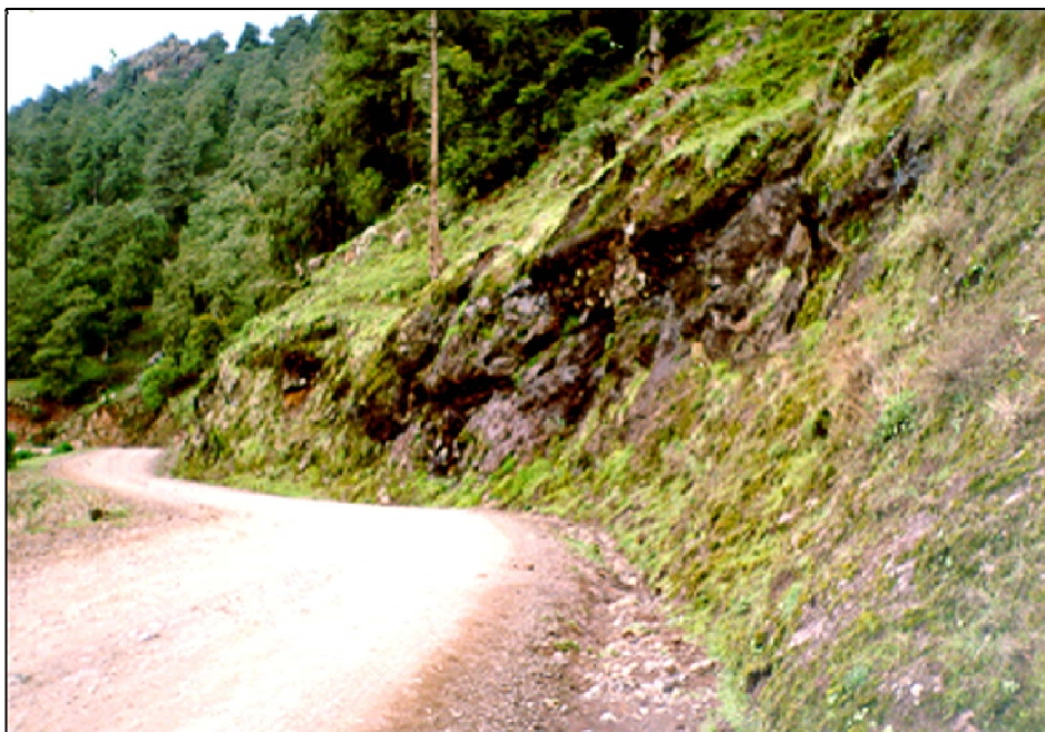
Figure 5-11: Escarpment Terrain; Escarpment Roadway Alignment
