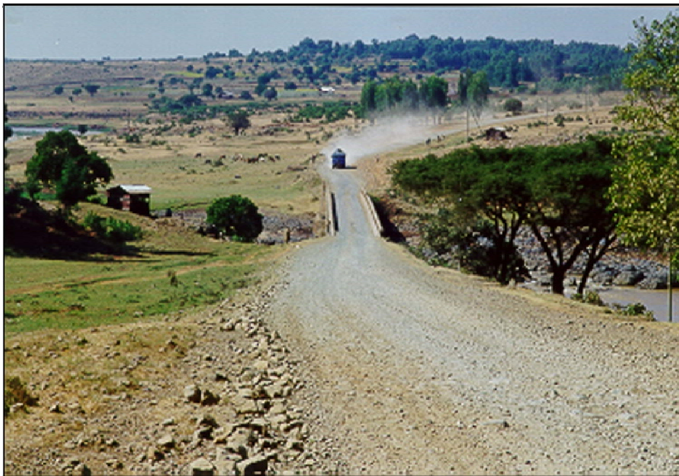
Figure 5-7: Rolling Terrain; Rolling Roadway Alignment
