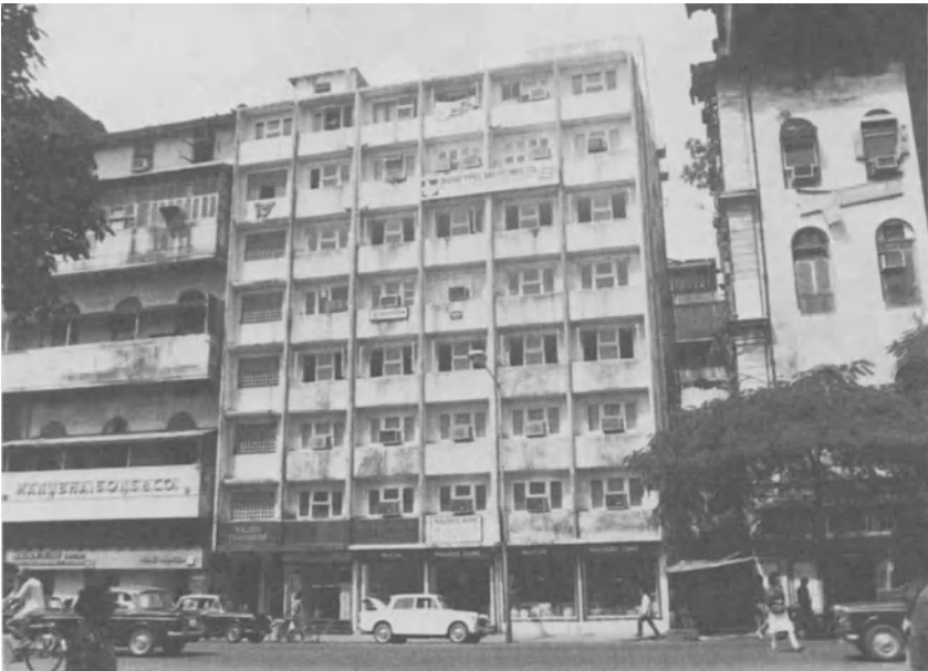
Fig. 2 The current building codes of Bombay permit a FAR of 1.33. A situation is created whereby the owners or developers with the help and cooperation of the occupants, maneuver and manage to maintain the old FAR under the guise of repairs-cum-renovation. The illustration shows a reconstructed 'old' building. The old higher floor height of 4.3 m (14 ft) or so is also used to advantage by subdividing it into two floors, providing the developer a FAR of 7 or 8 against the permitted 1.33 and old existing FAR of 4 or so. Permission for taller buildings of the same or slightly higher FAR than existing built up area, leaving adequate open spaces, would be a desirable and practical proposition.
