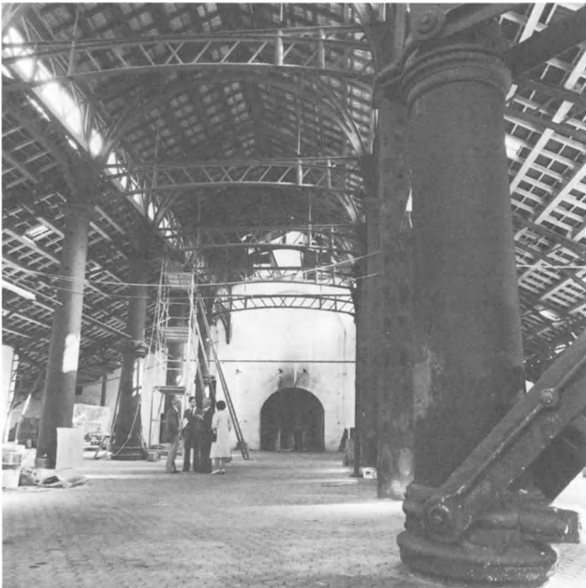
Fig. 3 Foundry Hall, Sayner Hütte, West Germany, 1830
