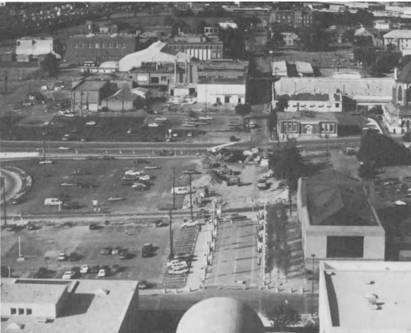
Fig. 4 Construction photo shows Flora Street beginning to take form in front of the new LTV Center
