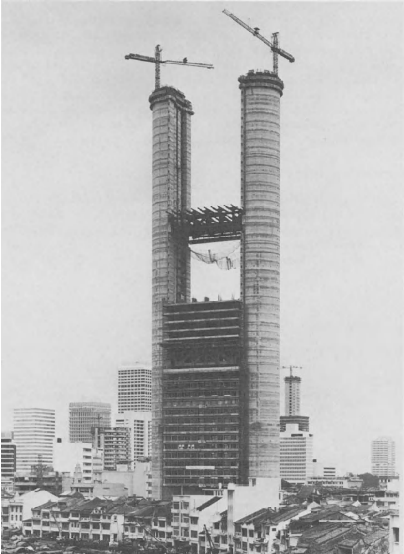
Fig. 5 OCBC Bank, Singapore—transfer girder shown during construction
