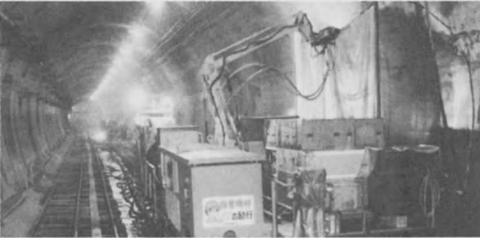
Fig. 25 Abrasive jet-cutting robot ( Kajima )
