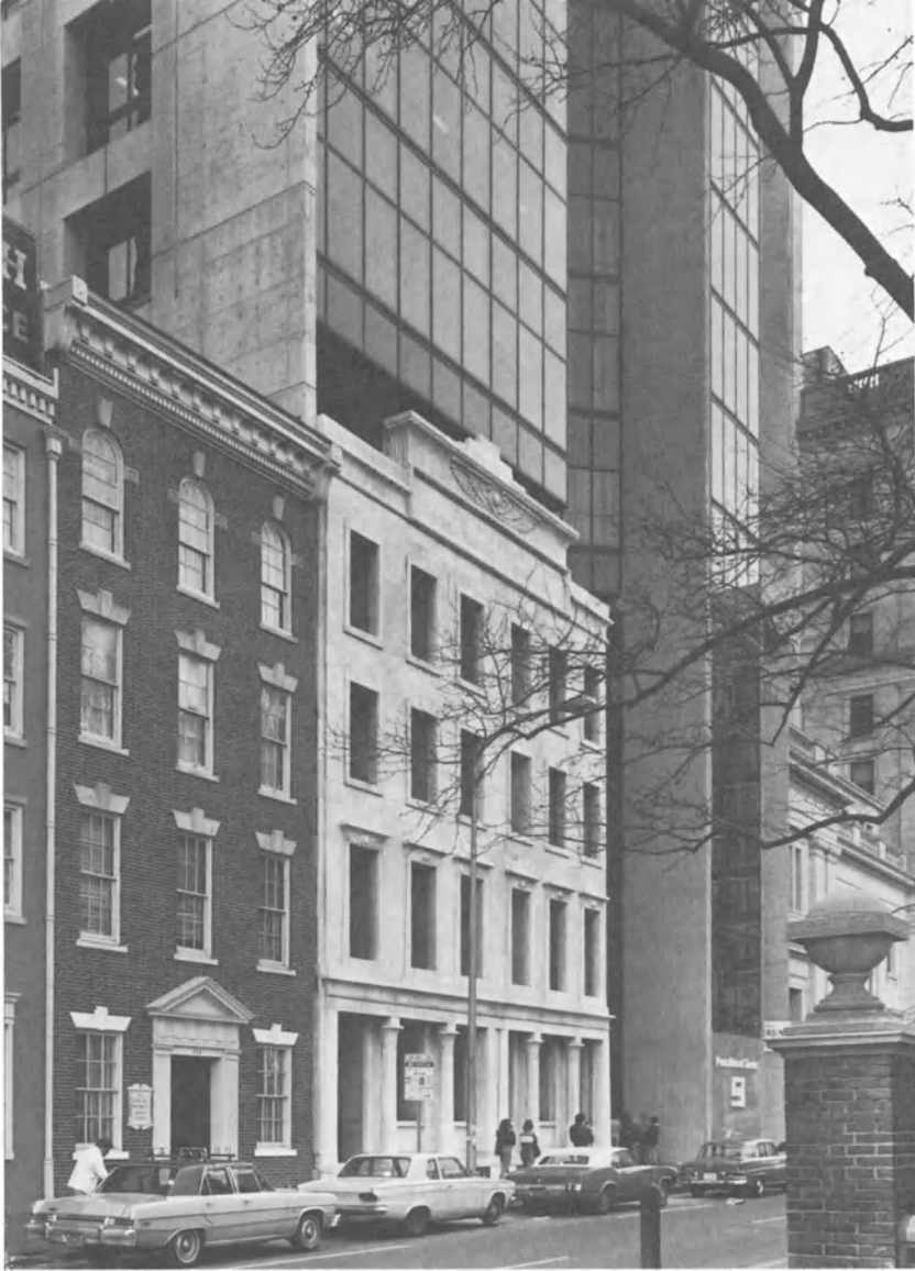
Fig. 2 Penn Mutual Tower incorporating the 1835 Haviland facade (Photo by Rollin LaFrance)
