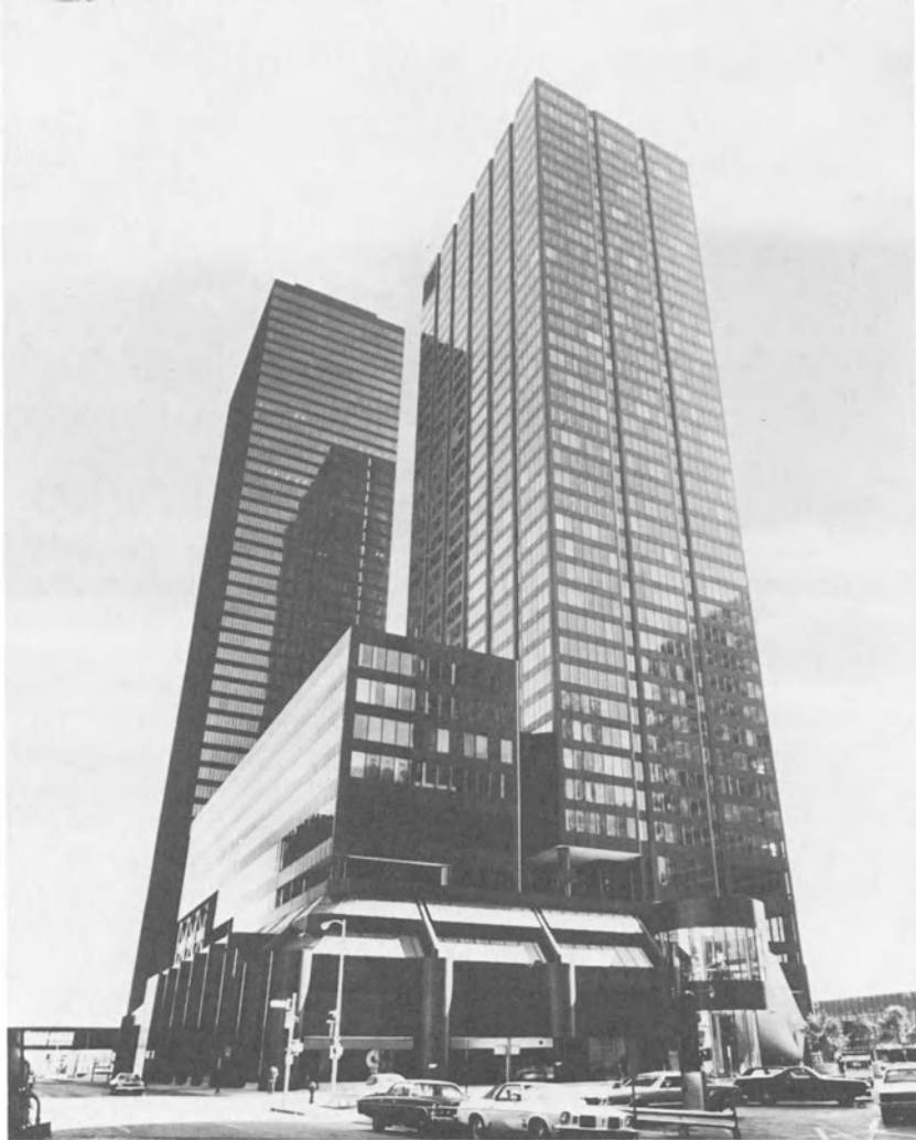
Fig. 1 Houston Center, Houston, Texas (Courtesy: Walter P. Moore and Associates)
