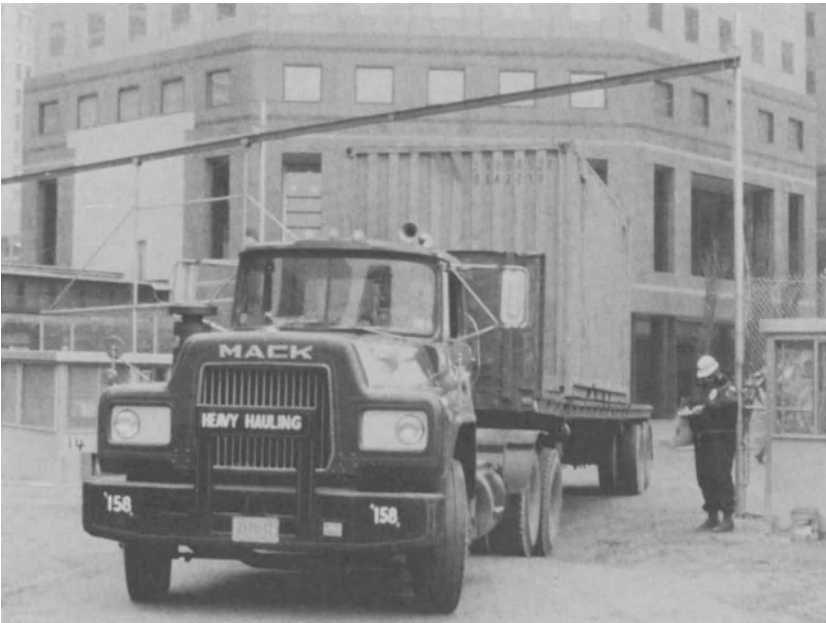
Fig. 11 Deliveries to the site
