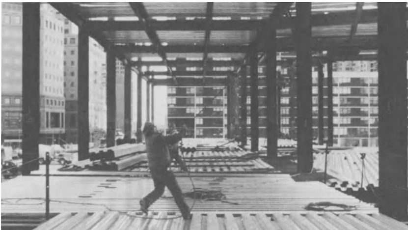
Fig. 12 Construction of steel-framed tall building
