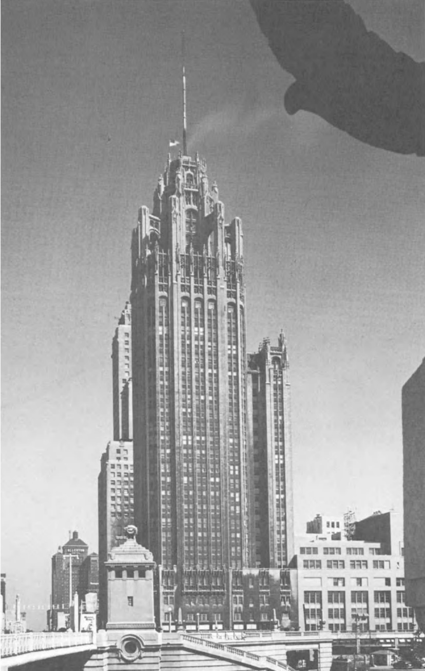
Fig. 6 Tribune Tower (Photo by Hedrich Blessing)
