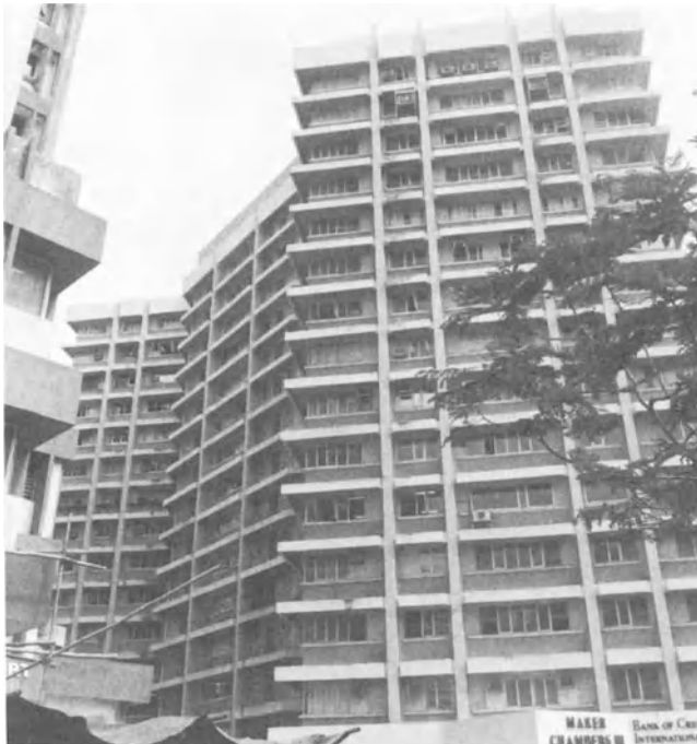
Fig. 4 A commercial high-rise in South Bombay. The elevation treatment relies heavily on sun-breaking devices such as continuous horizontal overhangs above windows intercepted by vertical fins. Numerous window air-conditioners can be seen.
