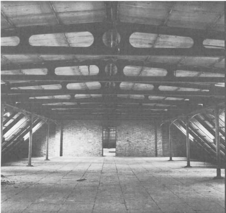
Fig. 2 Quadrangle Store roof
