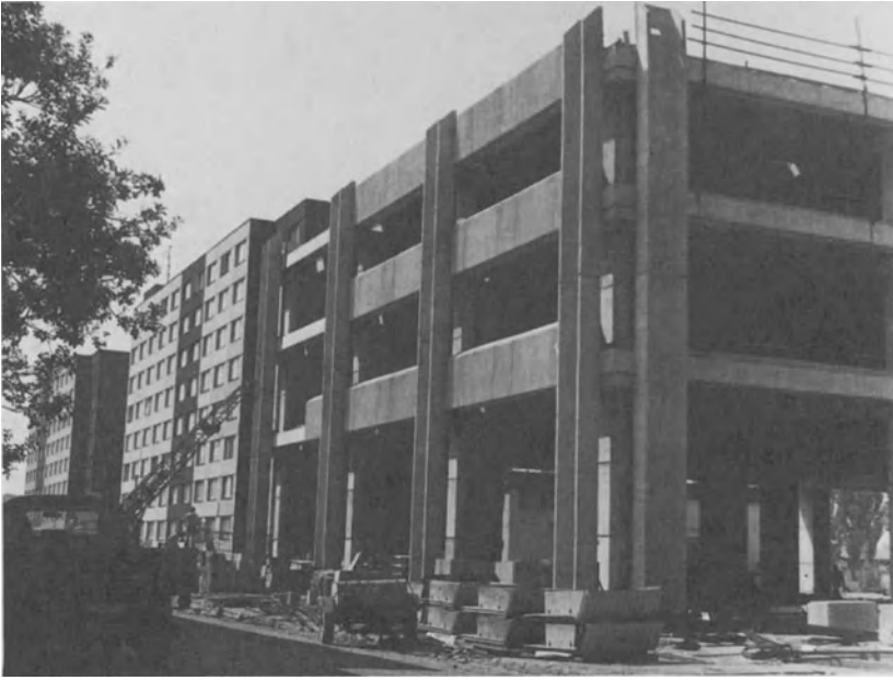
Printing house under construction in Prague
