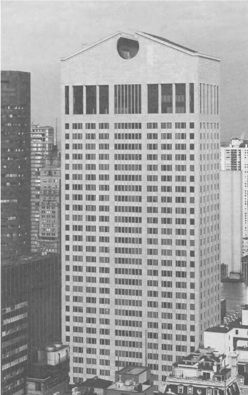
Fig. 1 AT&T Corporate Headquarters
