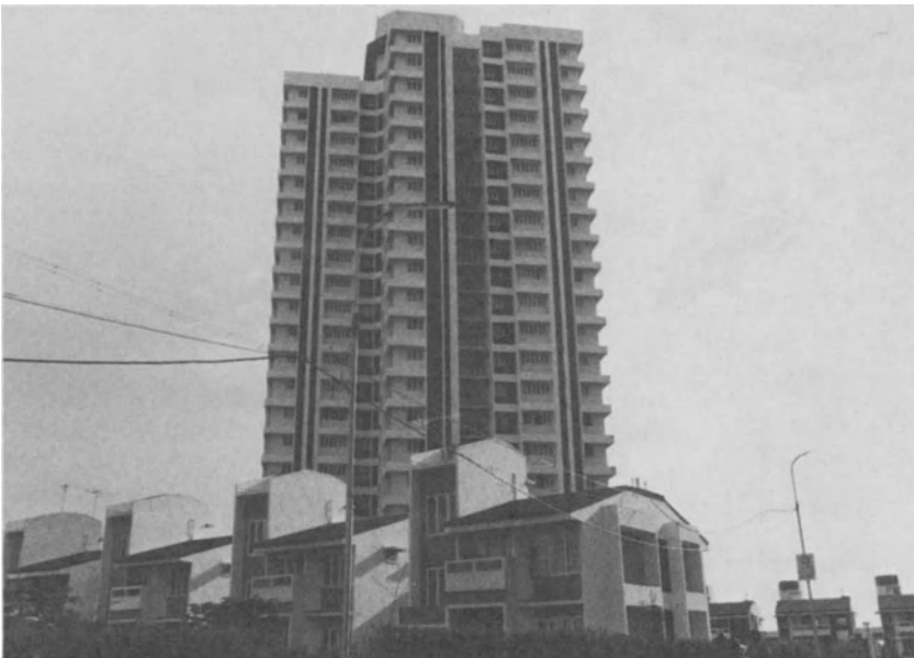
Fig. 1 High-rise buildings in suburban areas in a city like Bombay with a low FAR of 1.00 create space for semiprivate bungalows or row-houses.
