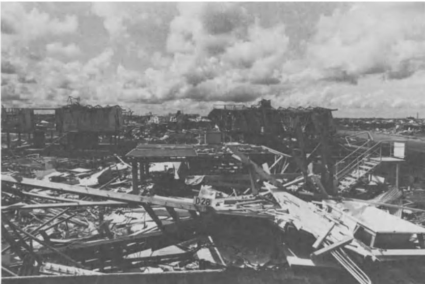
Fig. 5 Debris produced by cyclone Tracy in Darwin, NT, Australia (1974)
