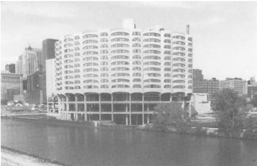
Fig. 1 River City is a mixed-use predominantly residential project on the south edge of Chicago's office core (Photo by Stephen Roman; Courtesy: City of Chicago)
