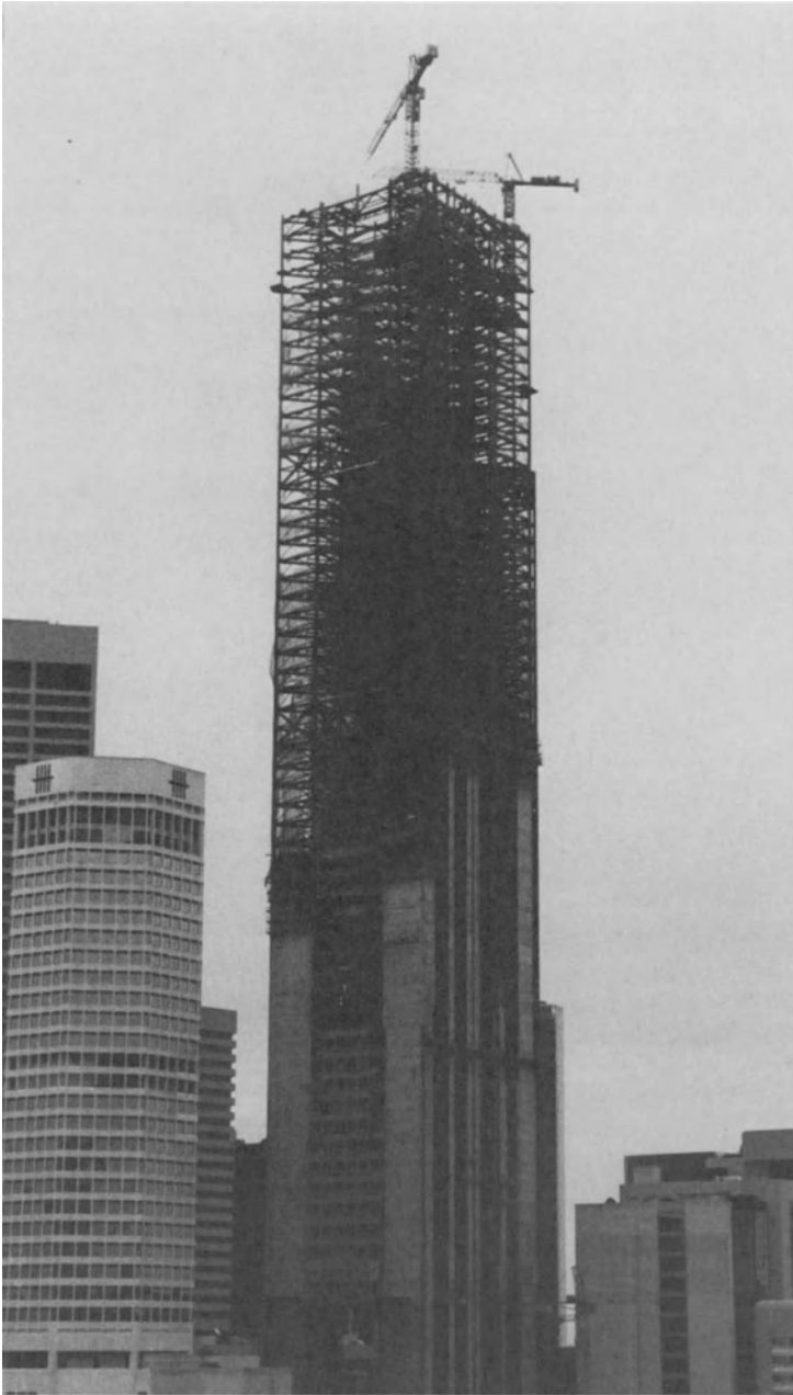
Fig. 1 Final stage of steel erection on OUB Centre
