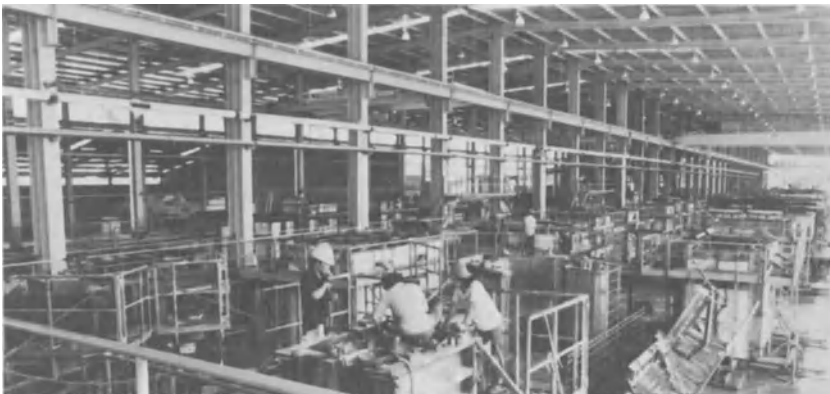
Fig. 3 Precasting factory showing volumetric molds
