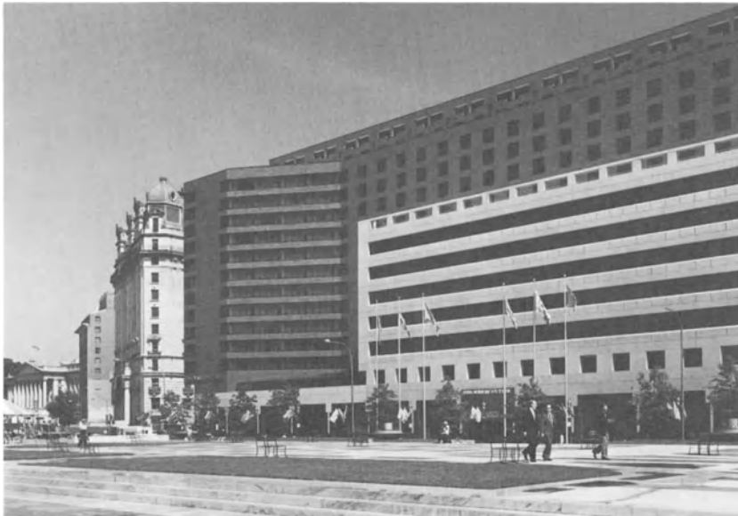
Fig. 4 The National Place project on Pennsylvania Avenue (Photo by Tom Crane)
