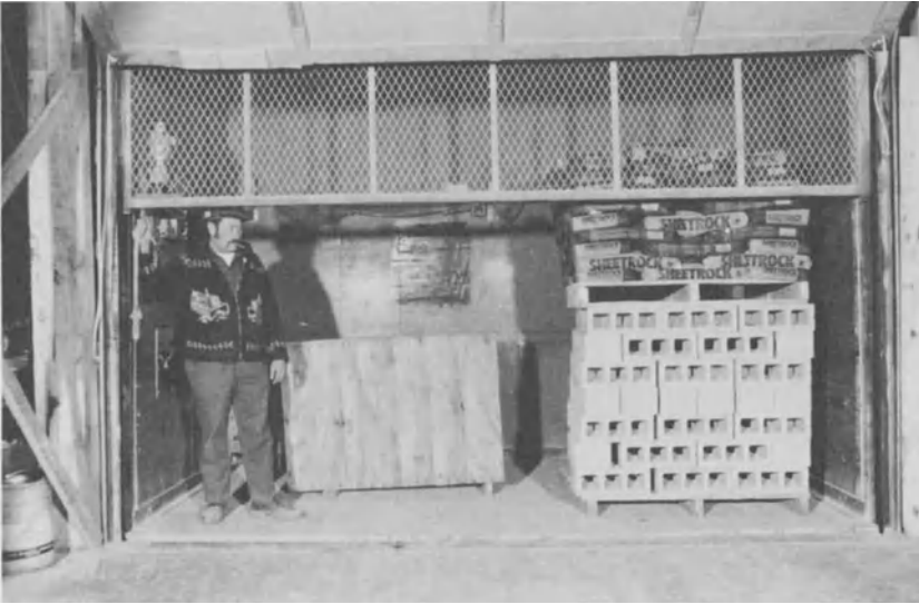
Fig. 5 Internal construction elevators
