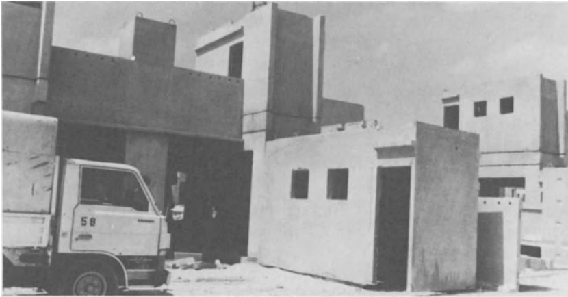
Fig. 2 Complete volumetric units ready for erection
