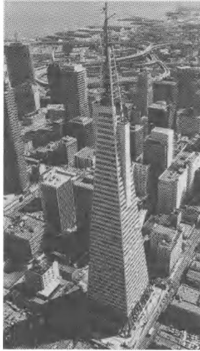
Fig. 18 Transamerica Building during construction (1972) (Courtesy: Chin and Hensolt.)
