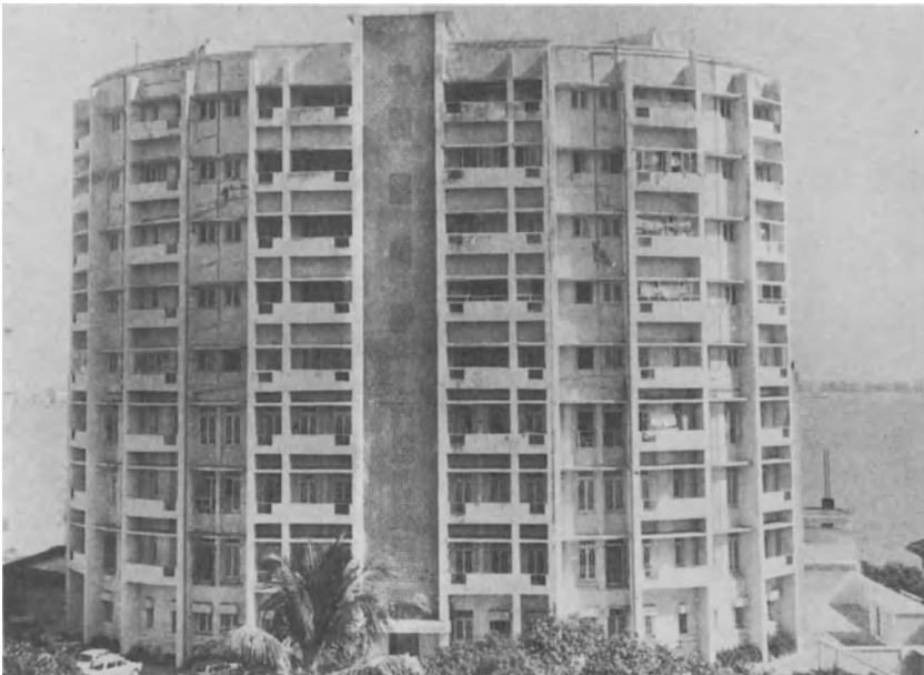
Fig. 6 The Panorama building in Bombay is an interesting conversion from low-rise to high-rise. On an existing 4 story tall building (constructed in 1935-1937), 5 more floors were added in 1966-1967. (The building is named Panorama because it commands a panoramic view of Bombay city, being located at a high point.)
