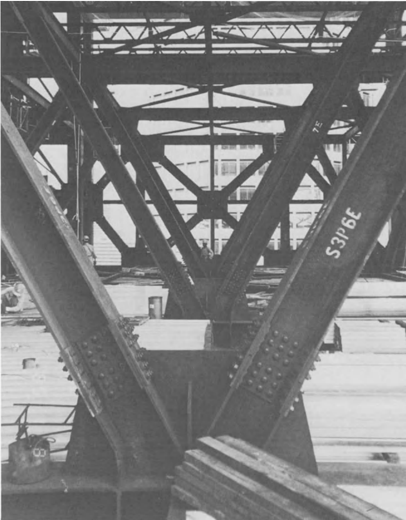
Fig. 7 Outrigger trusses
