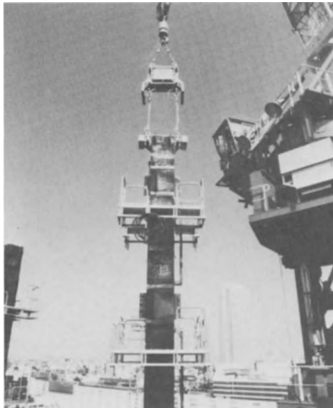
Fig. 33 Auto clamp placing a steel column ( Ohbayashi Gumi )
