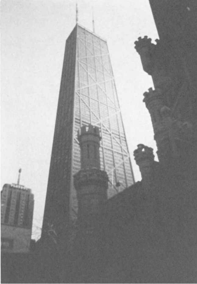
Fig. 24 John Hancock Center ( Photo by Hedrich-Blessing )
