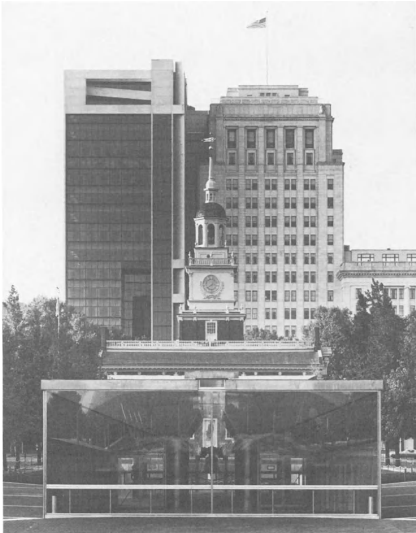
Fig. 1 Penn Mutual Tower with Independence Hall and the Liberty Bell Pavilion in the foreground (Photo by Rollin LaFrance)
