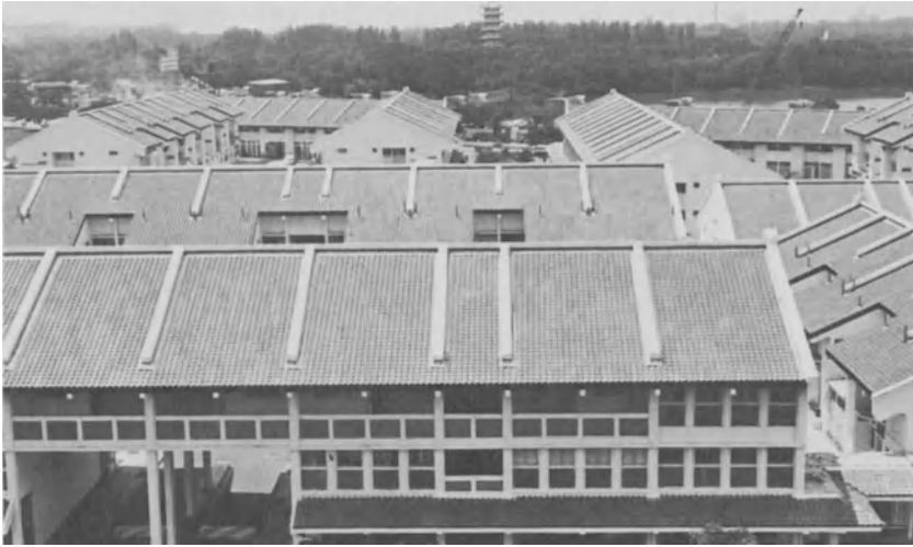
Jurong East Neighborhood Center—design with a 'Chinese village' flavor in response to the context of the adjacent Chinese Garden
