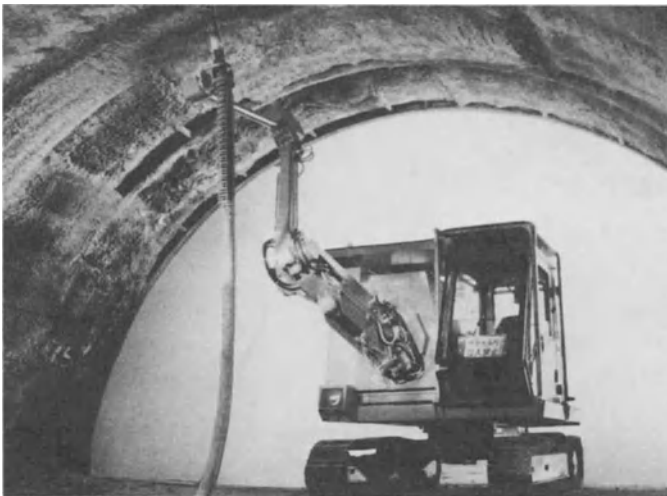
Fig. 24 Automatic concrete sprayer ( Kobe Steel )
