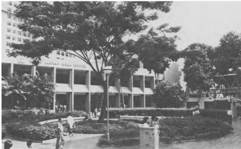
Bukit Merah Town Center. Introduction of natural landscape provides shade and softens the impact of the intense urban development
