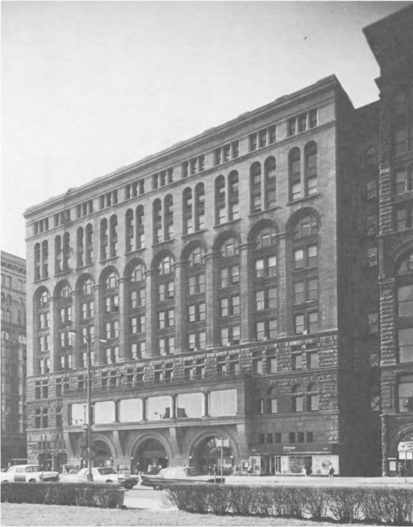
Fig. 2 The Auditorium, built in 1899, designed by Louis Sullivan (Photo by Hedrich Blessing)
