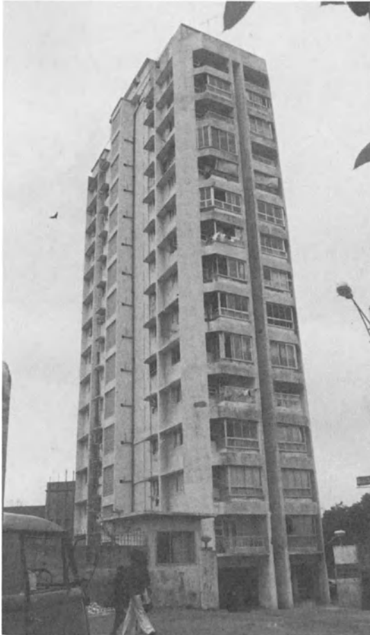
Fig. 1 A typical suburban high-rise. There are numerous such slim high-rise buildings all over Bombay, almost all of which have a nominal built up area of 250-400 m 2 (2700-4300 ft 2 ) per floor.
