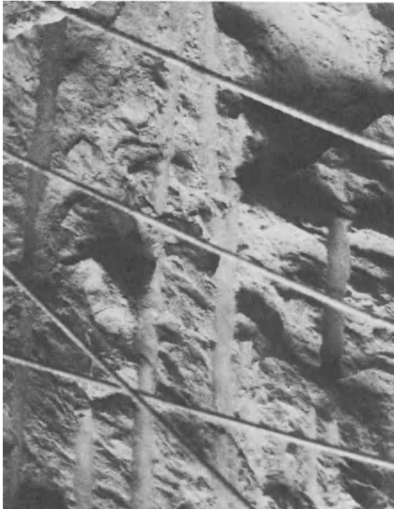
Fig. 5 Drilled and blasted rock face
