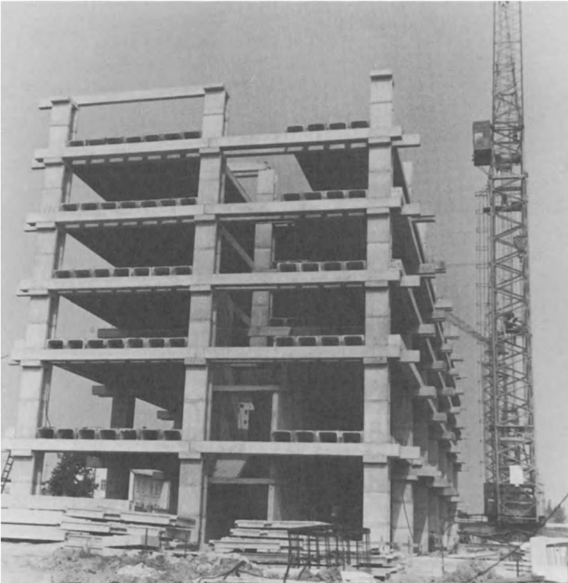
Multistory industrial building TESLA in Vrable—under construction
