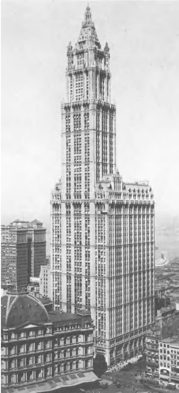
Fig. 2 Woolworth Building (Courtesy: Library of Congress)
