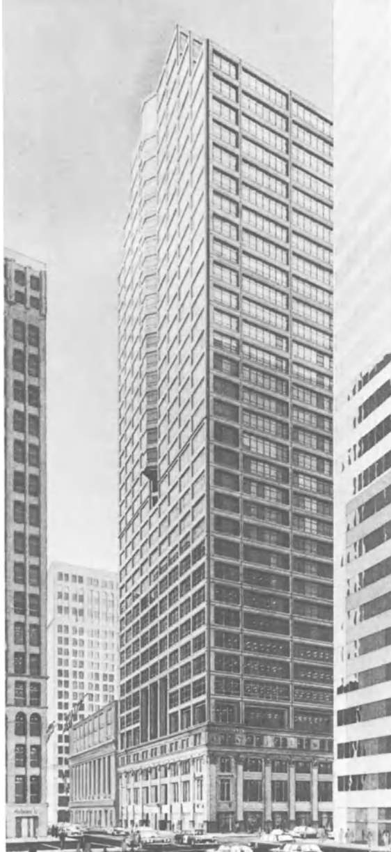
Fig. 2 Manufacturer's Hanover Plaza employs contextual design in enhancing its place in the LaSalle Street financial corridor (Photo by Fidinem USA; Courtesy: City of Chicago)
