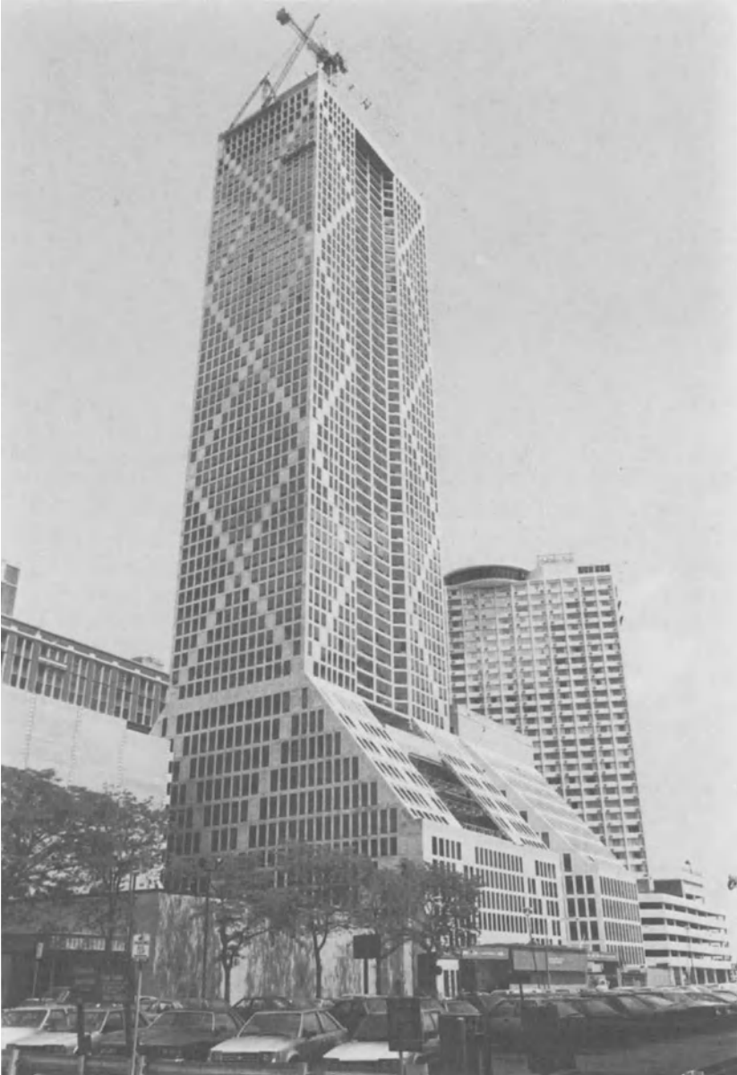
Onterie Center, a mixed-use high-rise in Chicago
