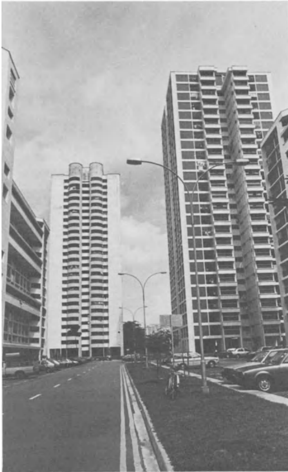
Delta Avenue. Variations on a theme provide visual relief to avoid the sense of monotony in a high-rise high-density development
