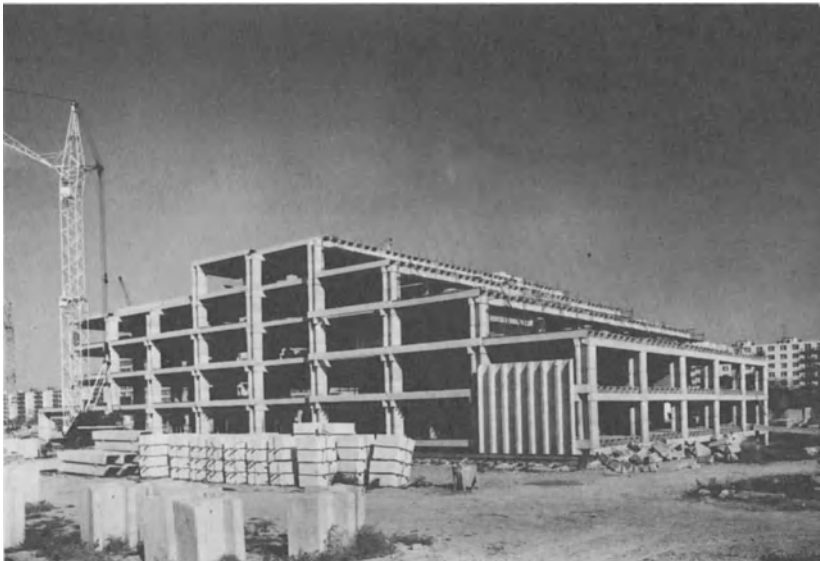
Multiuse department store ZOD Ruzinov in Bratislava under construction
