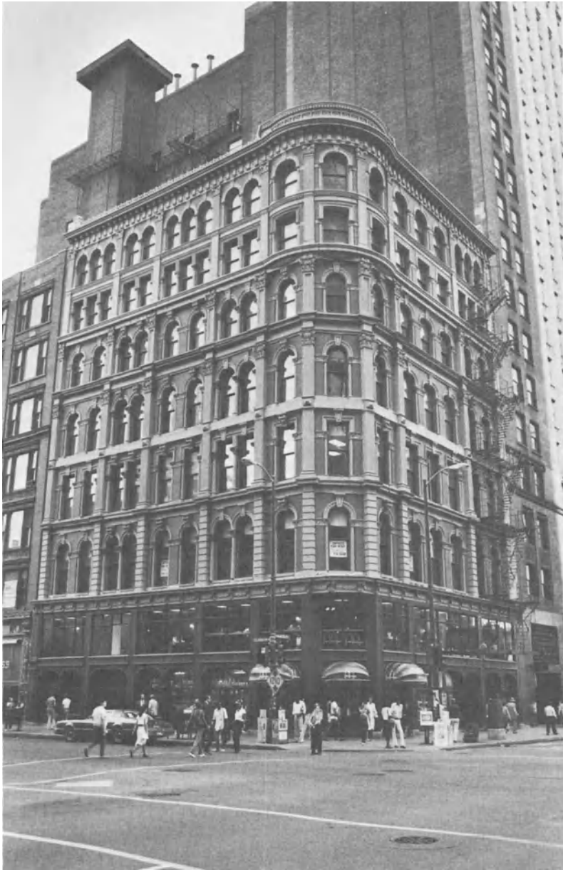
Fig. 1 Delaware Building, built in 1874, survived the Chicago fire (Photo by Steven A. Herrlin)
