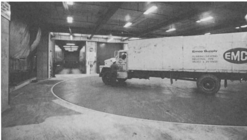
Fig. 6 Truck on turntable is being aligned with basement loading dock
