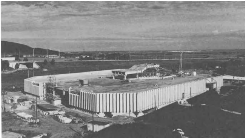
Cladding of Lamac commercial center, Bratislava
