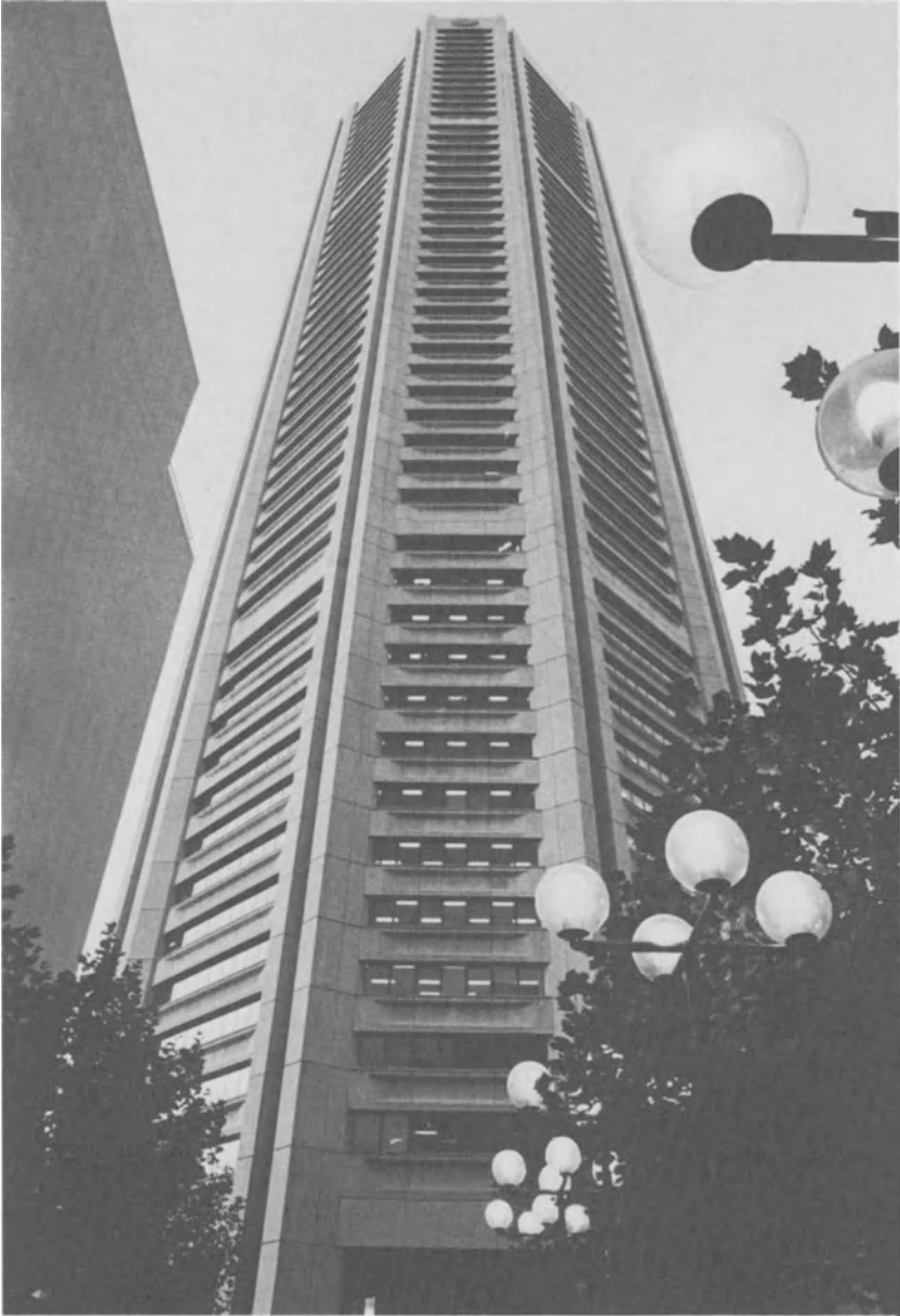
Fig. 4 Nuru House—total precast facade
