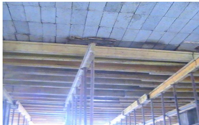
Fig. 5.10.5 Formwork for slabs
