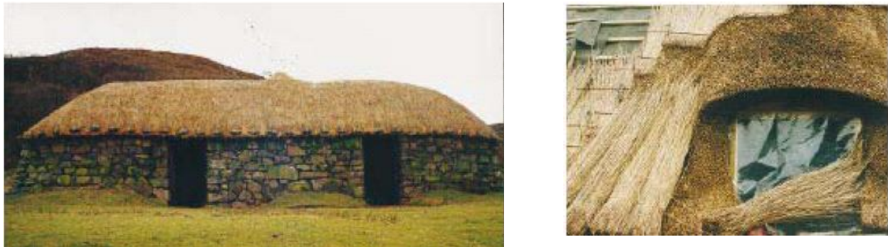
Fig. 5.6.16 Thatch roof covering
