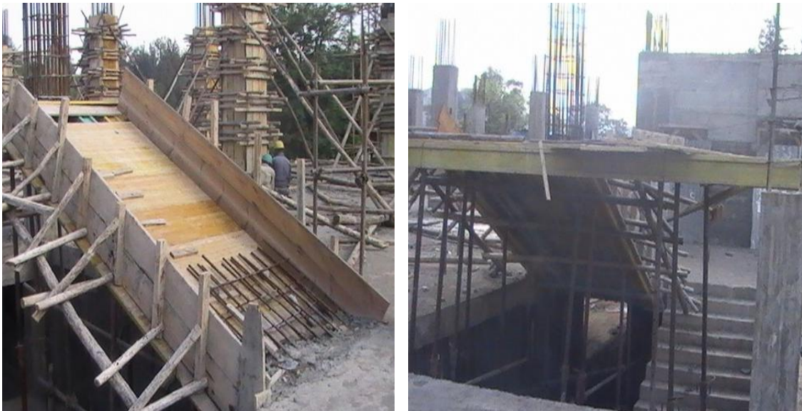
Fig. 5.10.7 Formwork for stairs
