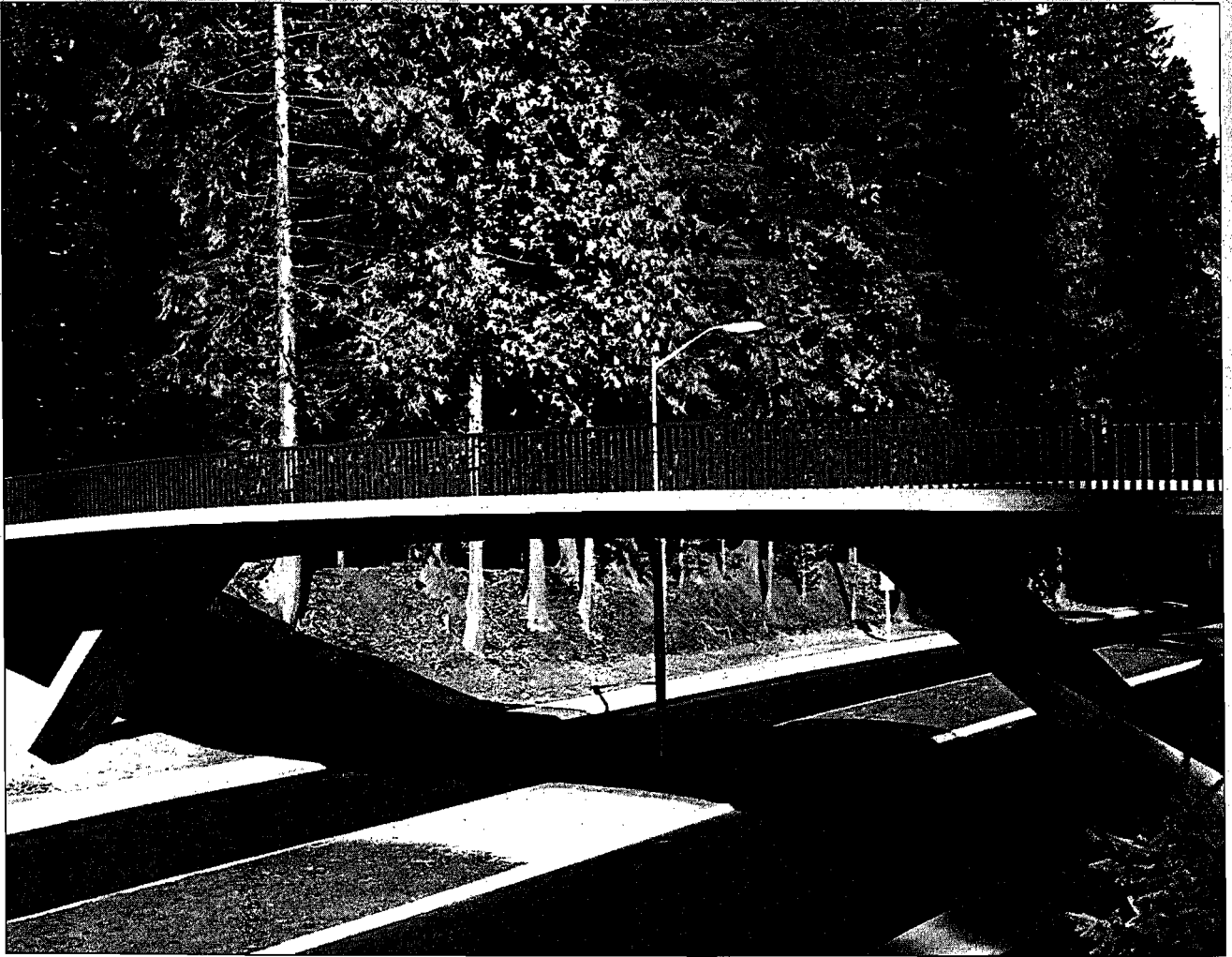
East Bay Drive, a post-tensioned concrete frame bridge, 146 ft long, mainspan 60 ft, edge of concrete girder 7 in thick.
