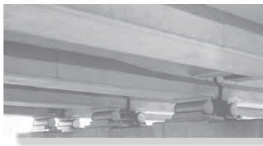
Rollers and associated bearing pads are used to support the prestressed concrete girders of a highway bridge.
