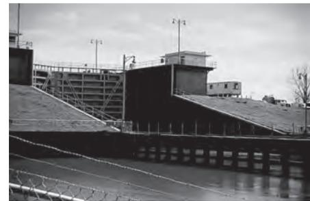
The design of this retaining wall requires estimating the soil pressure acting on it. Also, the gate of the lock will be subjected to hydrostatic pressure that must be considered for its design.
