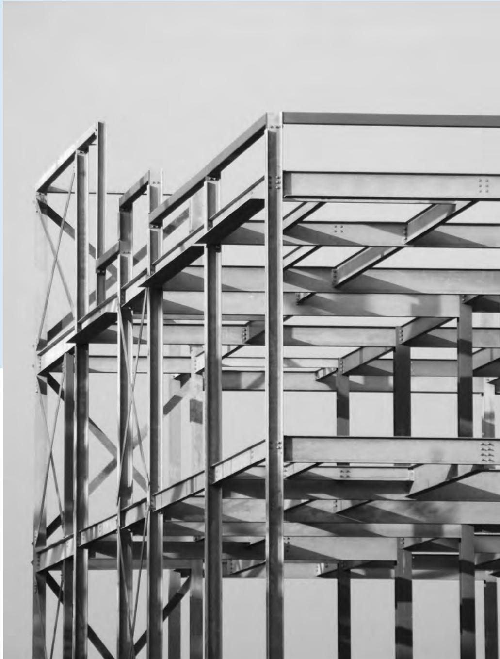
Oftentimes the elements of a structure, like the beams and girders of this building frame, are connected together in a manner whereby the analysis can be considered statically determinate.
