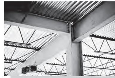
The two girders and floor beam are assumed to be pin connected to this column.
