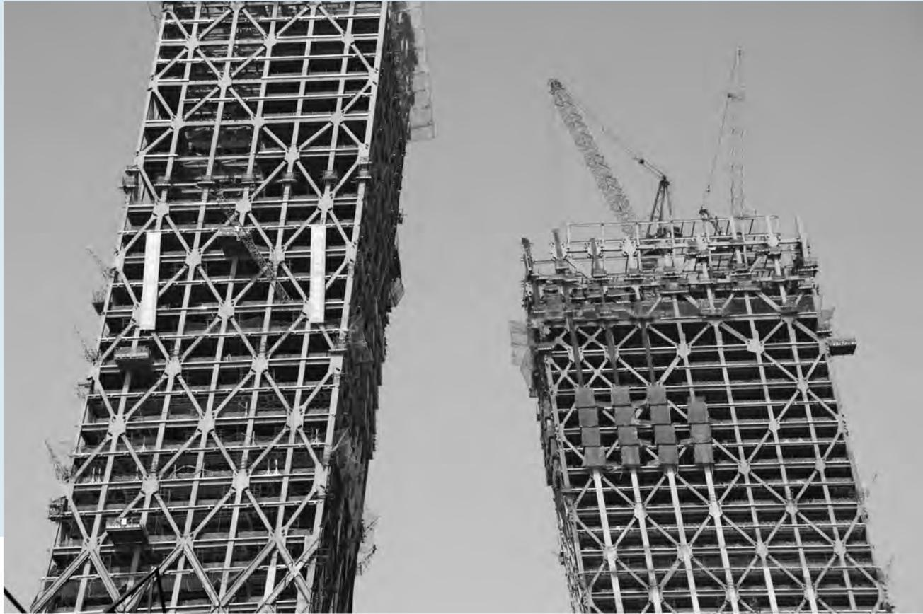
The diamond pattern framework of this high-rise building is used to resist loadings due to earthquake or wind.
