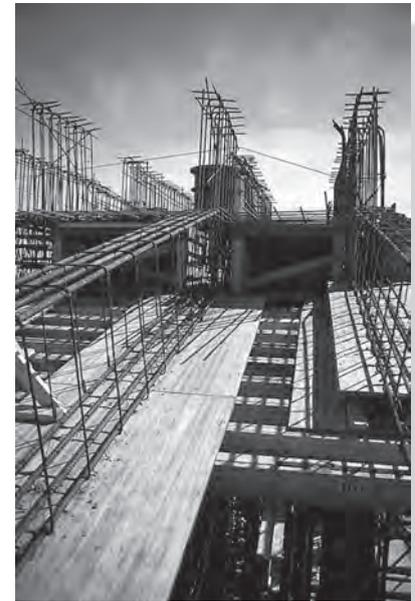
The steel reinforcement cage shown on the right and left is used to resist any tension that may develop in the concrete beams which will be formed around it.
