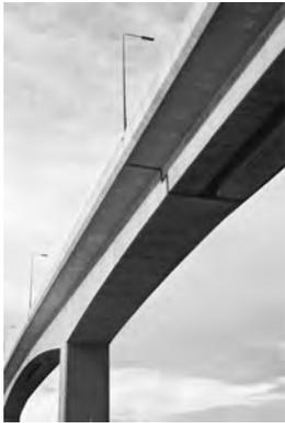
The deck of this concrete bridge is made so that one section can be considered roller supported on the other section.
