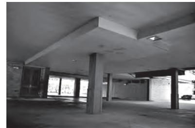
Shown is a typical example of an interior building column. The live load office floor loading it supports can be reduced for purposes of design and analysis.
