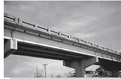
The prestressed concrete girders are simply supported and are used for this highway bridge. Also, note the tapered beams used to support these girders.
