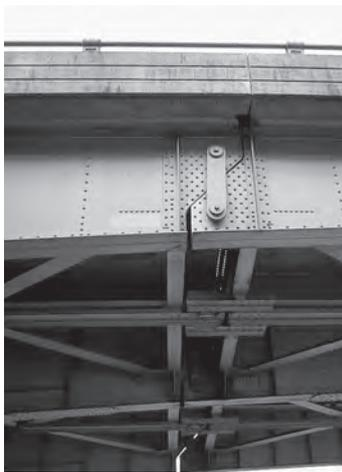
The short link is used to connect the two girders of the highway bridge and allow for thermal expansion of the deck.
