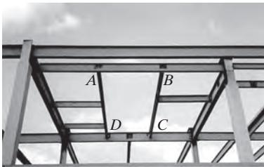
The flat roof of the steel-frame building in Fig. 2-16a is intended to support a total load of  $2 \text{ kN/m}^2$  over its surface. If the span of beams  $AD$  and  $BC$  is  $5 \text{ m}$  and the space between them ( $AB$  and  $DC$ ) is  $3 \text{ m}$ , determine the roof load within region  $ABCD$  that is transmitted to beam  $BC$ .
