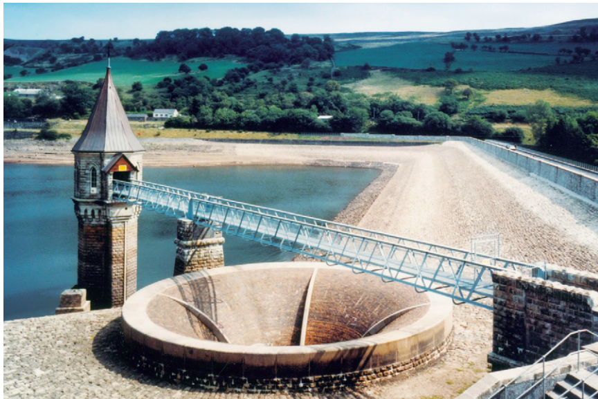
(b) Taf Fechan dam drawoff tower and bellmouth spillway, Wales. (Engineer: Sir Alex Binnie, Son & Deacon)
