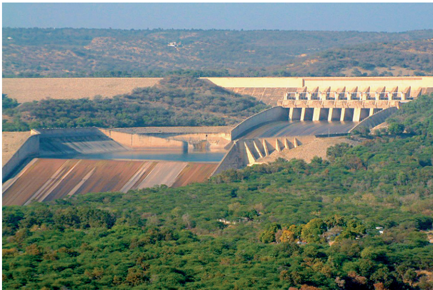
(b) Main spillway of 138 m high earth dam at Mangla, Pakistan—capacity 25 000 m 3 /s. (Engineer: Binnie & Partners) (Courtesy of O J Berthelsen)
