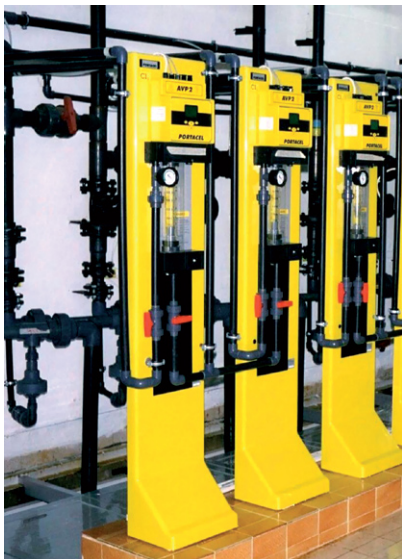
(c) Floor mounted chlorinators. (Manufacturer: Portacel, UK)
