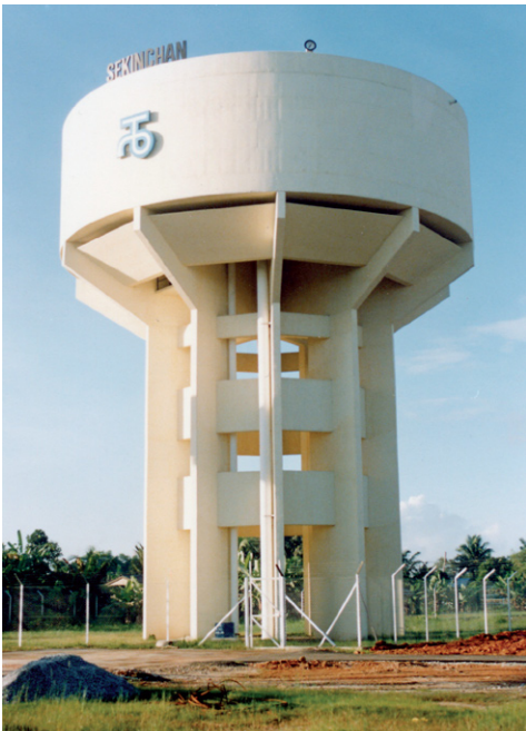
(c) 2270 m 3 reinforced concrete water tower, Malaysia. (Engineer: Binnie & Partners in association with SMHB)
