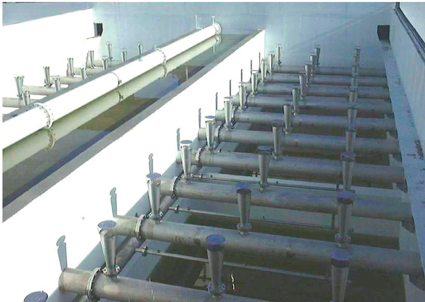
(b) Interior view of a CoCo-DAFF (counter-current dissolved air flotation filtration) clarifier unit.
