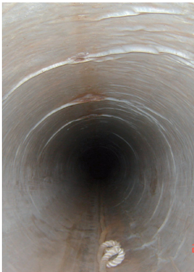
(c) Cure-in-place lining in 600 mm diameter steel pipe. CCTV survey identified defect. (Black & Veatch)
