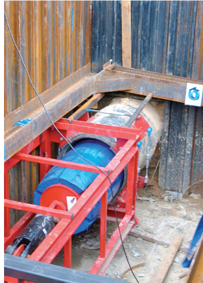
(b) Exit pit—757 mm OD PE still in tension and in its 'swaged' reduced diameter (Black & Veatch)
