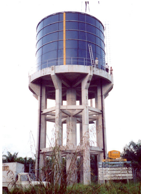
(d) 700 m 3 welded steel water tank on reinforced concrete tower, Malaysia. (Engineer: Binnie & Partners in association with SMHB)
