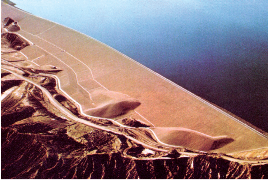
(a) Jari 42 m high earth dam, Mangla, Pakistan. (Engineer: Binnie & Partners)
