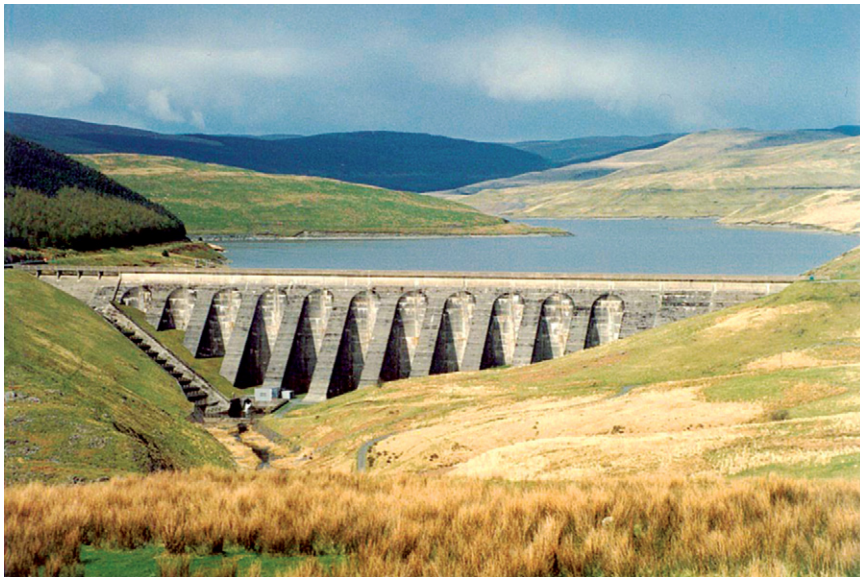
(c) Nant-y-Moch 53 m high buttress dam, Wales. (Courtesy of John Sawyer)
