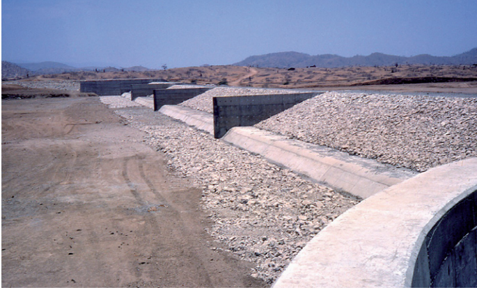
(a) 14 000 m 3 /s capacity fuse plug emergency spillway at Poechos Dam, Peru.
