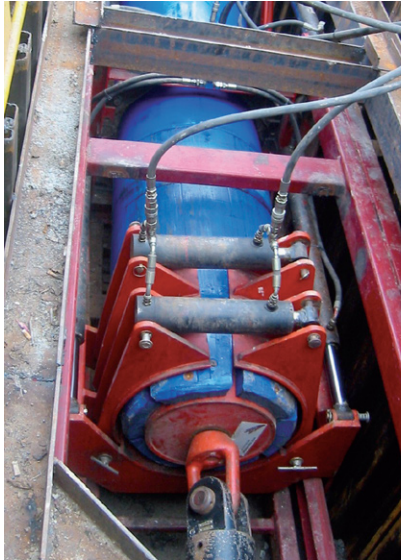
(a) 757 mm OD PE 'swagelining' entering 800 mm diameter host pipe. (Black & Veatch)
