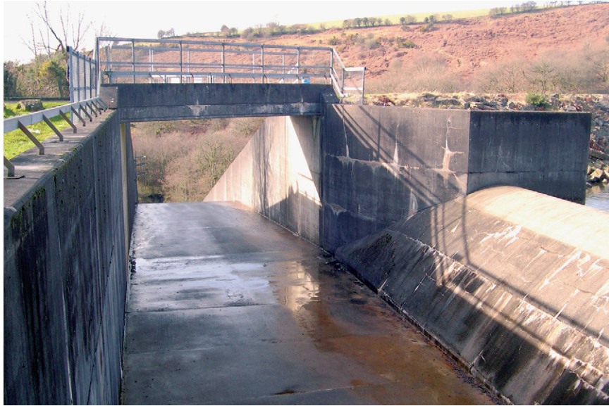
(a) Lower Lliw dam side spillway, Wales. (Courtesy of Welsh Water).
