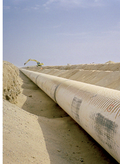
(b) 1524 mm diameter steel pipeline awaiting backfilling in Middle East. (Binnie Black & Veatch)
