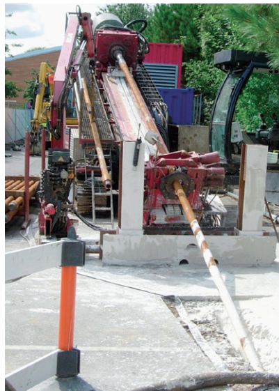
(d) Directional drilling for a 350 mm OD pumping main. (Black & Veatch)
