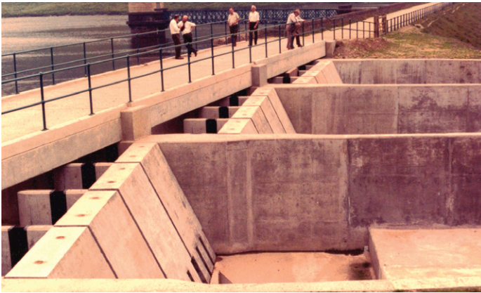
(b) Concrete tipping gates at dam in UK. (Courtesy of John Ackers)
