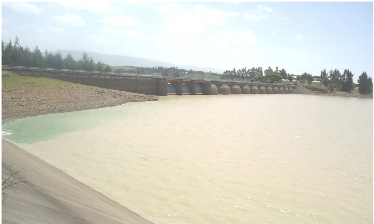
Figure 2.4: Photos of Legedadi Reservoir
