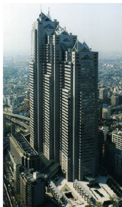
Shinsuku Park Tower (1993) installed with V-shaped HMDs
