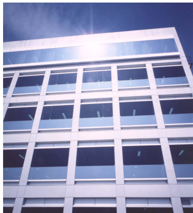
Base Isolated Research Building
