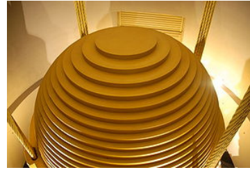
Tuned mass damper atop the of Taipei 101 .
