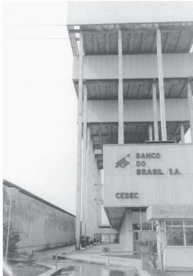
Fig. 12-7 Bank of Brazil building, Porto Alegre, Brazil. Each floor extends out over the floor below it. (Photograph courtesy of J. G. MacGregor.)
