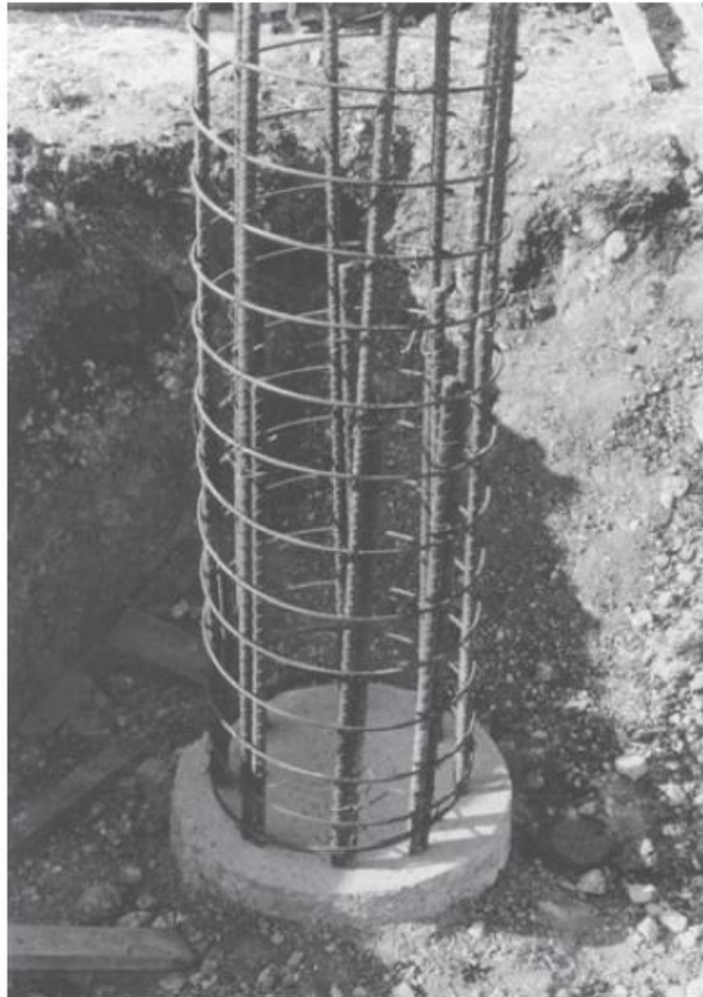
Fig. 11-3 Spiral column. (Photograph courtesy of J. G. MacGregor.)
