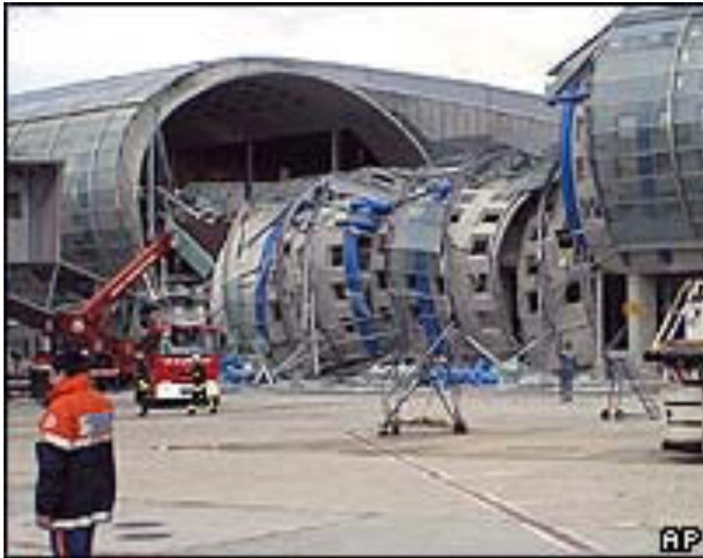
Charles De Gaulle International Airport, Terminal 2E May 23, 2004, 05:00 GMT
