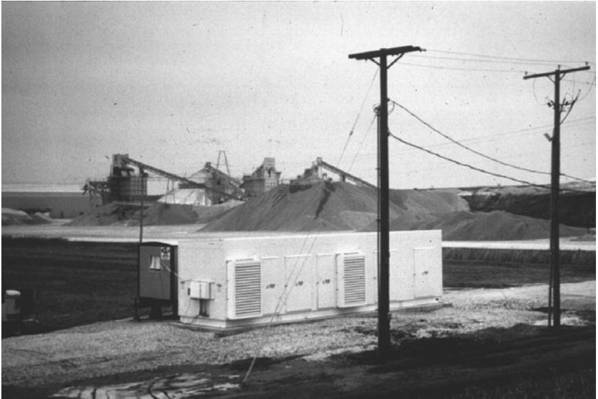
Figure 4.26 DSTATCOM installation. (Courtesy of EPRI.)
