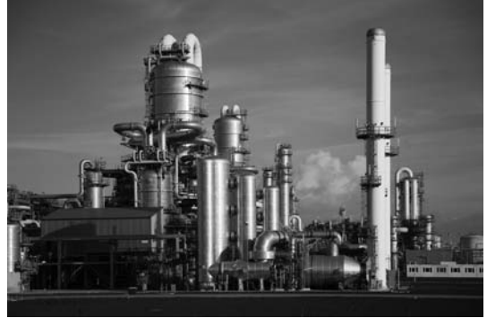
Refinery in Europoort, Rotterdam, Holland iStockphoto
