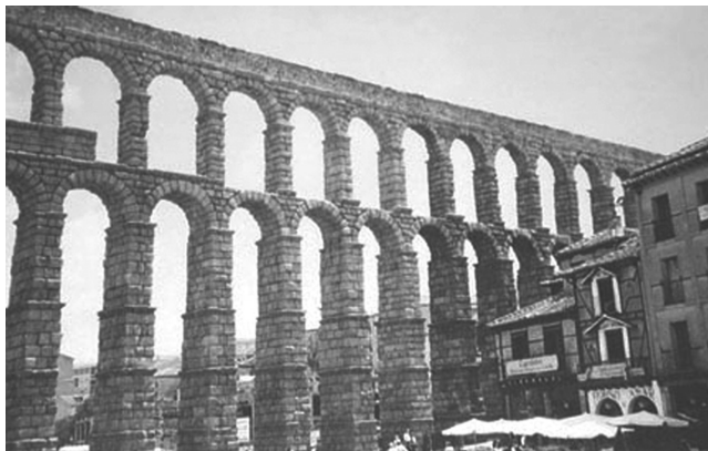
FIGURE 2.5 Roman aqueduct in Segovia, Spain, from the first century AD. (Copyright © 1998 by Stephen L. Sass; reprinted from Sass, S.L., The Substance of Civilization , Arcade, New York.)
