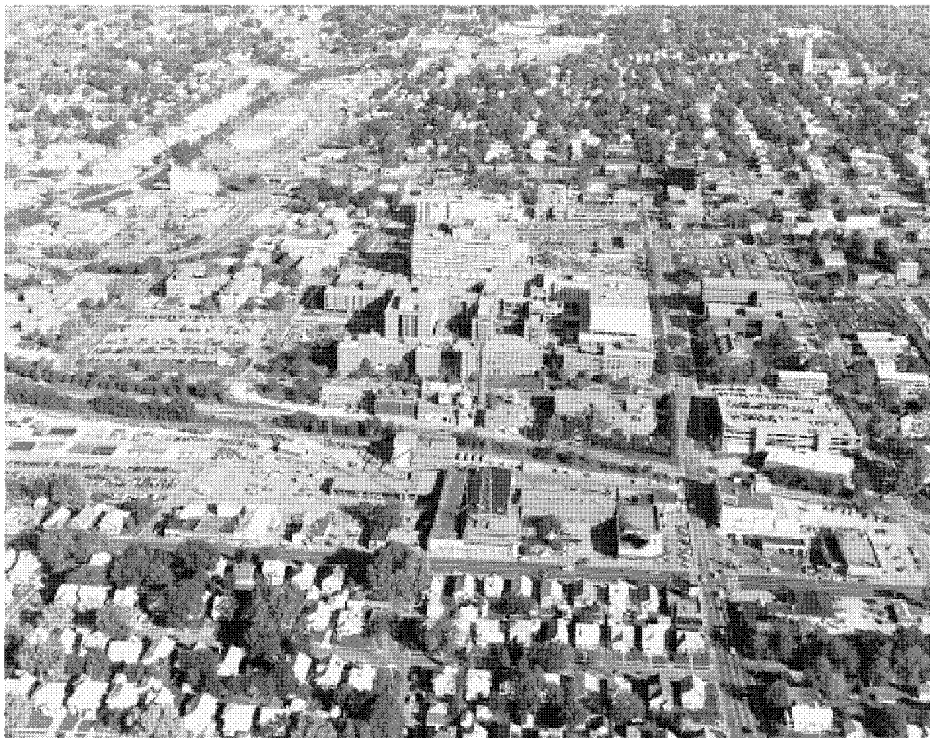
EXPOSURE B URBAN AREA WITH NUMEROUS CLOSELY SPACED OBSTRUCTIONS HAVING SIZE OF SINGLE FAMILY DWELLINGS OR LARGER. FOR ALL STRUCTURES SHOWN, TERRAIN REPRESENTATIVE OF SURFACE ROUGHNESS CATEGORY B EXTENDS MORE THAN TWENTY TIMES THE HEIGHT OF THE STRUCTURE OR 2600 FT (792 M), WHICHEVER IS GREATER, IN THE UPWIND DIRECTION.
