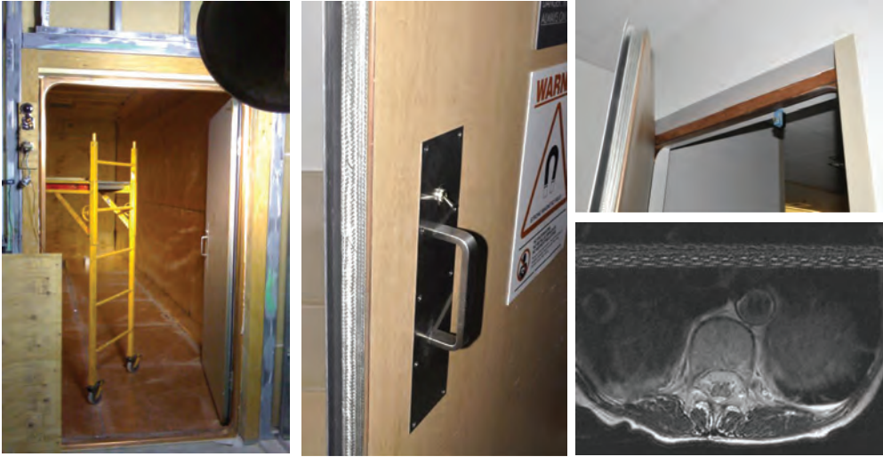
■ FIGURE 13-44 The MR scanner room requires protection from extraneous radiofrequency signals. This is achieved with the installation of a “Faraday cage” comprised of copper sheet that lines the inner walls of the room ( left ), copper mesh covering the operator viewing window (not shown), and a copper lined door and doorjamb with an inflatable bladder conductor (note switch above the door handle) to seal the door ( middle and upper right ). A leak in the Faraday cage will result in RF artifacts that will occur at specific frequencies as streaks across the image, perpendicular to the FEG direction. ( Lower right . FEG is vertical, PEG is horizontal.)
