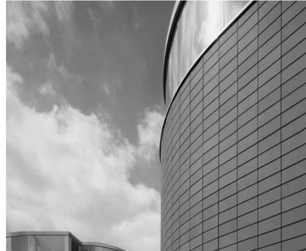
2.4 Argeton terracotta at Churchill Centre Rotterdam (architects: Brookes Stacey Randall). Photo: Christian Richters and Nik Randall.
