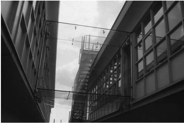
7.38 Laminated toughened glass as used at the glass bridge in Rotterdam by engineer Robert Nijse.
