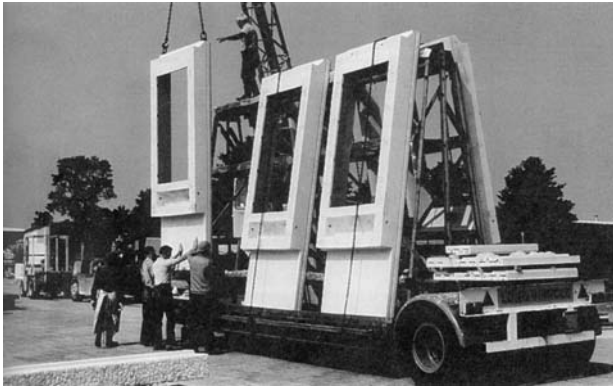
1.8 Wall panels being loaded onto A-frame trailer.
