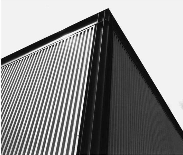
5.30 Corner detail with exposed steel frame.
