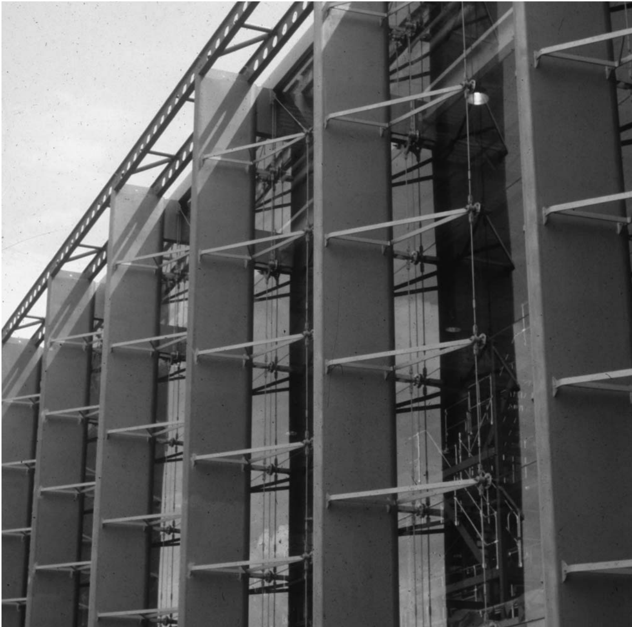
7.28b Suspended glazing at Financial Times Building, London (architects: Nicholas Grimshaw & Partners).
