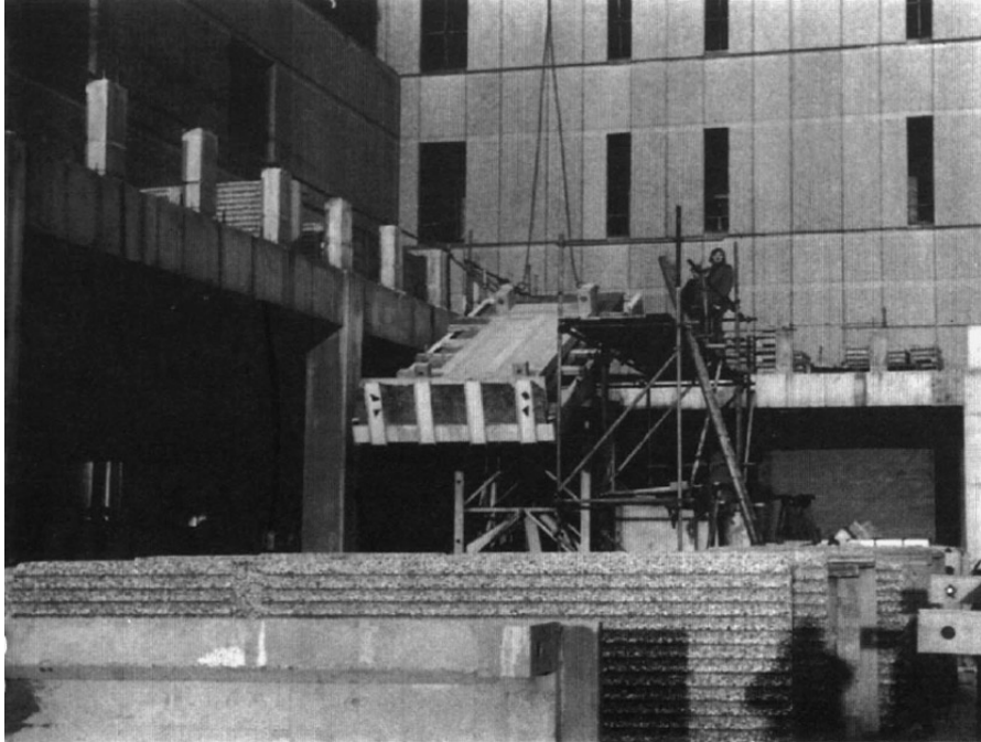
I.15 Tilting platform as used at Liverpool Royal Insurance building.
