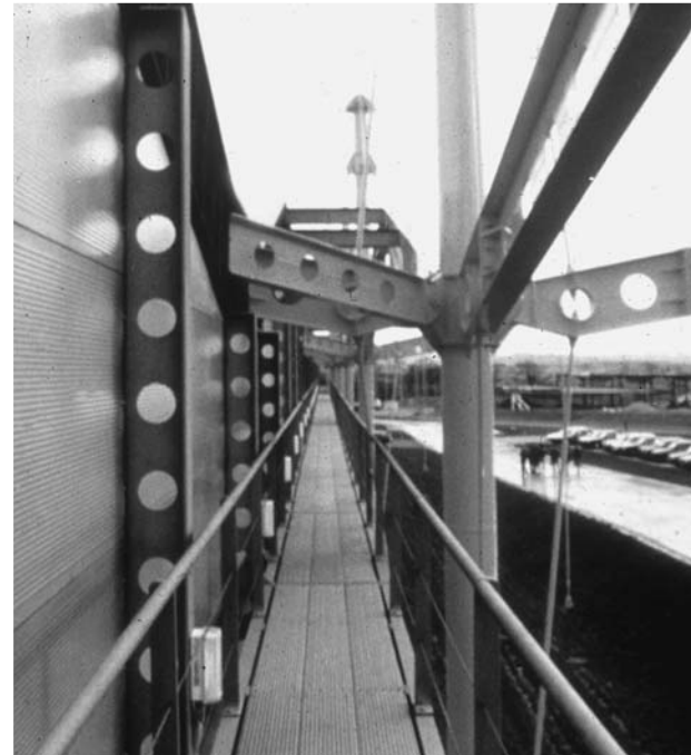
6.11 Panels at Renault Centre.
