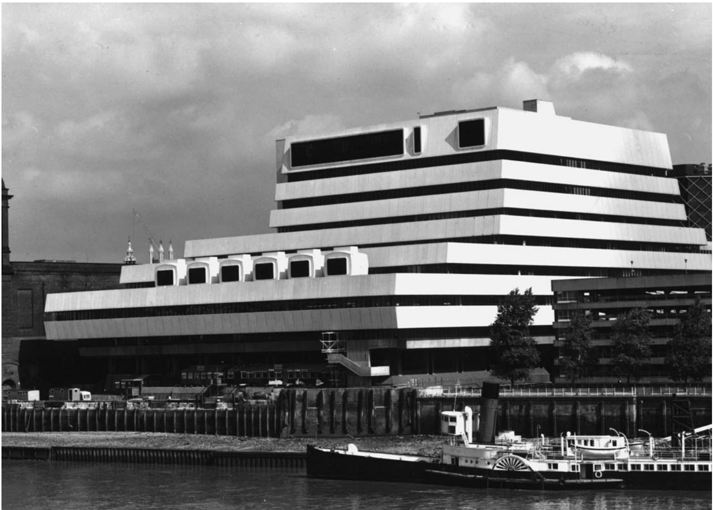
3.7 Mondial House, London, demolished 2006 (architects: Hubbard Ford & Partners).
