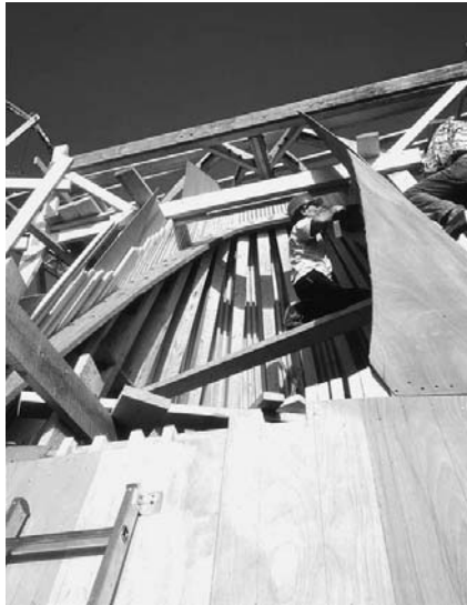
8.30 Timber construction of the Law Courts in Bordeaux.
