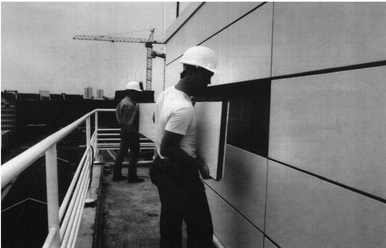
6.37 Interchangeable facade panels.
