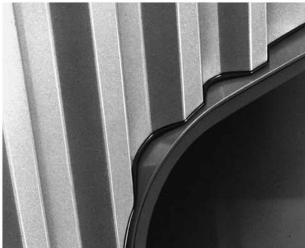
5.31 Neoprene flashing at window opening.
