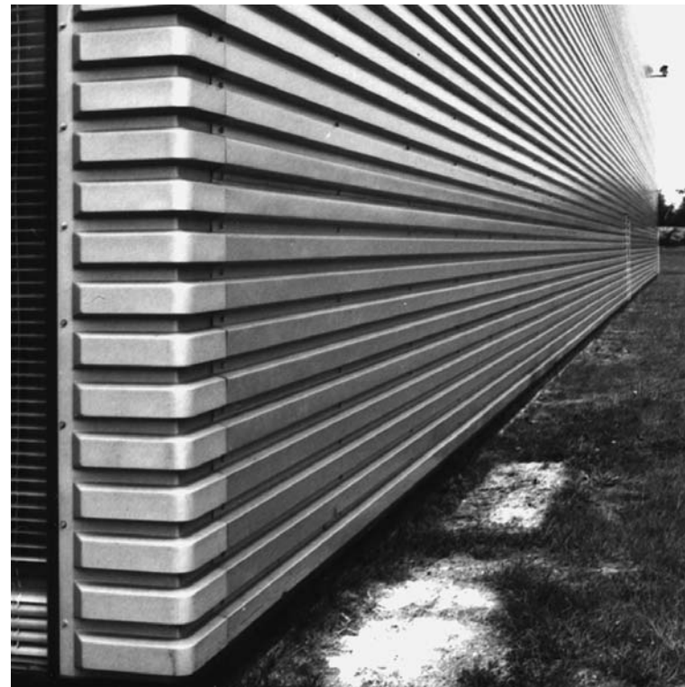
5.14 IBM offices, Greenford (architects: Foster Associates).
