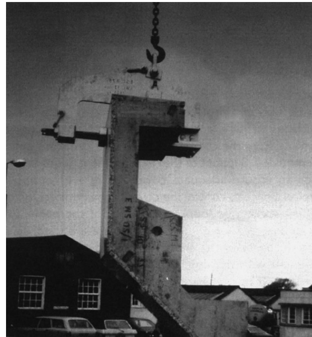
1.14 Special lifting tackle for cranked units.
