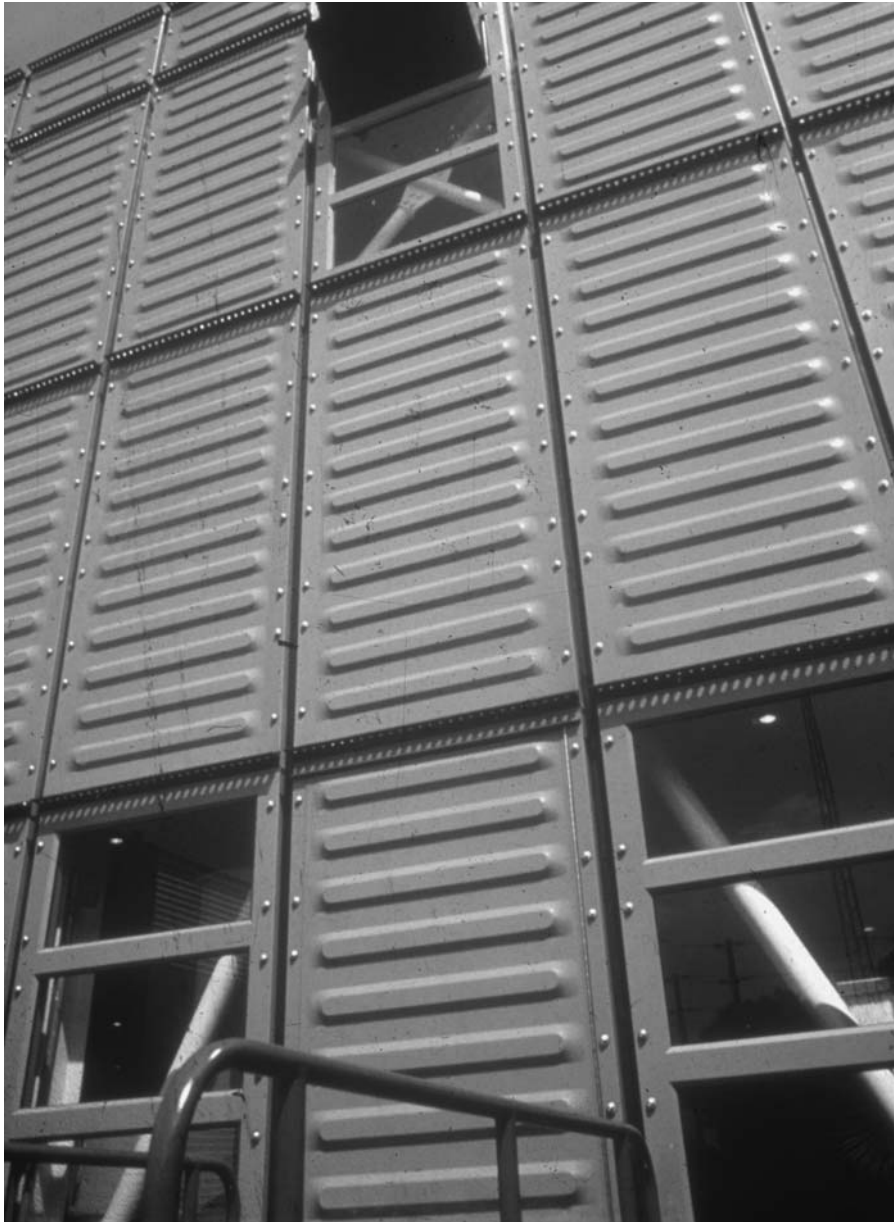
5.9 Stamped aluminium panels 2.4 m × 1.2 m at Herman Miller extension, Bath.
