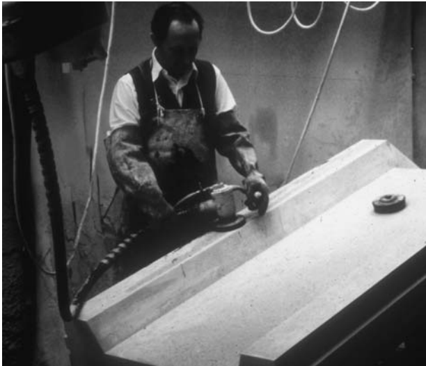
1.6 Cladding unit in course of finishing by hand.
