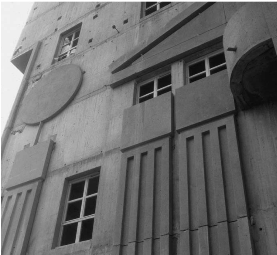
1.1 Construction of precast and in situ concrete at the Les Espaces d'Abraxas, a monumental housing scheme near Paris (architect: Ricardo Bofill).
