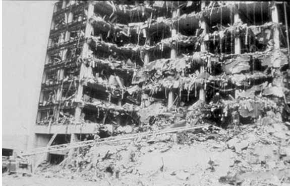
Figure 2.4 Oklahoma City Federal Building, following explosion. (Source: City of Oklahoma City, Public Information and Marketing. Used with permission.)
