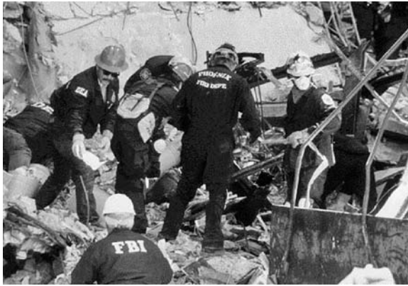
Figure 10.2 Urban Search and Rescue Team from Phoenix, working at the Alfred P. Murrah Federal Building explosion in Oklahoma City. (Source: FEMA.)
