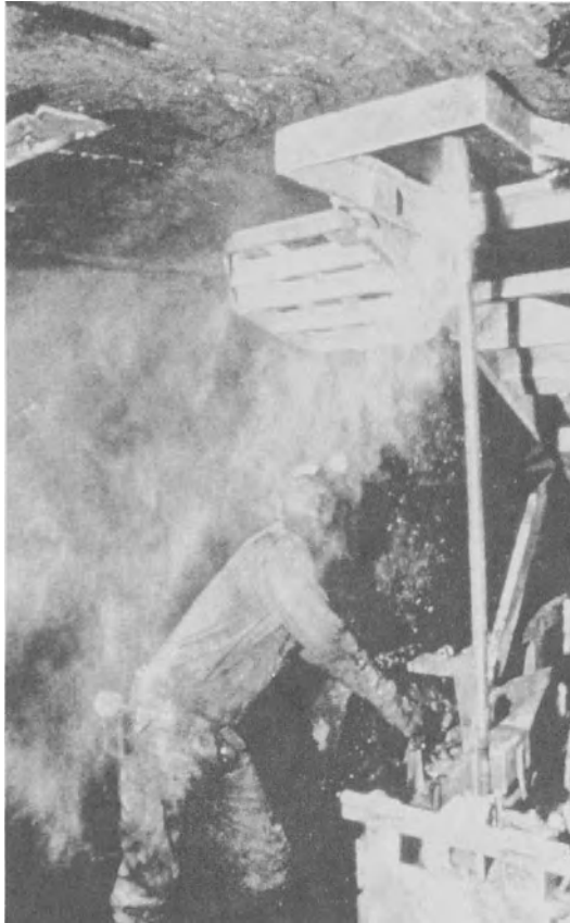
FIGURE 1. - Dust being generated by roof bolting in underground coal mine.
