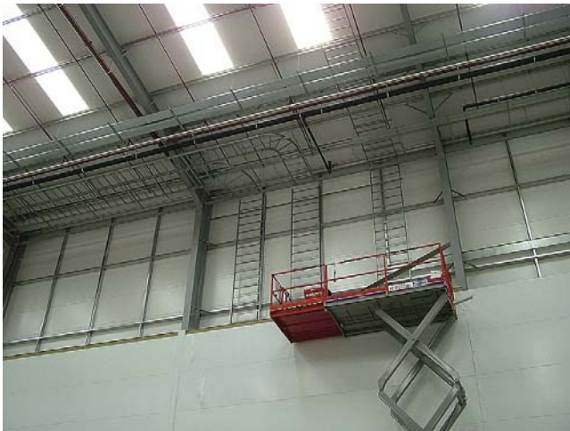
FIGURE 1.4 Another scissors lift suitable for safe working at height. Many industrial and commercial sites require installation work which demands the use of such equipment.
