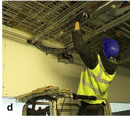
(c) Distribution board in position with modular wiring looms fitted into the distribution cupboard, carried on a cable basket route. (d) Installing modular cable units on cable basket behind a suspended ceiling.
