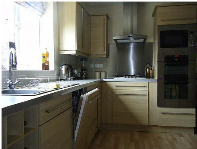
FIGURE 4.1 Kitchens often require a separate ring circuit to cater for the expected loads. Dish washers, clothes washers and dryers are often encountered in addition to the equipment shown here.
