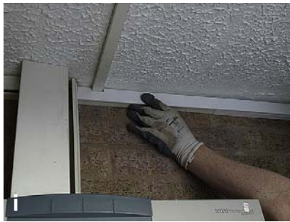
FIGURE 10.7 cont'd. Installing plastic mini-trunking.
