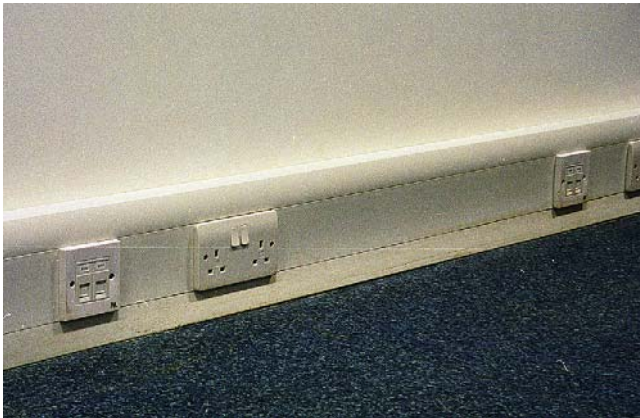
FIGURE 10.4 Multi-compartment skirting trunking allows the segregation of different types of circuit. In this example 13 A ring main socket outlets and telecommunications circuits are provided (W.T. Parker Ltd).
