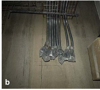
(a) The pre-formed wiring units with plugs attached are conveniently stored and carried on this wheeled trolley preparatory to installation. All units are numbered to ensure correct installation. (b) Modular wiring installed ready for the distribution board to be secured and plugged in.
