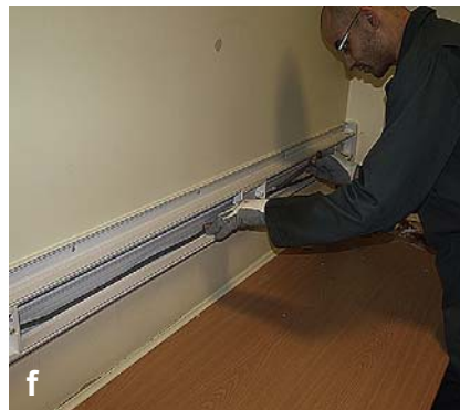
(e) After the cable has been placed into the centre compartment, the socket boxes are clipped in position. (f) The cable feeding the socket outlets is installed behind the outlet boxes.
