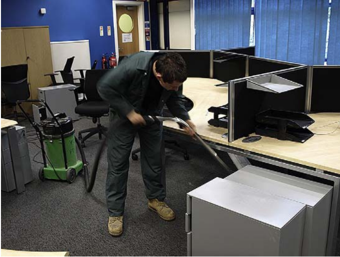
FIGURE 8.16 The installation is completed, the competent electrician makes sure the site is left tidy. A vacuum cleaner is an essential part of the electrician's equipment (M.W. Cripwell Ltd).
