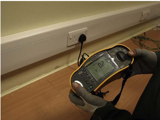
FIGURE 16.7 The same instrument in use for a continuity test.
