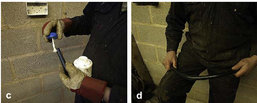
(c) Jointing is carried out by the use of solvent adhesives, and care must be taken in their application to avoid blocking small-sized conduits. (d) Bending can be by hand and a bending spring is used to retain the shape of the bore. In cold conditions, the conduit should be warmed before being bent through an angle slightly greater than that required. It is then returned to the right angle generally needed for bends.
