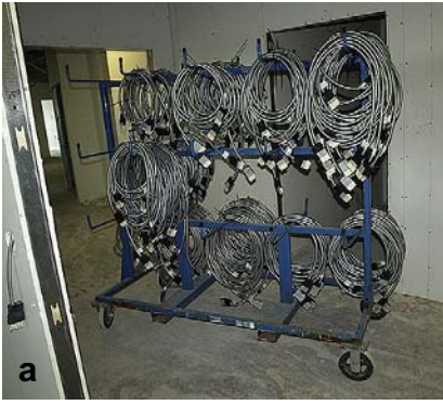
(a) The pre-formed wiring units with plugs attached are conveniently stored and carried on this wheeled trolley preparatory to installation. All units are numbered to ensure correct installation. (b) Modular wiring installed ready for the distribution board to be secured and plugged in.
