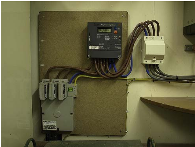
FIGURE 5.2 Typical three-phase commercial intake arrangement.
