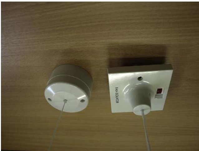
FIGURE 7.1 Cord-operated switches for use in bathrooms can be obtained in a variety of designs, with or without a neon pilot light and, if needed, with engraved labelling as with the fan isolator shown.
