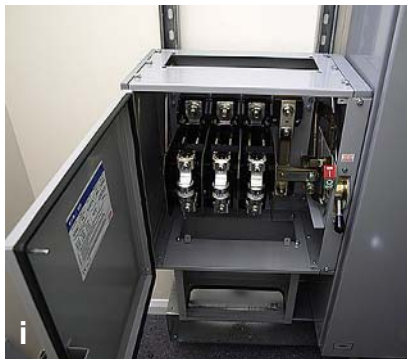
FIGURE 12.1 cont'd. Installation of main incoming switch.
