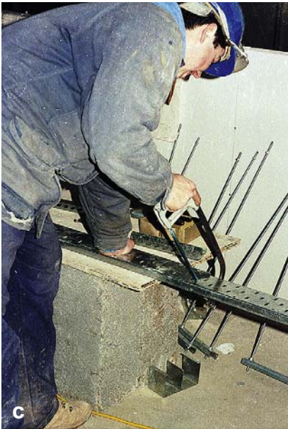
(c) The cable tray is cut using a hacksaw. (d) Using a file, burrs are removed to prevent damage to cables.
