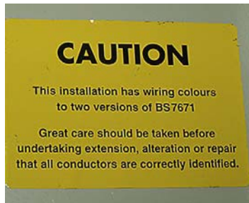
FIGURE 8.8 In any installation where alterations to the wiring give rise to a mixture of colours from the old and current standards, it is a requirement to display a warning notice worded as shown. This should be placed 'at or near the appropriate distribution board' (IEE Regulation 514.14.1).
