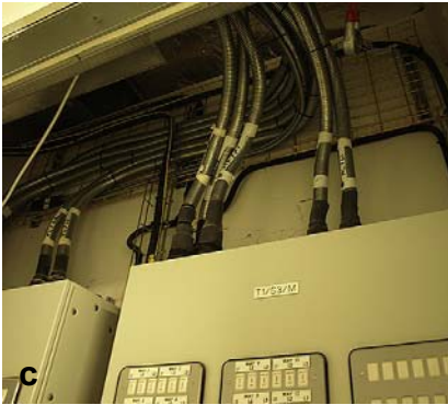
(c) Distribution board in position with modular wiring looms fitted into the distribution cupboard, carried on a cable basket route. (d) Installing modular cable units on cable basket behind a suspended ceiling.
