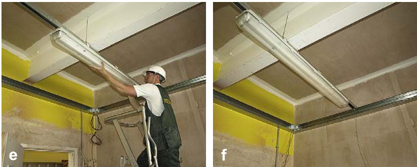
FIGURE 15.3 Installing a fluorescent lighting fitting.
