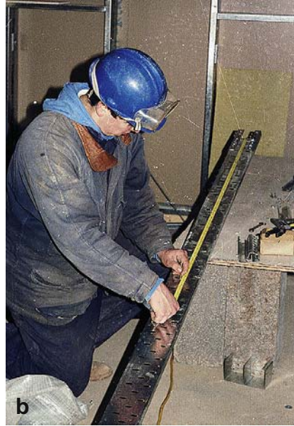
(a) Supports appropriate for the installation are first fitted. Here ceiling supports to carry cable tray and trunking above a suspended ceiling can be seen. (b) The length of tray required is measured and marked off, ready for cutting.
