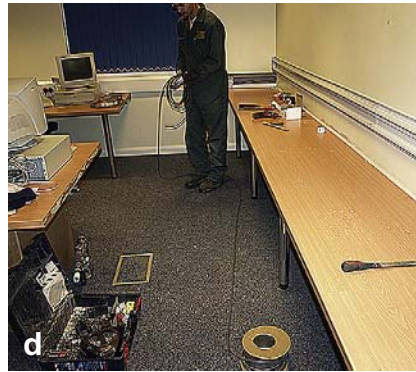
(c) Having checked the length required, cut the trunking using a fine-tooth hacksaw, the complete section is screwed in position on the wall. In this case the battery powered electric screwdriver is fitted with a light to aid the work. (d) The flat twin and CPC cable is prepared for use by running it out to avoid twists and kinks.
