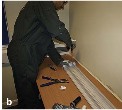
(a) Three-compartment dado trunking ready for fitting. The compartments and one of the lid sections can be clearly seen. (b) The end caps are screwed into position.
