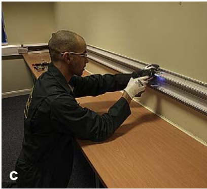
(c) Having checked the length required, cut the trunking using a fine-tooth hacksaw, the complete section is screwed in position on the wall. In this case the battery powered electric screwdriver is fitted with a light to aid the work. (d) The flat twin and CPC cable is prepared for use by running it out to avoid twists and kinks.
