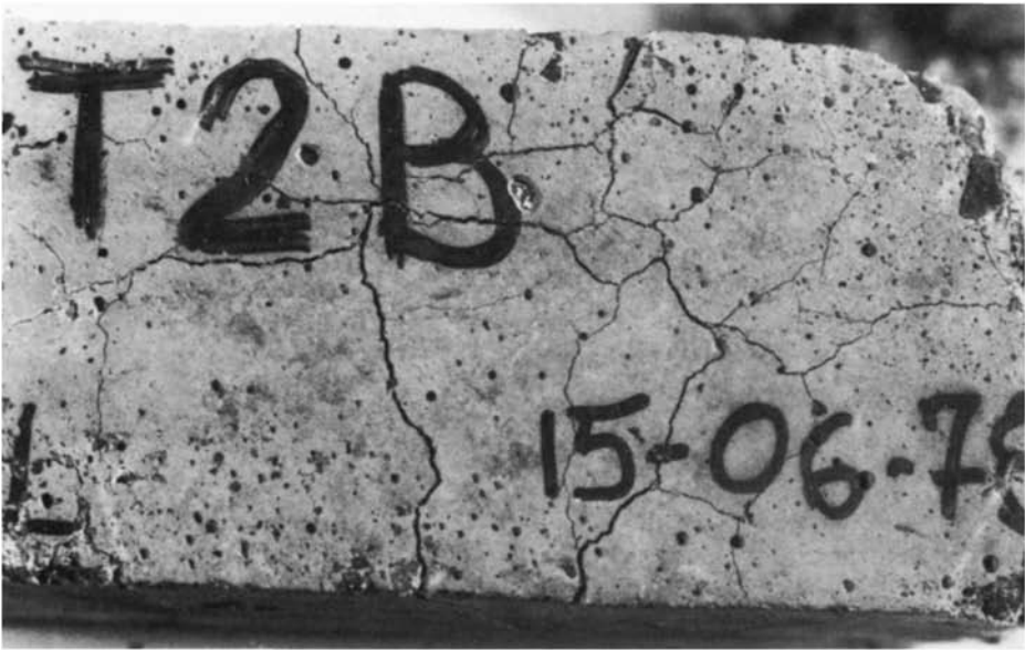
Figure 2.5 Typical map cracking on a concrete specimen caused by repeated cycles of freezing and thawing in air (after Pigeon and Lachance, 1981).
