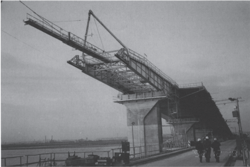
Fig. 4.16 The 605 m-long north approach built as an incrementally launched structure. The final weight of the approach was 26000 tonnes. Courtesy of Paul Acker.
