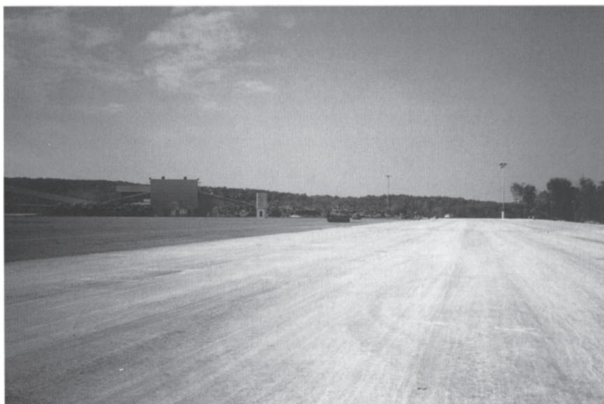
Fig. 18.15 General aspect of the finished surface, the white colour results from the use of a curing membrane.
