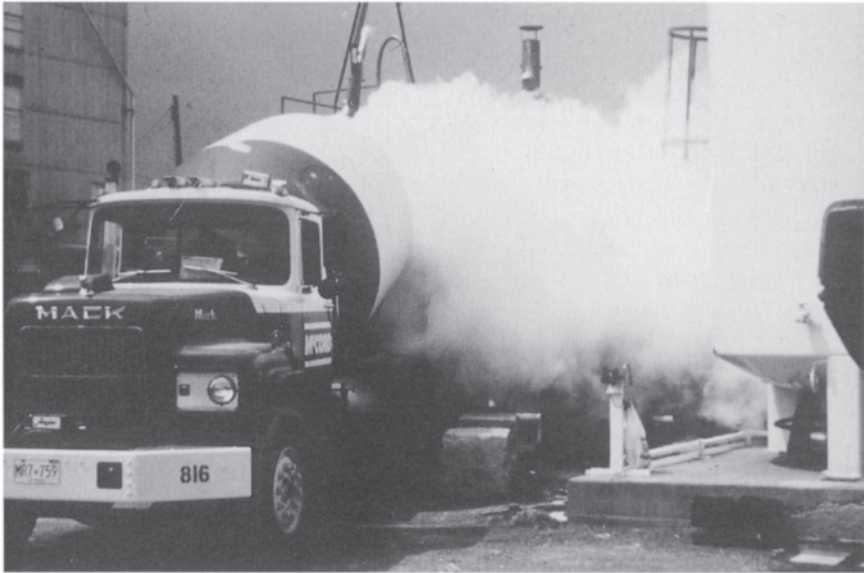
Fig. 9.2 Liquid nitrogen cooling of the high-performance concrete used to build Scotia Plaza in Toronto.
