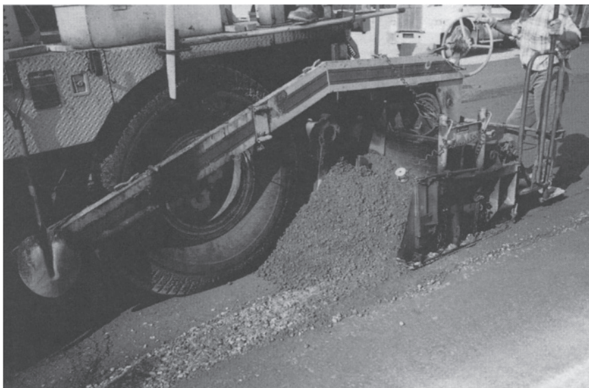
Fig. 18.11 Placing the roller-compacted high-performance concrete with an asphalt paver.
