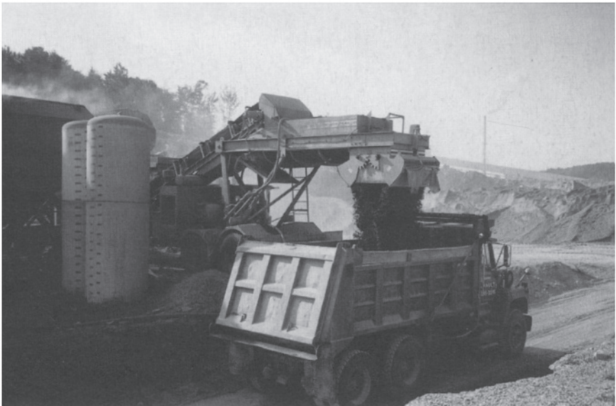
Fig. 18.10 Preparation of the roller-compacted high-performance concrete mix in an asphalt plant.
