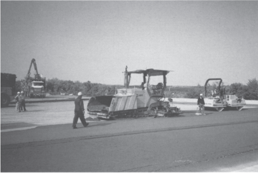
Fig. 18.13 Compacting the concrete surface and checking the unit mass with a nucleodensimeter.
