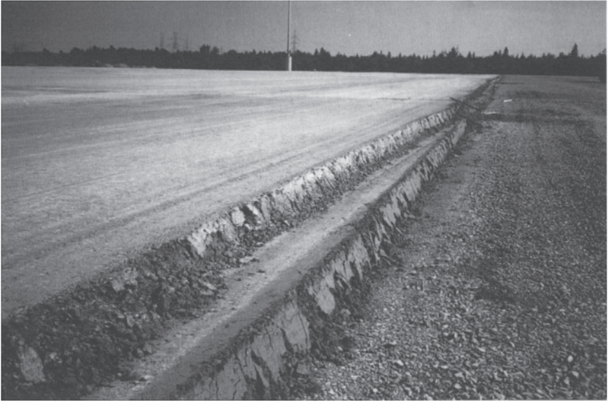
Fig. 18.9 Aspect of two 150 mm layers after their compaction. Note that the longitudinal joints of the two layers are slightly apart from each other.
