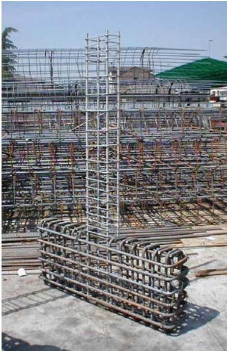
Fig. 11. Steel reinforcement of the column prototype.
