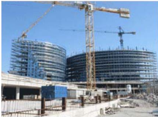
Fig. 2. WTC in San Marino construction site.
