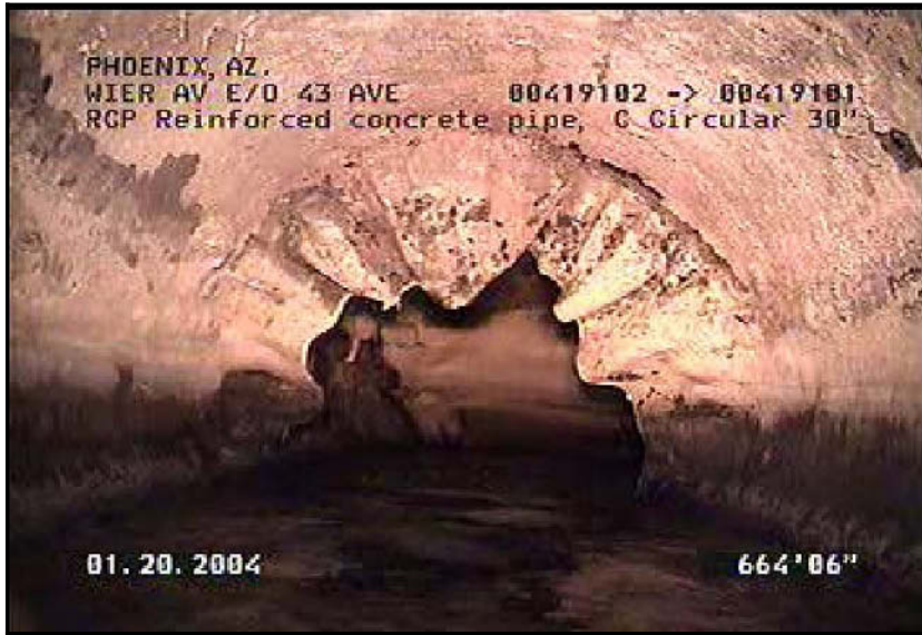
Figure 2. Detached liner
