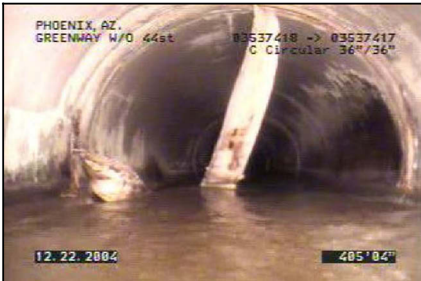
Figure 3. Detached weldstrip
