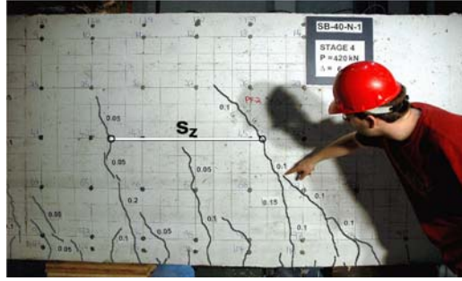
Fig. 5. Crack pattern in member without stirrups. s_z is spacing at mid-depth.
