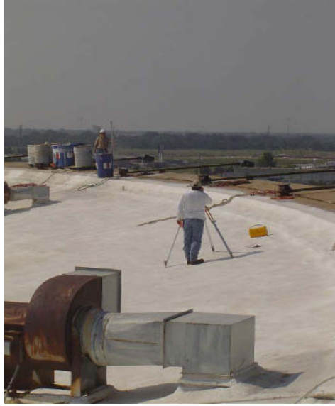
Figure 3. Surveying to determine roof sag.
