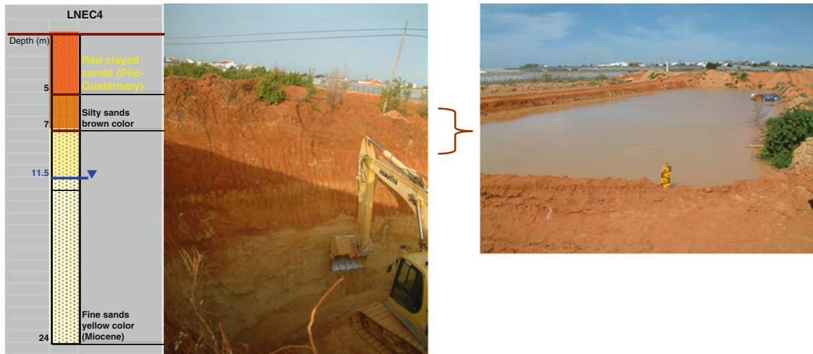
Fig. 9 Vertical profile of lithological materials in Areal Gordo (at right) and LNEC4 well lithological column and infiltration basin in the first layer (at left)
