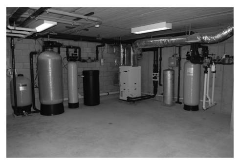
Potable water system on the left comes from the well. Ground source heat pump is in the Center. Nonpotable water system on the right comes from the cistern. *Photograph Taken by Dr. Luke Gascho. Reproduced by Permission.*
