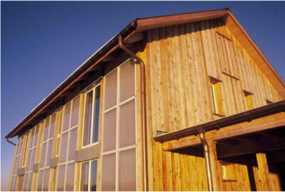
Passive Solar Heating in Built Environment. Figure 18 Swiss TWD house at Hundwiler Höhe (architect and photo source: P. Dransfeld, www.dransfeld.ch )
