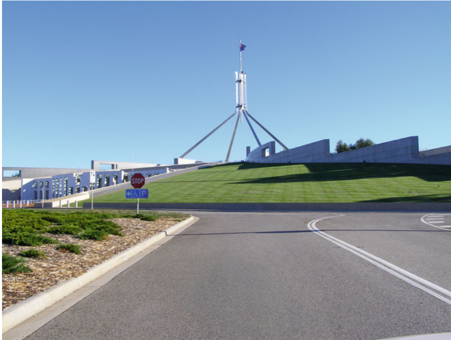
Green Roof Infrastructures in Urban Areas. Figure 2
