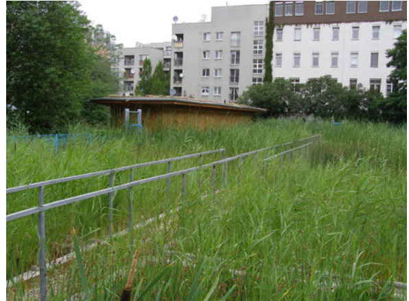
Green Roofs, Ecological Functions. Figure 8 Block 6. Plant sewer system in Berlin with rainwater cleaning facility in the back yard of a residential area of the City Center of Berlin, Details on this project can be seen at: http://www.stadtentwicklung.berlin.de/bauen/oekologisches_bauen/download/modellvorhaben/flyer_block6_engl.pdf
