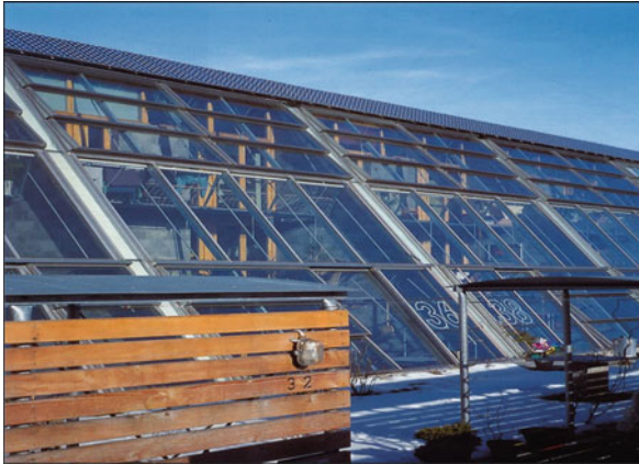
Passive Solar Heating in Built Environment. Figure 26 Attached sunspaces as part of the concept of low energy row housing in Bern (Architects, AARPLAN; Bern, CH)
