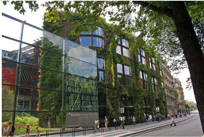
Facades and Enclosures, Building for Sustainability. Figure 12 Green walls at Musée Branly reduce heat gain in summer
