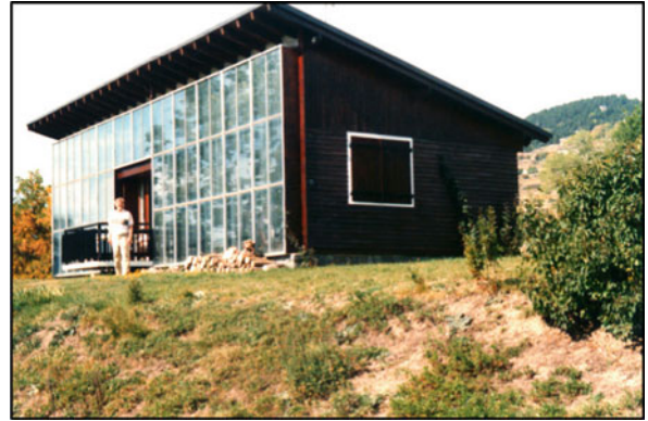
Passive Solar Heating in Built Environment. Figure 15 The prototype Michel-Trombe wall house in Odeillo, FR (source: Robert.hastings@aeu.ch)
