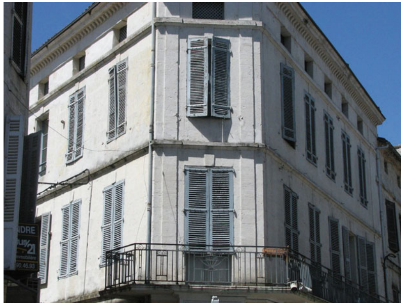
Daylight, Indoor Illumination, and Human Behavior. Figure 4 Solar protection using moveable shutters (Dordogne region, France)
