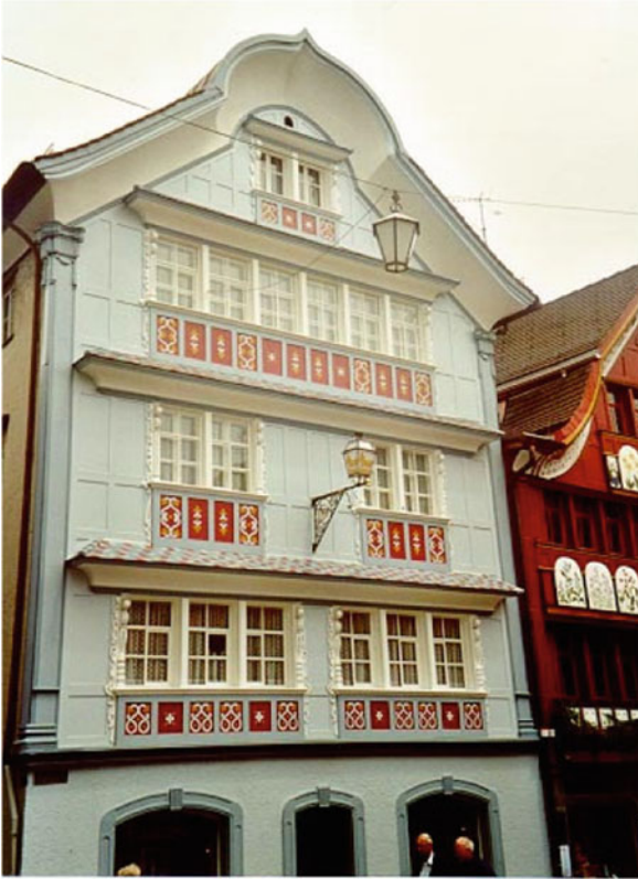
Passive Solar Heating in Built Environment. Figure 4 An Appenzell house with large window area protected by multiple roof projections (photo: robert.hastings@aeu.ch)
