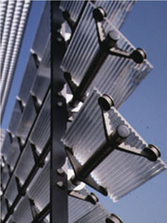
Daylighting Controls, Performance and Global Impacts. Photo 10 Prisms are translucent but prevent visual transmission [14]
