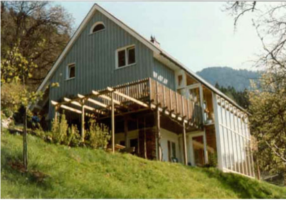
Passive Solar Heating in Built Environment. Figure 9 An Austrian passive solar house with solar air radiant heating and a sunspace in Nüziders, Vorarlberg (architect and photo source: Sture Larsen, www.solarsen.com )
