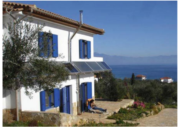
Passive Solar Heating in Built Environment. Figure 23 A solar air heater for a vacation home on a Greek island (photo and system information: www.grammer-solar-bau.de )
