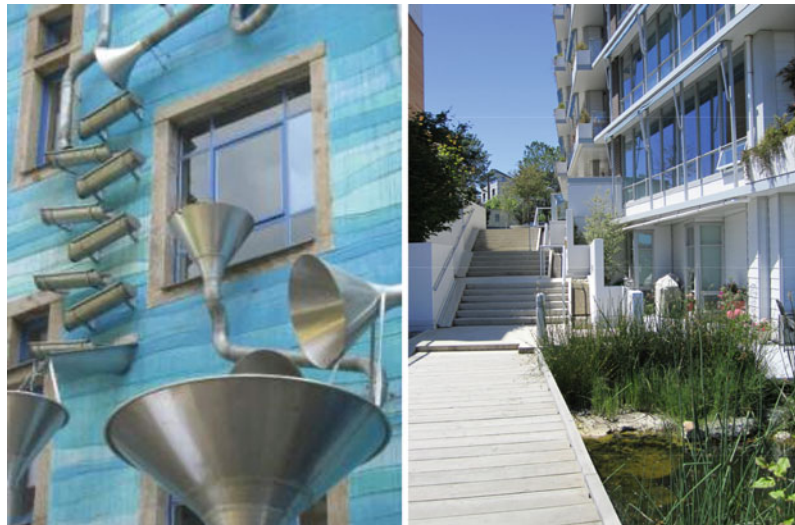
Facades and Enclosures, Building for Sustainability. Figure 25 On the left , water sculpture by Herbert Dreisetl playfully manages storm water, enticing visitors to return in the rain to watch. On the right , rainwater capture provides acoustic and visual richness in the Dockside Green development by Joe Van Bellingham
