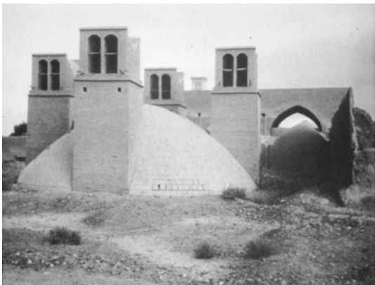
Natural Ventilation in Built Environment. Figure 2 Wind towers in Yazd, Iran to ventilate houses, are also constructed to cool underground cisterns (water reservoir) [3]
