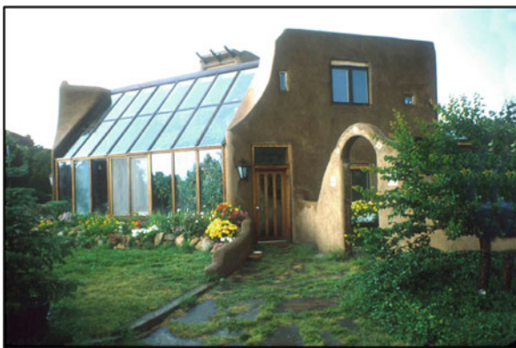
Passive Solar Heating in Built Environment. Figure 6 The Balcomb house in New Mexico (photo source: robert.hastings@aeu.ch)
