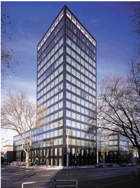
Daylighting Controls, Performance and Global Impacts. Photo 19 Daylight façade with RetroLux (Fig. 15), municipal works, Bochum, Germany. Architects: Gattermann + Schossig, Cologne
