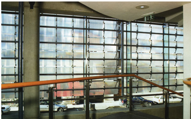
Daylighting Controls, Performance and Global Impacts. Photo 11 Prisms are translucent but prevent visual transmission [14]
