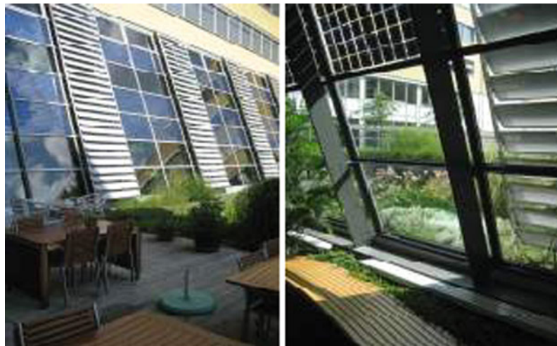
Facades and Enclosures, Building for Sustainability. Figure 22 Interior and exterior views of the south facade at Fraunhofer Institute in Freiburg illustrate the integration of active and passive solar strategies
