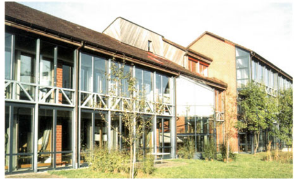
Passive Solar Heating in Built Environment. Figure 10 A Swiss school in Gumpenwiese ZH with sunspaces tied into the ventilation concept [16] (photo: robert.hastings@aeu.ch)
