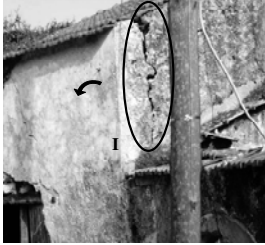
Fig. 7. Vertical crack, 2007
