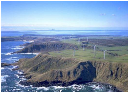
Fig. 2. The Woolnorth wind farm at cliff
