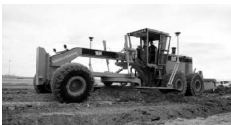
Grader with GNSS antennae mounted on blade
