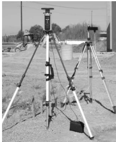
Figure 7.19 • RTK base station showing reference receiver (left) with UHF transmitter (courtesy Thales).
