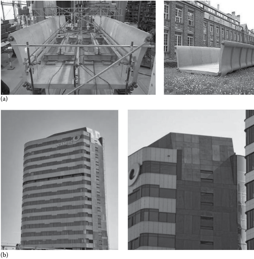
Figure 1.5 Structural and architectural components from TRC: (a) profile for a bridge (Technical University, Dresden, Germany) and (b) curtain walls for facades, office building, Arnhem, NL (Fydro B.V., NL). (a: From Hegger, J. et al. (eds.), in First International Conference in Textile Reinforced Concrete (ICTRC1) , Aachen, Germany, 2006a; b: From Hegger, J. et al., Applications of textile reinforced concrete, Chapter 8, in W. Brameshuber (ed.), Textile Reinforced Concrete: State of the Art Report, RILEM TC 201-TRC , RILEM Publications, Paris, France, 2006b, pp. 237–270.)
