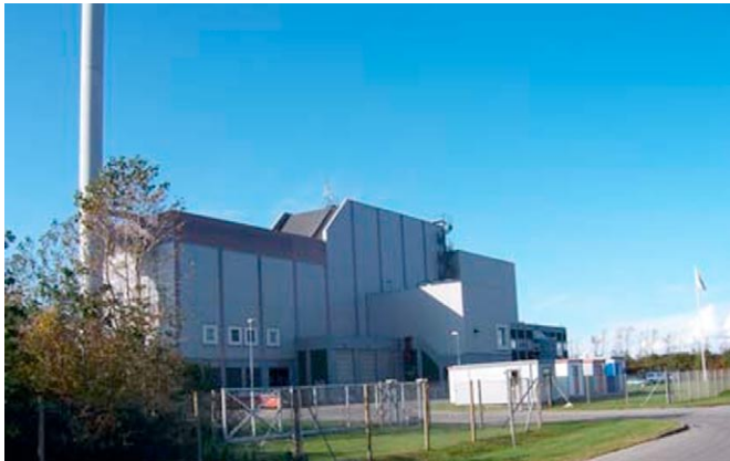
Figure 14.7 Waste incineration plant in Frederikshavn.
