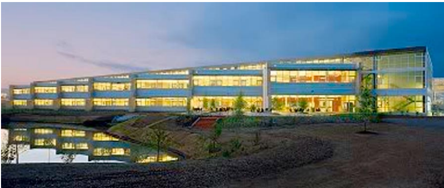
Figure 4.3 Making a statement about green design, the Alberici construction company of Missouri built its new headquarters as one of the highest scoring LEED™ platinum buildings. (LEED™, Leadership in Energy and Environmental Design, is the green building certification program of the U.S. Green Building Council, a nonprofit trade association in the building industry. LEED™ attempts to encompass all environmental impacts of building. LEED™ platinum is the most demanding of four levels of certification.) The architects reused the shell of a 50-year-old manufacturing and office facility, orienting the new facades of the rebuilt structure to the south to capture more winter sun and optimized natural ventilation flows to increase energy efficiency and improve indoor air quality.
