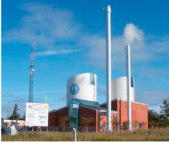
Figure 14.6 Natural-gas-fired cogeneration heat and power plant in Strandby, Denmark.
