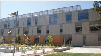
L.A. Valley College's Allied Health & Science Center's rooftop has a solar energy system that generates approximately 10 percent of the building's electricity needs.
