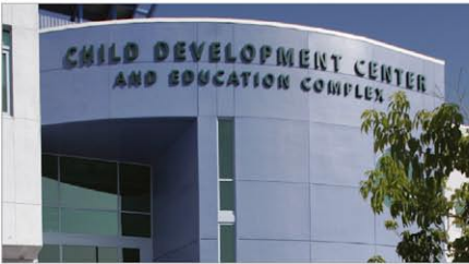
L.A. Southwest College's Child Development Center is LEED™ certified and was honored with a Project Achievement Award.
