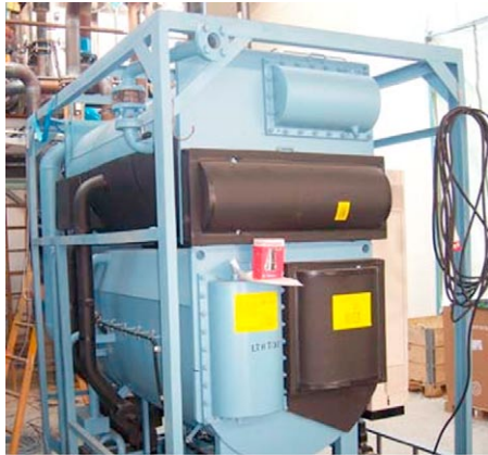
Figure 14.9 Absorption heat pump in Strandby.
