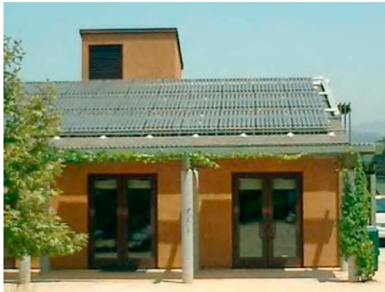
Figure 4.5 This near-zero energy building in Los Angeles, the Audubon Center at Debs Park, has an innovative system of rooftop solar thermal collectors and absorption cooling, which use solar heated water to both heat and cool the well-insulated interior space (also a LEED™ platinum building).
