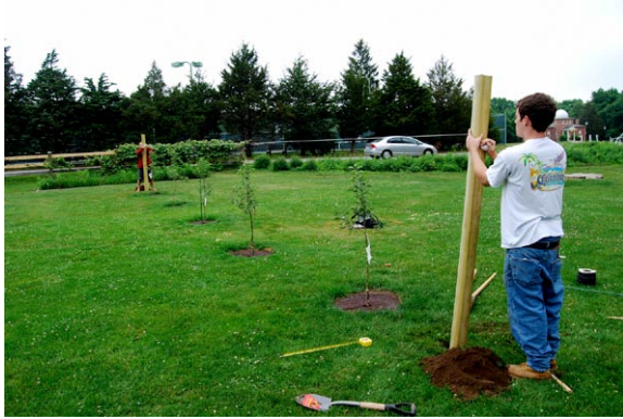
Figure 13.10 In order to strategically yield the most fruit, orchard manager Schuyler Horn takes the lead during the construction of orchard structural scaffolding.
