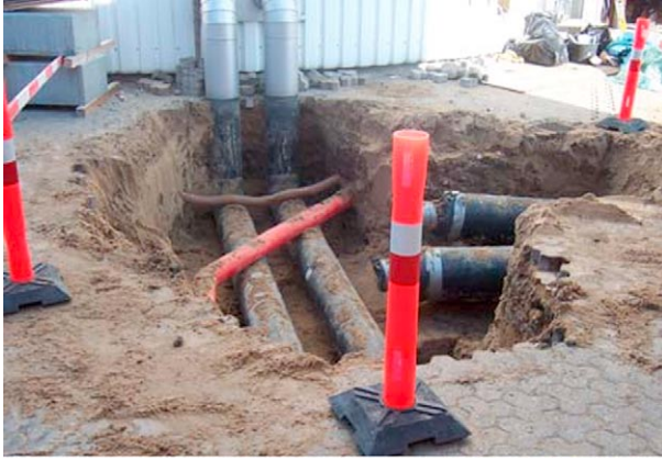
Figure 14.5 Installation of district heating pipes.
