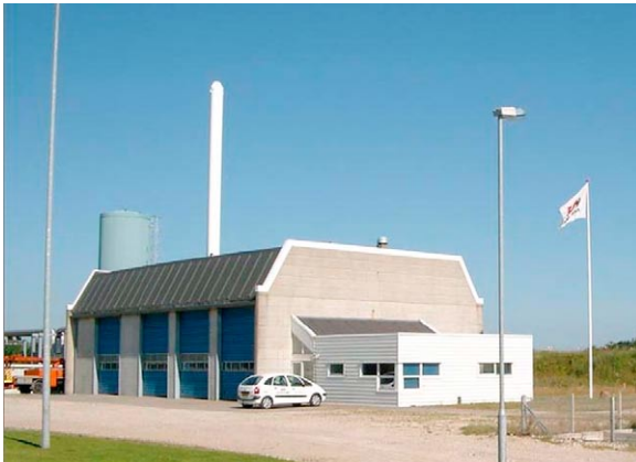
Figure 14.14 The geothermal plant in Thisted, Denmark.
