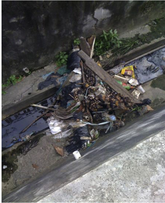
Figure 19 Trash, including plastic bags and plastic water bottles, often clogs drainage systems, contributing to flooding (Balikpapan).
