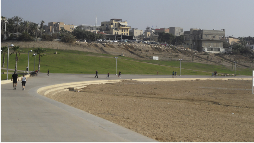
Figure 5 A stretch of beach currently being rehabilitated at Jaffa Slope Park.
