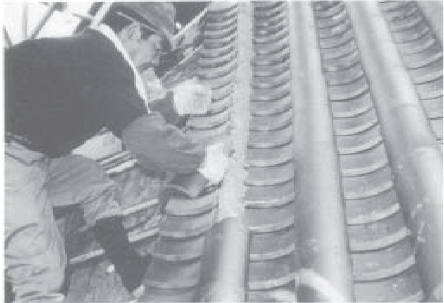
Fig 3.9 Terracotta tiles being laid on temple roof (Enryakuji restoration, 1980)
