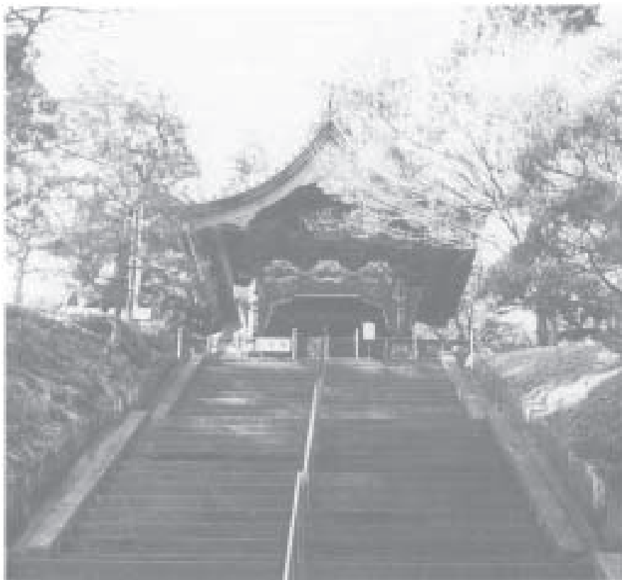
Fig 7.7 Taitokuin mausoleum, Onarimon. View from approach steps. Relocated at Fudoji, Saitama prefecture in 1972
