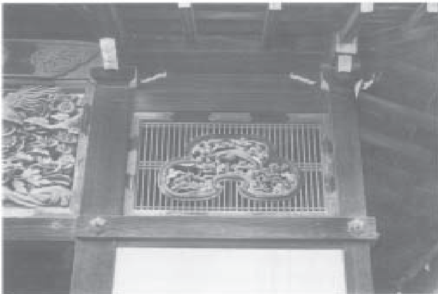
Fig 6.14 Nijo Castle. Palace of the Second Compound. Entrance and side transom with kushigata (comb-pattern) frieze
