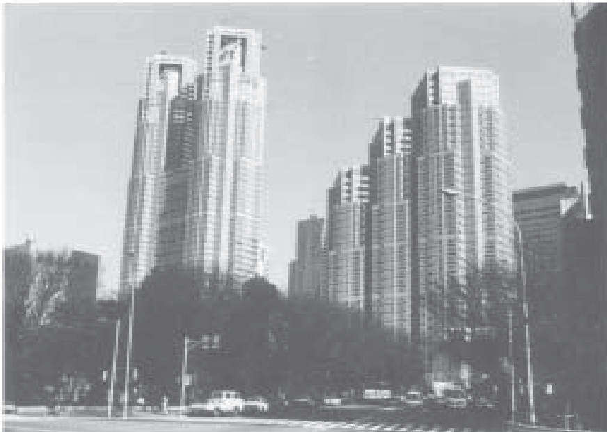
Fig 10.11 New Tokyo Metropolitan Government Headquarters. View of Tower I (left) and Tower II (right) from west
