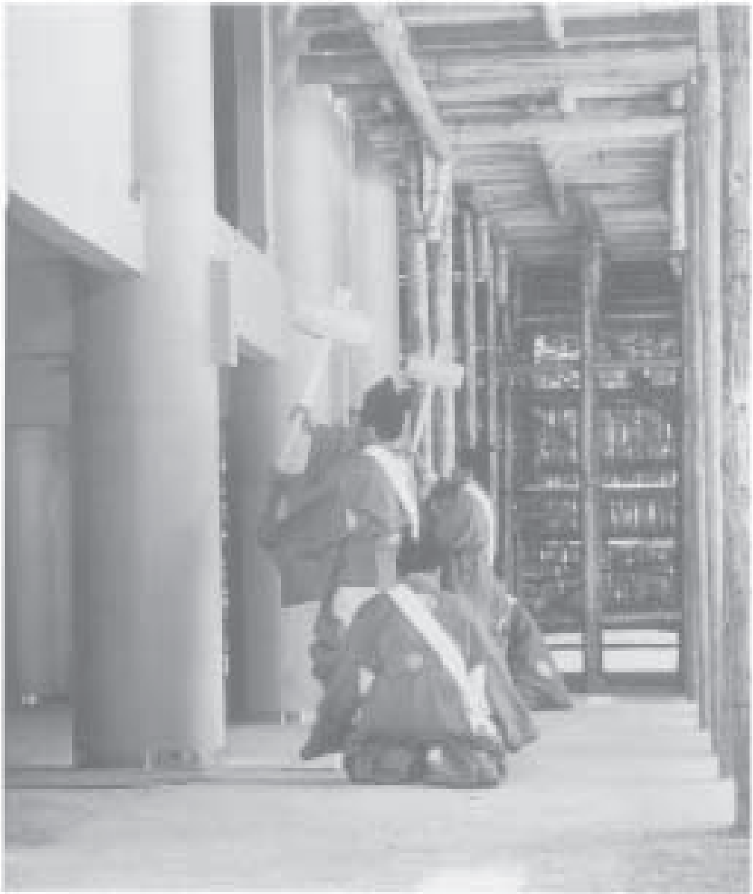
Fig 2.18 Ceremonial enactment of carpentry practice. The 'Pillar Erection Ceremony' ( Ritchu-sai ) for the Shoden of the Inner Shrine, March 31, 1992 (Courtesy of Ise Jingu)
