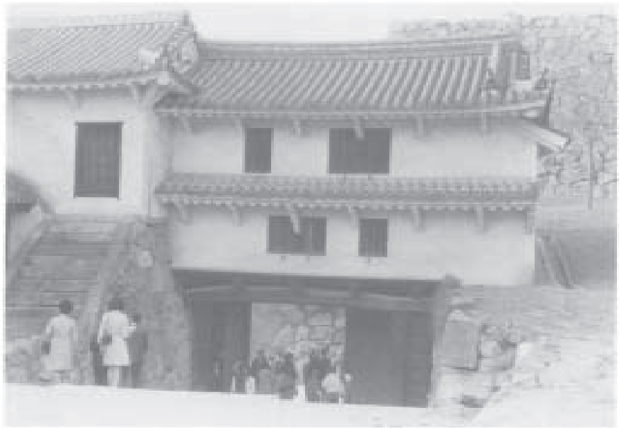
Fig 8.4 Himeji Castle, Hyogo prefecture. Two-storey gatehouse. Rear view
