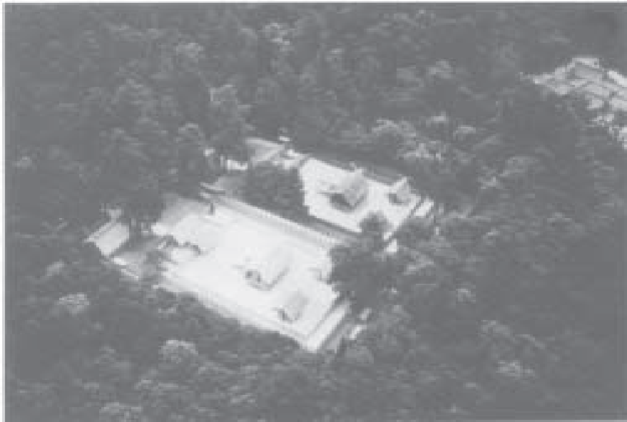
Fig 2.16 Aerial view of Inner Shrine, Ise, showing old and new shrines side side in 1992 prior to the dismantling of the structures built in 1965–73 (Courtesy of Ise Jingu)
