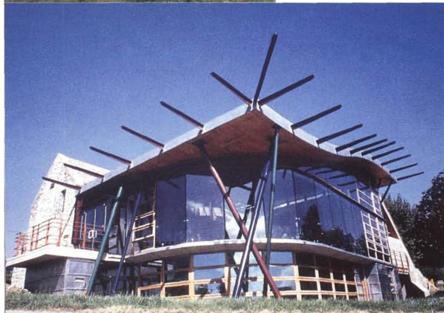
Fig. 4.12 Glass walls at St. Donat's Arts Centre (courtesy of Martin McCabe)
