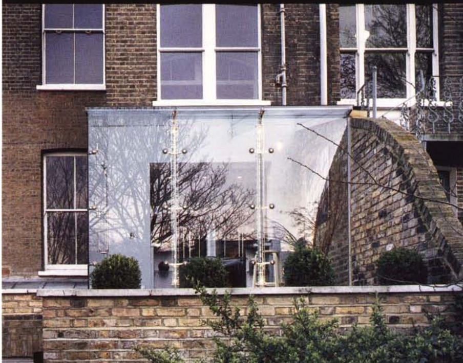
Fig. 8.2 Conservatory at a house in Clapham, South London (courtesy Bere Associates/Michael Heyward)
