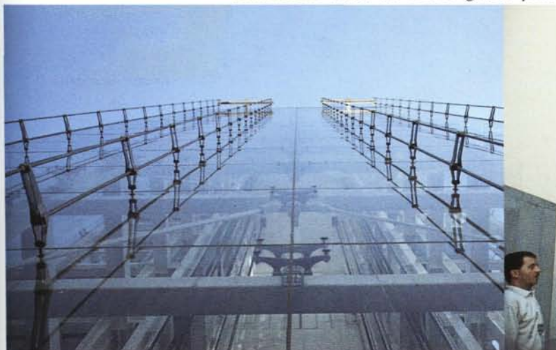
Fig. 4.8 Reina Sofia glass support structure (courtesy of Ove Arup & Partners/Bruce Gibbons)
