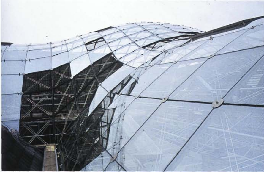
Fig. 4.19 Cutting and folding of panes (courtesy of Schlaich Bergermann)
