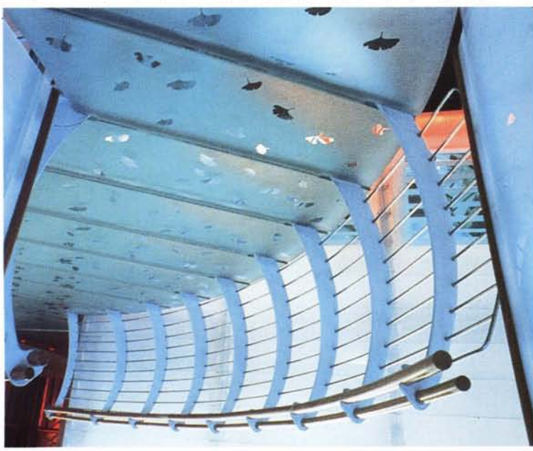
Fig. 13.9 Glass bridge in The Geological Museum, London (courtesy of Ian Ritchie Architects)
