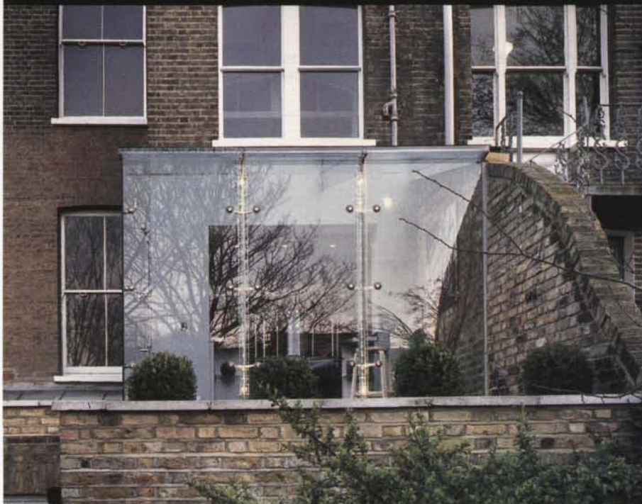
Fig. 8.2 Conservatory at a house in Clapham, South London (courtesy Bere Associates/Michael Heyward)
