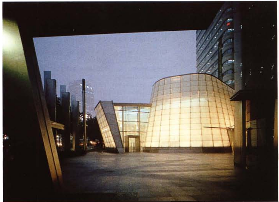
Fig. 8.4 The Rodin Pavilion at the Samsung Centre Seoul, South Korea (courtesy of Kohn Pedersen Fox, Tim Hursley)
