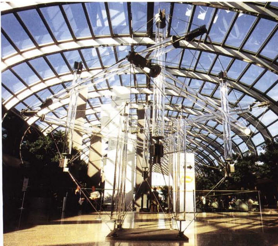
Fig. 10.4 Tensegrity structure at the Design Centre in Stuttgart (courtesy of Horst Schmeck)
