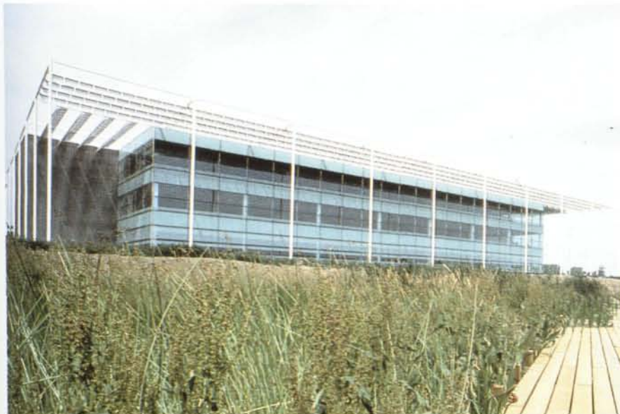
Fig. 2.12 Building B8 at Stockley Park, near London. (courtesy of Ian Ritchie Architects)
