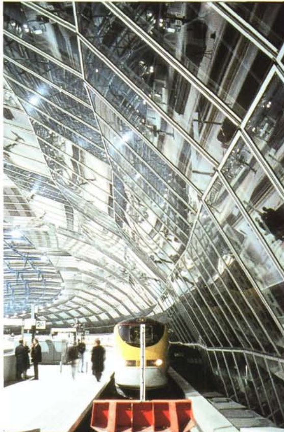
Fig. 2.25 Curved roof at Waterloo (courtesy of George Stowell)
