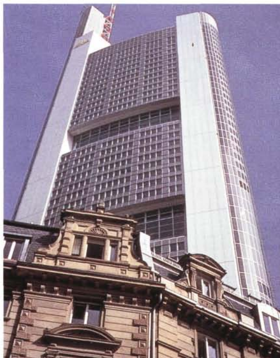
Fig. 2.3 The main legs of the Commerzbank, clad in glass (courtesy of Foster & Partners)
