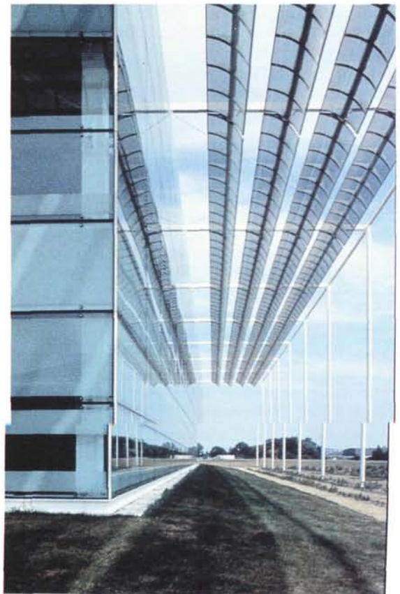
Fig. 2.31 Building B8 at Stockley Park, showing its external sunshades (courtesy Ian Ritchie Architects)
