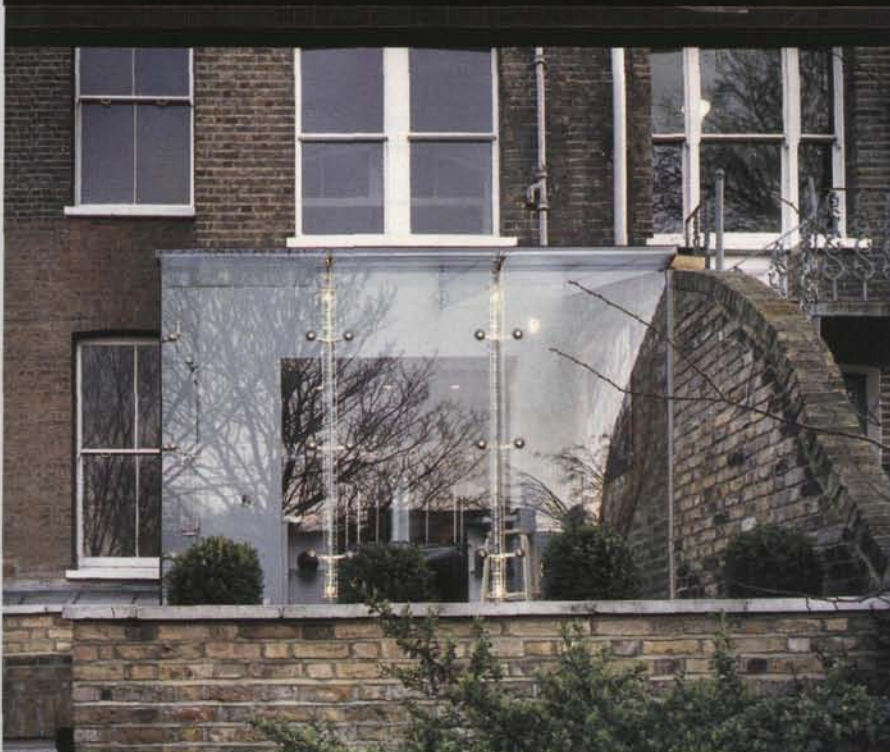
Fig. 8.2 Conservatory at a house in Clapham, South London (courtesy Bere Associates/Michael Heyward)
