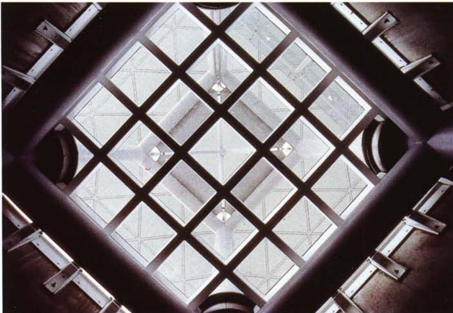
Fig. 13.1 Glass floors at Stansted (courtesy of Foster & Partners)
