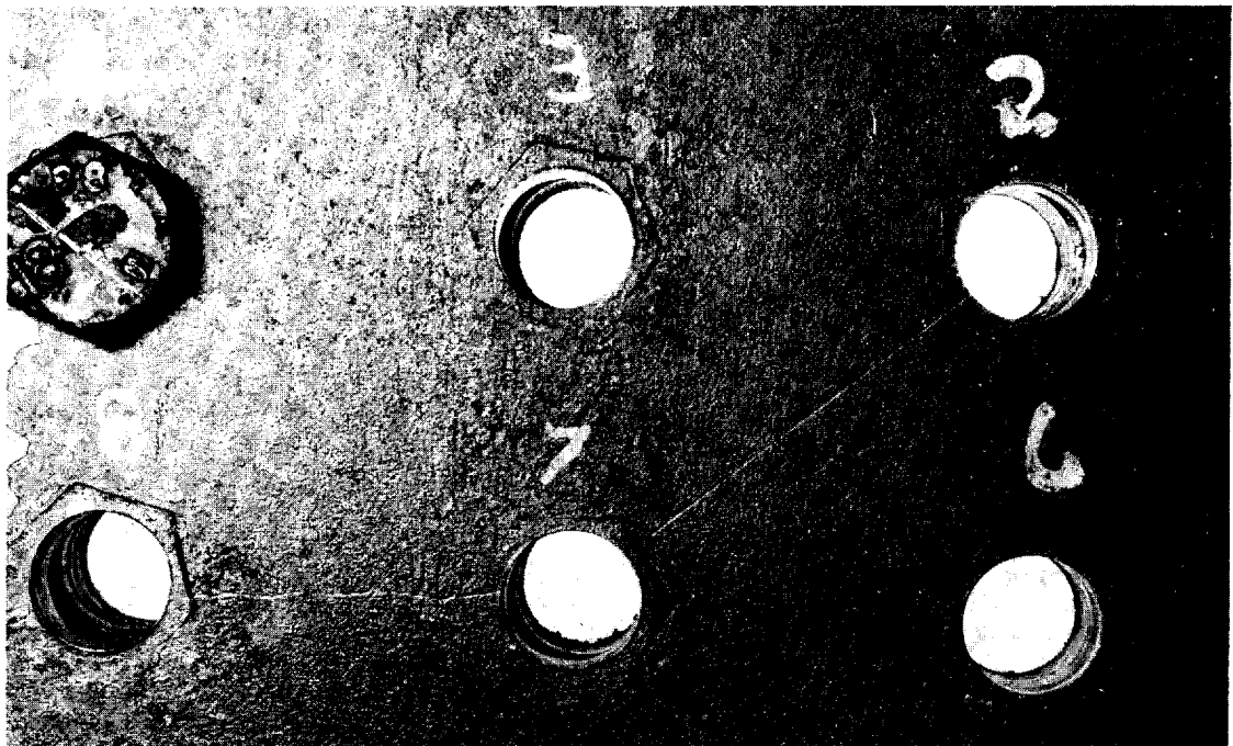
Figure 1.2 Part of bolted connection showing hole misalignment
