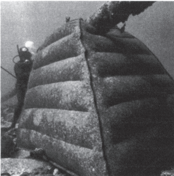
Figure 7.4 The construction of a pyramid-shaped pipeline support.
