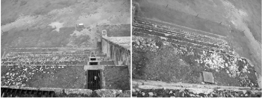
Fig. 7. a, left) Disregarding the natural distortion of the camera lens, it is evident how the platforms' borderlines do not run parallel, and do not recede accordingly in perspective as well; b, right) The same is true in this other view. Photographs by the author
