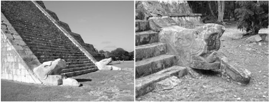
Fig. 11. a, left) Architects and laymen alike can notice the wrong way in which the serpent heads were placed in Kukulcán's stairway; b, right) In contrast, the dexterous stonework of the Osario Pyramid's serpent heads, well integrated to the balustrades, makes evident the erroneous placement of those of Kukulcán. Photographs by the author
