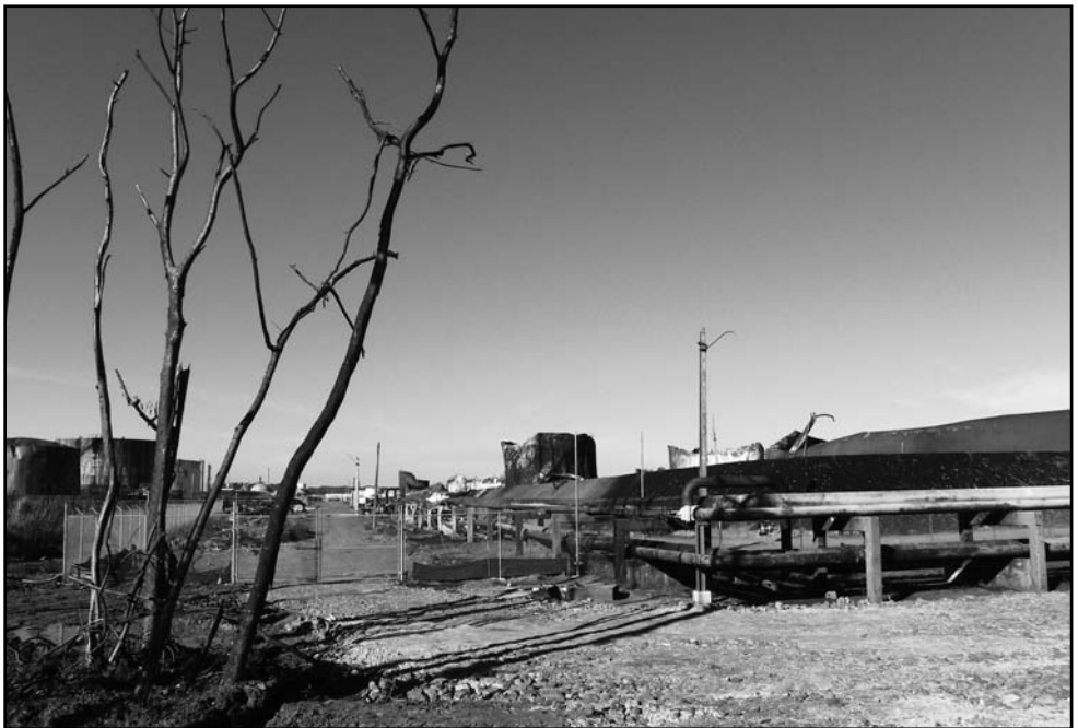
CAPECO facilities after a massive explosion in Cataño, Puerto Rico (@Eddie N. Laboy-Nieves)
