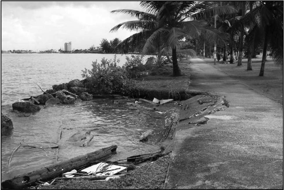
Coastal erosion in Cataño, Puerto Rico (@Eddie N. Laboy-Nieves)
