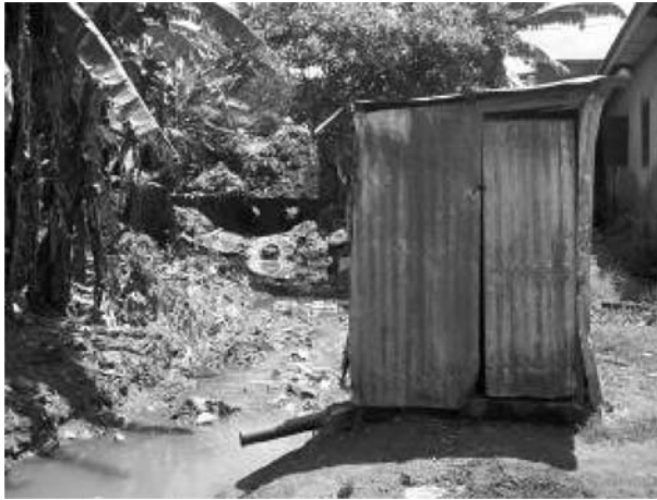
Figure 15.5 Latrine equipped with an overflow pipe.
