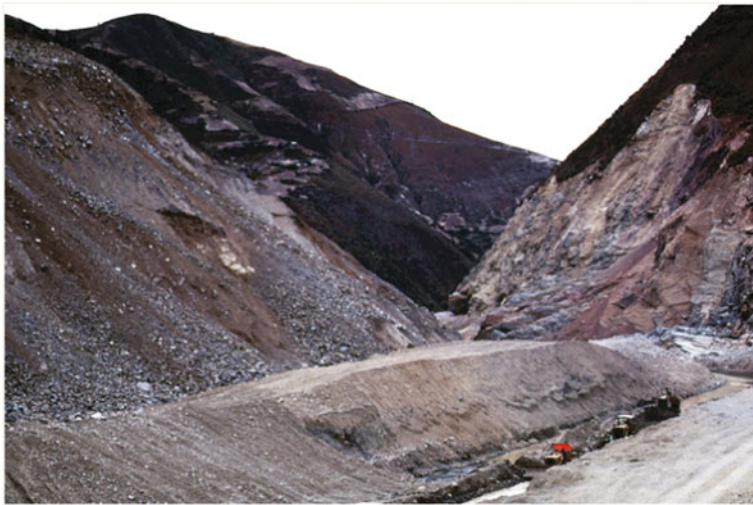
Fig. 3.16 Excavation of a new channel in the landslide mass after the May 1st, 1993 overflow. The unstable left slope that required a stabilizing scheme can be observed
