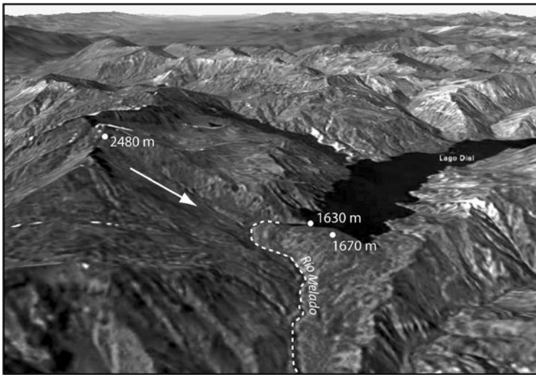
Fig. 24.8 Oblique view of the rock-avalanche deposit impounding Laguna Dial, Chile ( 36^{\circ} 25' 14'' S / 70^{\circ} 55' 28'' W ; Google Earth). This rock avalanche forms a single dam in a stretched valley (type II). The cross valley profile has asymmetric distribution of the landslide deposit overlying an apparent symmetric valley floor (type ii). This is a narrow mountain valley and direction of landsliding is normal to the thalweg, the dip of the thalweg is minor, therefore the run out is restricted and the landslide forms a massive thick deposit (type 2)
