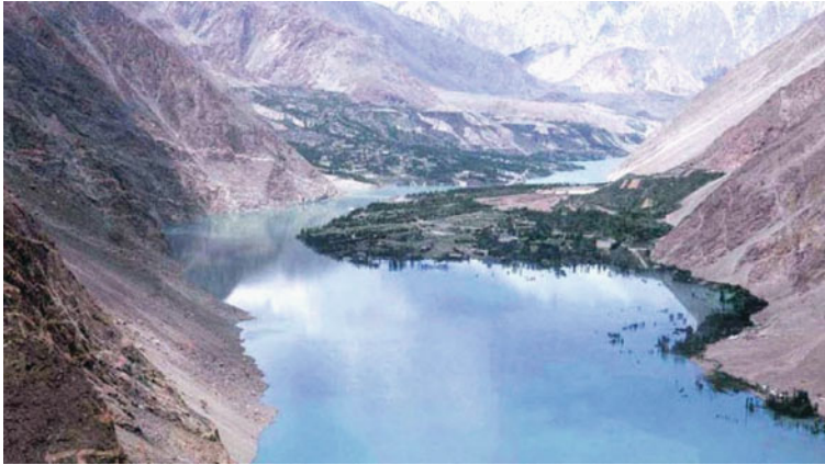
Fig. 2.1 Flooding in the Hunza Valley, northern Pakistan due to the filling of the rockslide-dammed lake impounded behind the Attabad rockslide which blocked the Hunza River on January 4, 2010 [23]. Lake waters submerged several villages, vast areas of agricultural lands adjacent to the Hunza, and 22 km of the Karakoram Highway. Photograph taken on May 28, 2010, a day before overtopping of rockslide dam ( Pakistan Tribune photograph)
