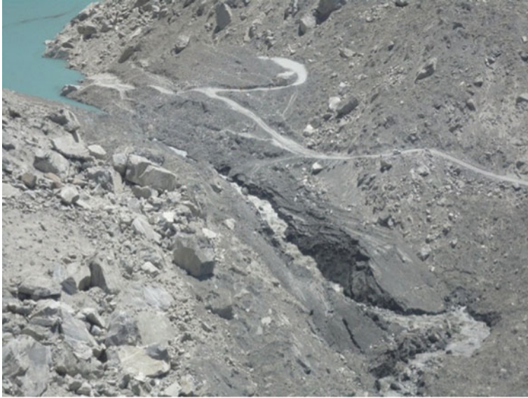
Fig. 2.19 Spillway in Attabad rockslide debris, shortly after overtopping began on May 28, 2010. Note vertical erosion of spillway and retrogression of “knickpoint”. As of July 25, 2010 (200 days after impoundment) stable overtopping continues with lake level more or less unchanged [Photograph courtesy of Focus Humanitarian, Pakistan]
