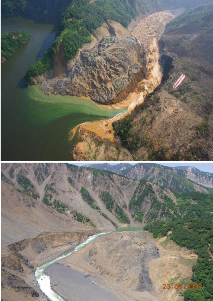
Fig. 10.14 Tangjiashan rockslide-dammed lake during and after partial drainage on June 10, 2008. Upper picture (view downstream) shows the incised channel over the debris caused by water release from Tangjiashan lake through the sluceway (photograph from Prof. Liu Ning). Lower photograph (view upstream) is an overview of new channel after water release from Tangjiashan landslide lake (photograph is provided by Water Resources Bureau of Mianyang city)
