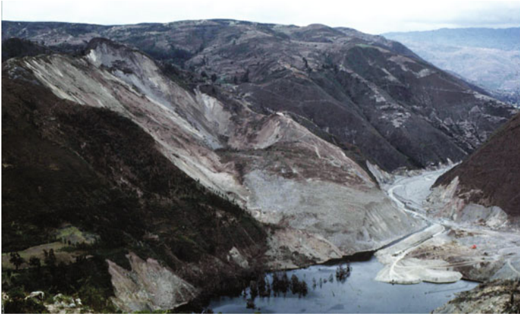
Fig. 3.15 View of the La Josefina landslide dam, some months after breaching. A deeper artificial channel was excavated to decrease the level of the residual lake
