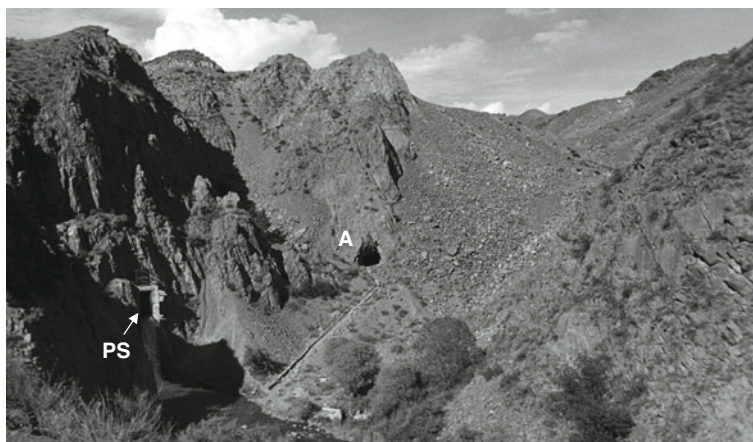
Fig. 26.1 The Burlykia experimental blast-fill dam. A – adit at the base of the right slope that was made to investigate seismic effect of the explosion on the underground structures. PS – permanent spillway. View from downstream
