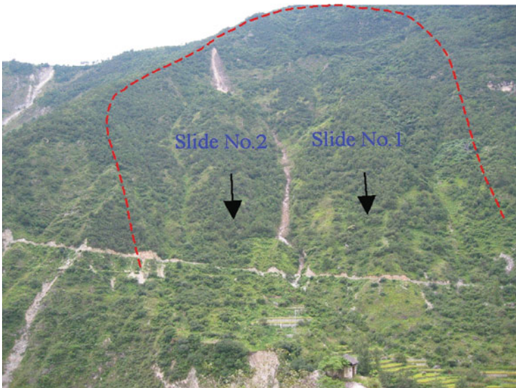
Fig. 13.6 Photograph showing the landslide site (view is to the west). The failure main scarp is marked with a dashed line and the location of the site shown in Fig. 13.4
