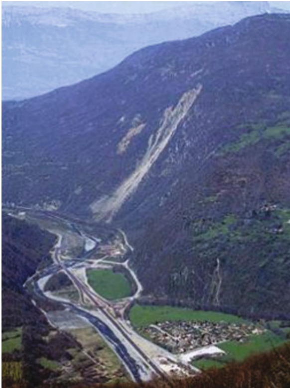
Fig. 3.17 Zone of impact of the Séchilienne rockfall
