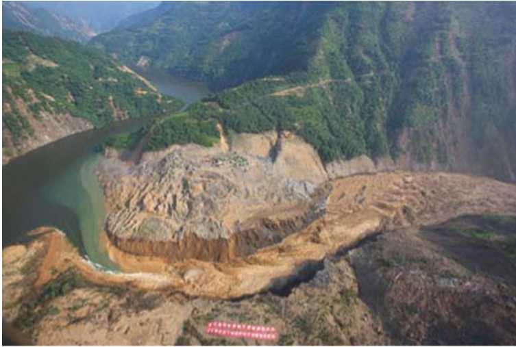
Fig. 2.18 Controlled breaching of Tangjiashan Lake, Sichuan, China taking place on June 10, 2008
