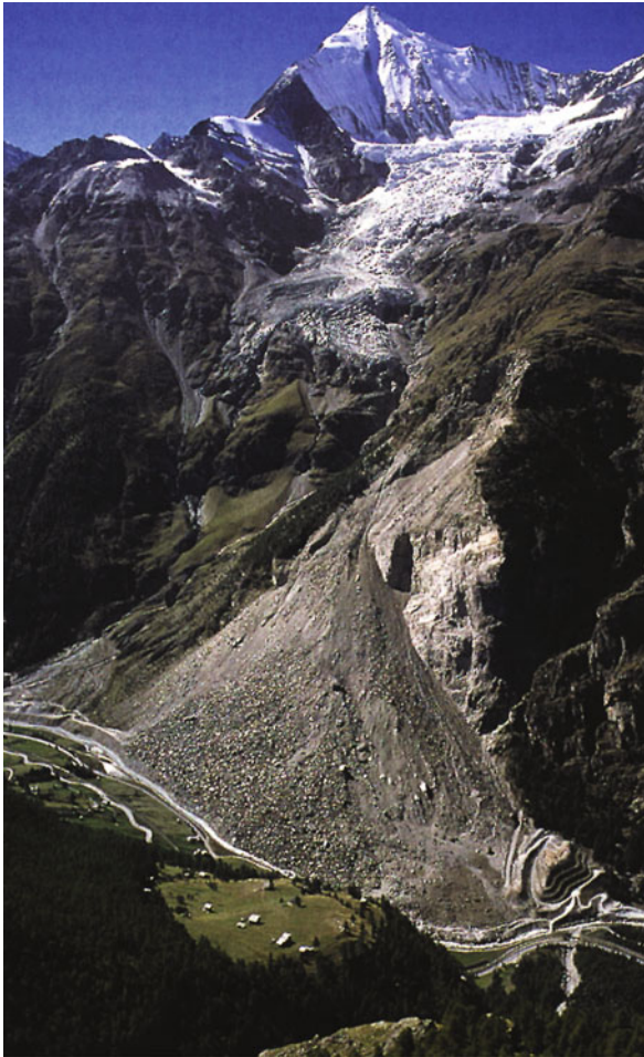
Fig. 3.11 General view of the Randa rockfall causing the damming of the Vispa River. The mitigation works have been already carried out
