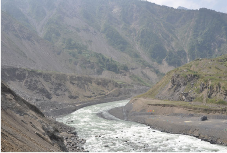
Fig. 10.15 Tangjiashan Lake: upstream view of the armoured spillway channel bed 15 months after risk reduction operation (Photograph taken on September 22, 2009)
