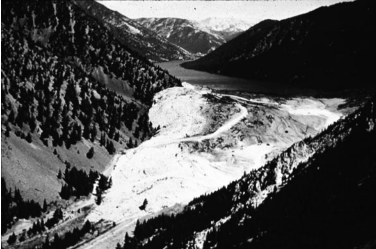
Fig. 2.3 The landslide dam formed by the 1959 earthquake-induced Madison Canyon rock slide, Montana, USA, and Earthquake Lake, which it impounded (Photo by J.R. Stacey, US Geological Survey)
