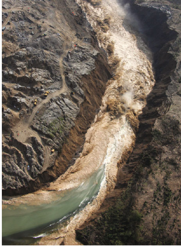
Fig. 1.22 Aerial view of flow in Tangjiashan spillway at about 9 a.m. June 10, 2008, during controlled partial drainage/breaching of rockslide dam. Discharge is approximately 2,000 \text{ m}^3/\text{s} . Note effects of spillway erosion and construction machinery for scale (photograph by Xinhua News Agency, China)
