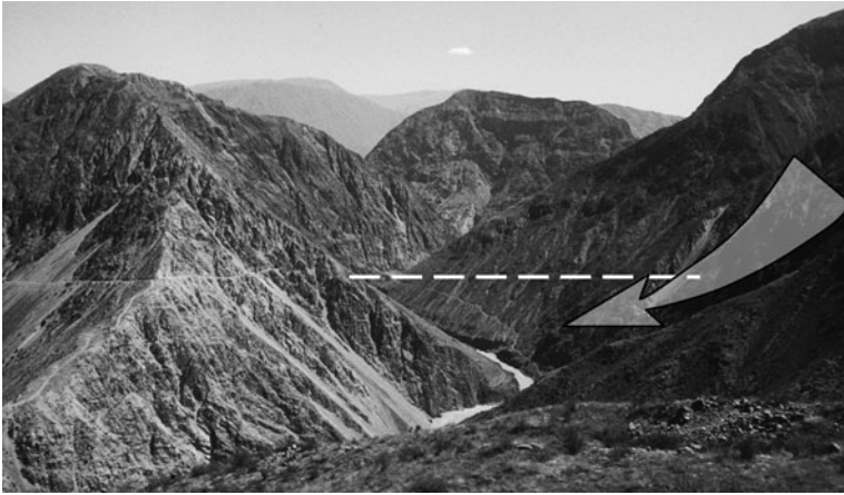
Fig. 25.20 The Kambarata-1 dam site. Dashed line corresponds to the designed dam crest; arrow shows the direction of rock sliding
