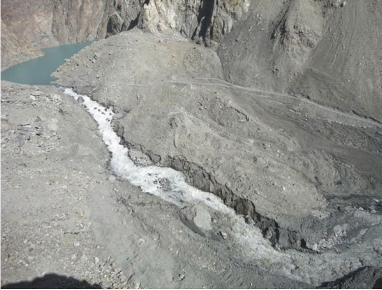
Fig. 1.26 View of spillway over the Attabad rockslide dam on June 14 (Day 159 of impoundment) as stable overflow continued after the May 29 overtopping. Hunza rockslide-dammed lake is visible in the left background (Photograph courtesy of Focus Humanitarian Assistance, Pakistan)
