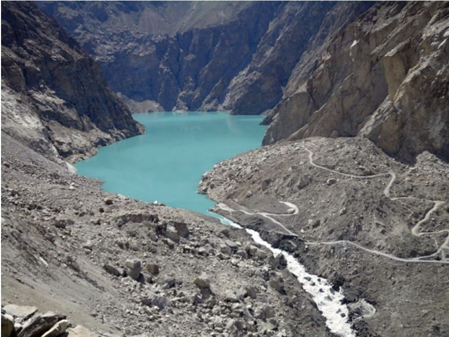
Fig. 7.15 View of overflow of 2010 Attabad rockslide dam and the Hunza rockslide-dammed lake in the background. Date of photograph is June 10, 2010 12 days after overtopping on May 29 (143 days after impoundment). Volume of lake is ca. 430 Mm 3 . Note limited erosion of spillway. Photograph by Focus Humanitarian Assistance, Pakistan
