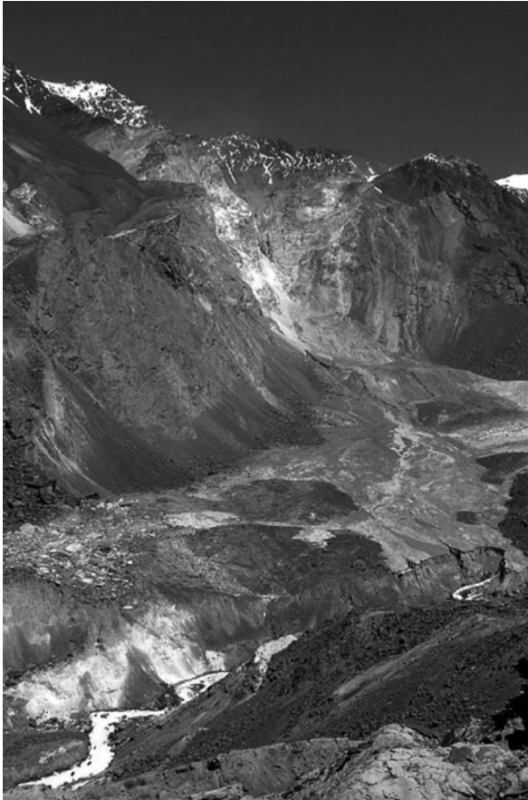
Fig. 16.6 Helicopter view of the downstream side of the Usoi Dam, debris flow and canyon (photo A. Ischuk, 2004)
