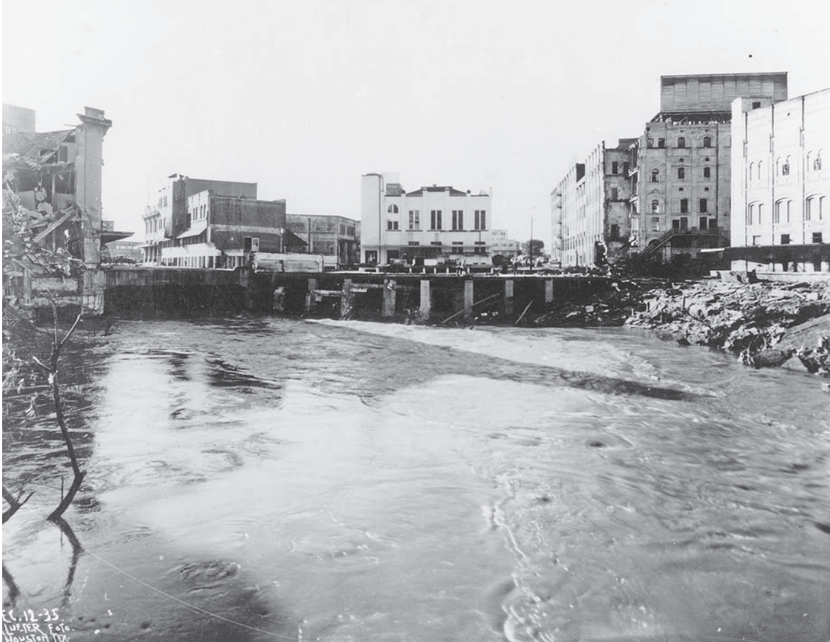
Flood damage, Buffalo Bayou, 1935. Showing the aftermath of the disastrous flood of December 1935, this photo clearly conveys the degree to which Houston was largely at the mercy of natural forces until the channelizing and concreting of local waterways was completed by the mid-twentieth century. (MSS 157-1095, Courtesy HMRC, Houston Public Library.)
