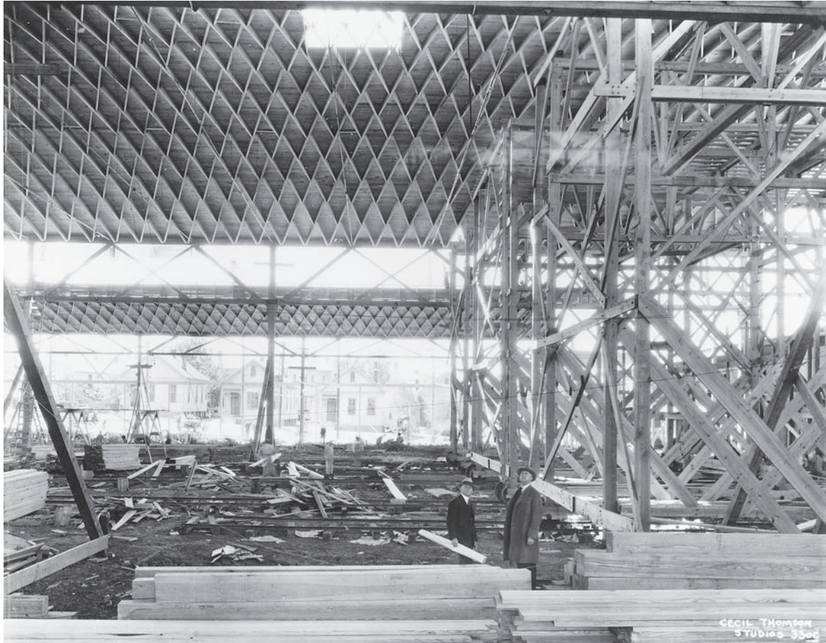
Jesse H. Jones (right), the Houston businessman responsible for ensuring that Houston was selected as the site of the 1928 Democratic National Convention, personally inspects the Convention Hall's lamella roofing during construction. Jones would later become the head of the Reconstruction Finance Corporation during the Great Depression and secretary of commerce in Franklin Roosevelt's cabinet. The middle-class housing that still occupied much of the present-day downtown area can be seen in the background. (MSS 157-358, Courtesy HMRC, Houston Public Library.)
