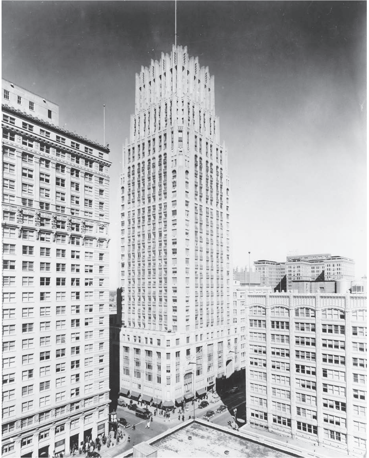
The selected design for the Gulf Building, shown after completion in 1929. The Gulf Building was one of several 1920s skyscrapers inspired by Eero Saarinen's second-place design in the competition to design a new headquarters for the Chicago Tribune. Designed by Finn with the assistance of Kenneth Franzheim and J. E. R. Carpenter, the Gulf Building is widely acknowledged as an Art Deco masterpiece. Today it is known as the J. P. Morgan Chase Tower. (MSS 19-924, Courtesy HMRC, Houston Public Library.)
