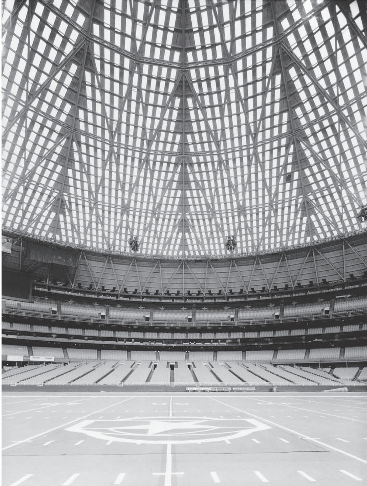
Interior view looking south toward moveable field-level seats, ca. 2003. (SC 1433-12, Courtesy HMRC, Houston Public Library.)
