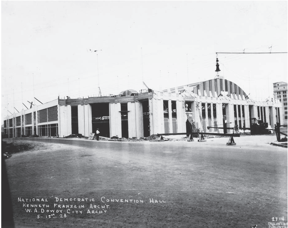
The nearly completed Convention Hall, May 12, 1928. W. A. Dowdy, who is listed as an architect along with Kenneth Franzheim on the lower left of the photo, served as the architect for the City of Houston and acted as on-site consultant during construction. (MSS 100-94I, Courtesy HMRC, Houston Public Library.)
