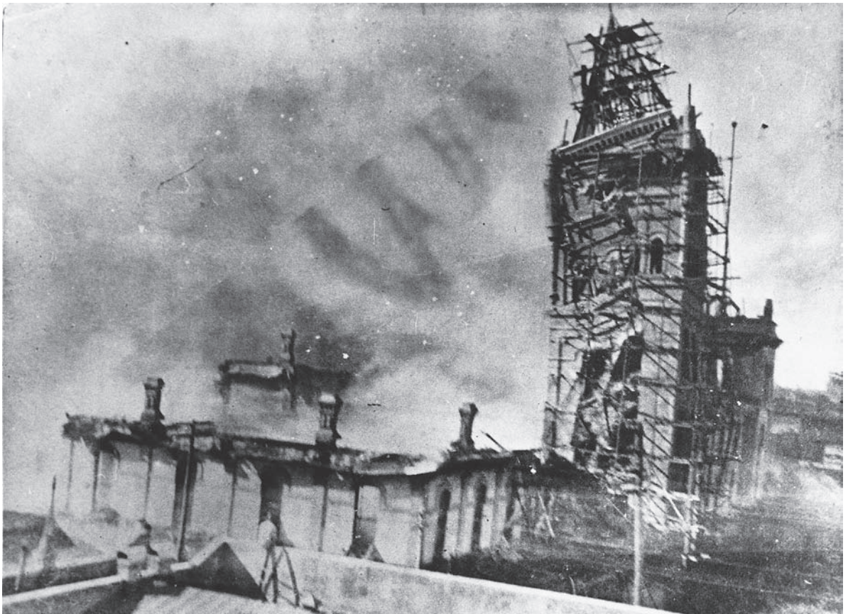
A photographer captured the City Hall's east tower as it collapsed during its demolition in 1948. Structural problems led to the demolition of both towers that year. When the remainder of the building was finally demolished in 1962, the outdated architecture, combined with the building's generally run-down appearance, was considered an eyesore by most Houstonians at the time, an outmoded reminder of a bygone era. (MSS 157-218R, Courtesy HMRC, Houston Public Library.)
