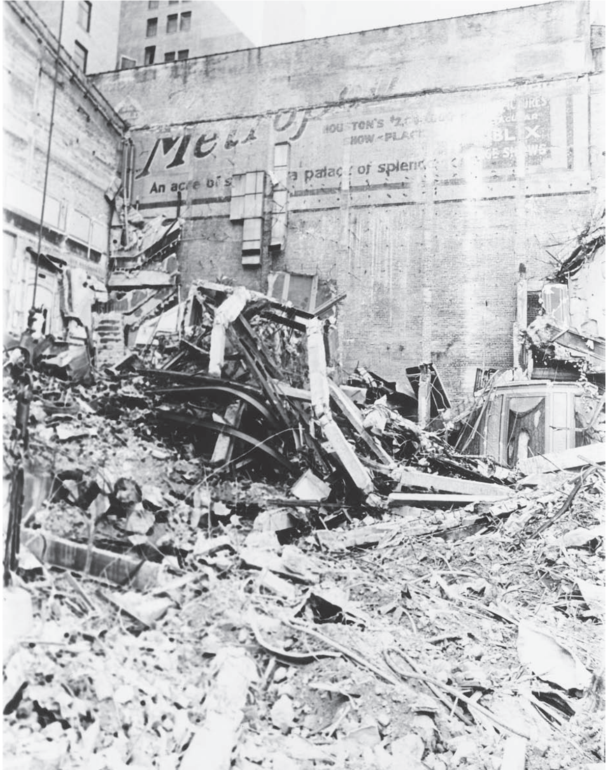
All that remained of the beautiful Loew's Theatre following its demolition in August 1973. An advertisement for the Metropolitan can still be seen on one of the remaining walls behind the piles of rubble and scrap metal. All of Houston's "big three" movie palaces suffered the same fate. (RG D6, Courtesy HMRC, Houston Public Library.)
