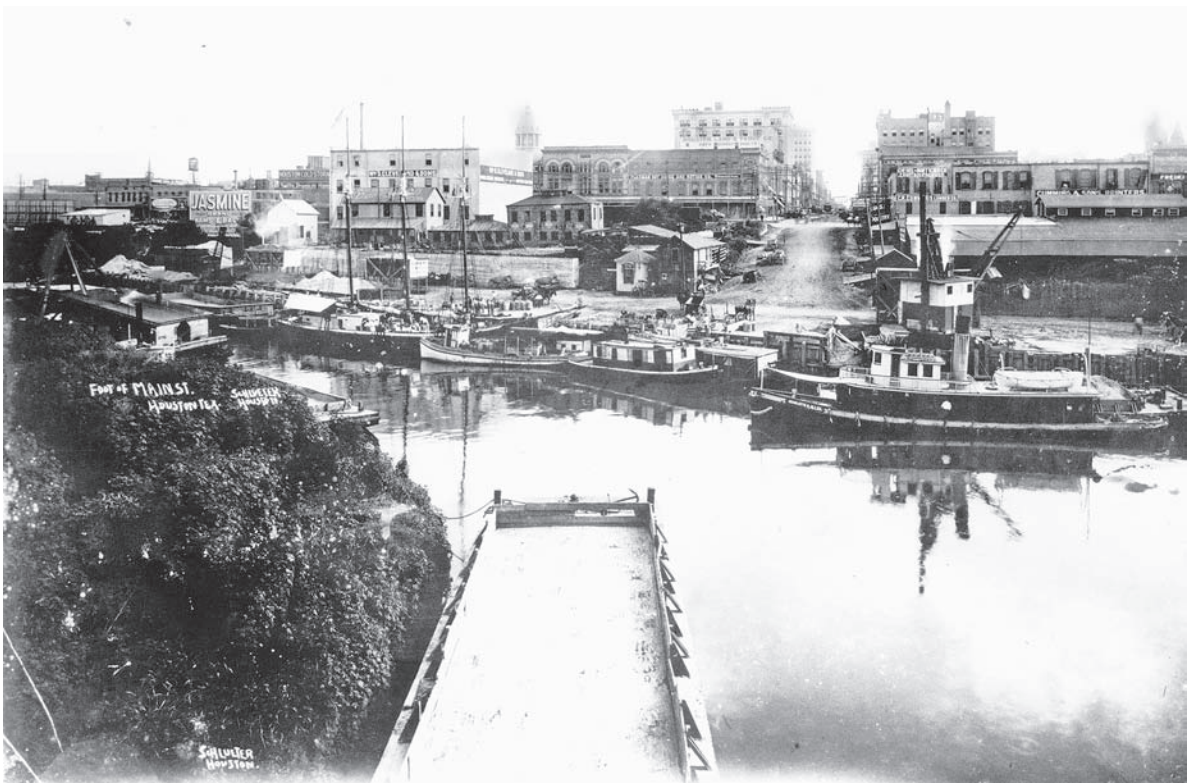
Main Street at Buffalo Bayou, 1910. This is another photograph by Frank Schlueter, showing the foot of Main Street at Buffalo Bayou. Because this port scene was photographed prior to the completion of the Houston Ship Channel in 1914, with the exception of some of the newer buildings in the background, it looks scarcely different than it would have at the time of the Civil War. (MSS 157-58, Courtesy HMRC, Houston Public Library.)
