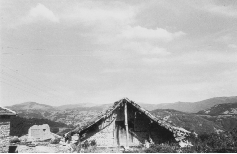
Figure 10.5 KOSHARA. A FOUNDING SHELTER FOR THE MYTH OF THE ORIGIN OF THE VILLAGE OFFERS A PRIMORDIAL TEXTURE TO LAUGIER'S PRIMITIVE HUT.
