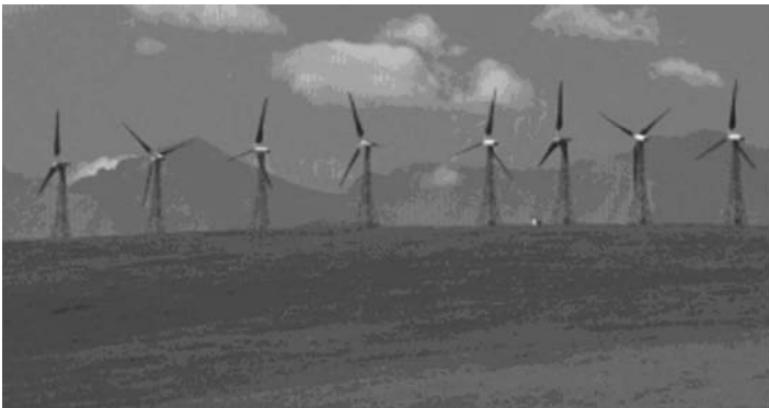
FIGURE 12.3 Big Wind Farm. 5
