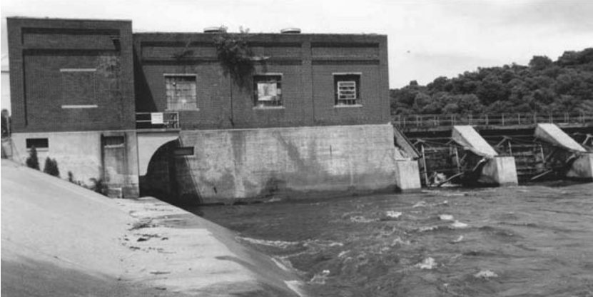
FIGURE 12.19 Fort Dodge Powerhouse and Mill Dam Gates, Fort Dodge, Iowa.
