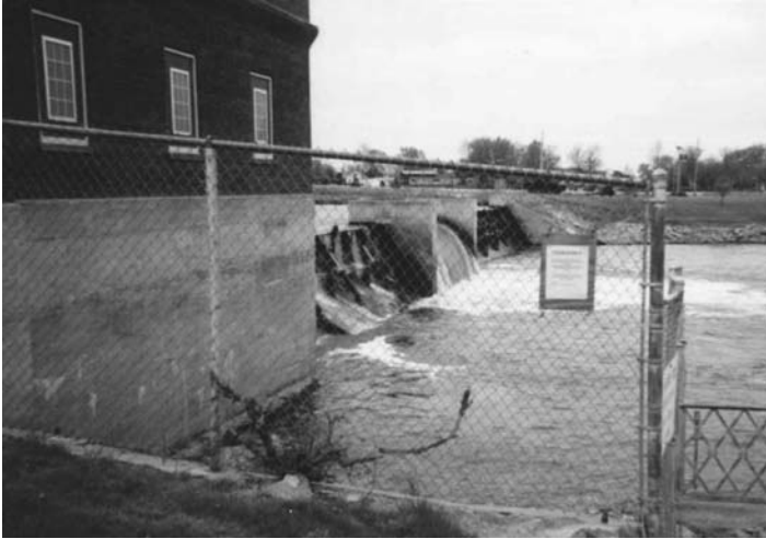
FIGURE 12.14 Nashua Mill Dam and Powerhouse, Nashua, Iowa.
