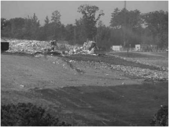
FIGURE 6.3 Trash Loaded and Compacted into a Landfill. 9
