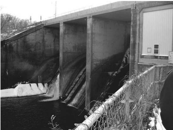
FIGURE 12.15 Delhi Mill Dam and Spillway, Delhi, Iowa.
