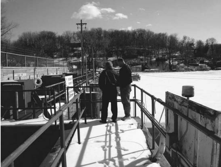
FIGURE 12.16 Delhi Mill Dam and Facility, Delhi, Iowa.
