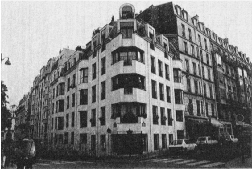
Plate 4.11 Paris: block of flats, rue Descartes
