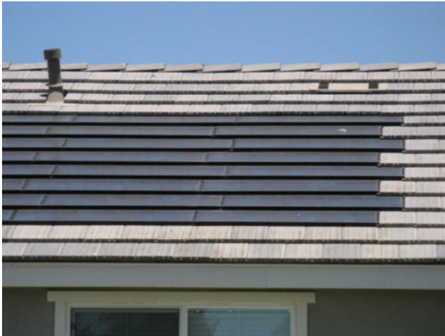
FIGURE 33-5 Building-integrated photovoltaic roof tiles.
