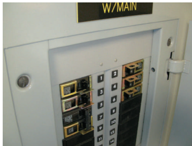
FIGURE 1-3 A lock-off accessory that can be added to circuit breakers allows for adding a padlock and tag to individual circuit breakers in a panelboard.
