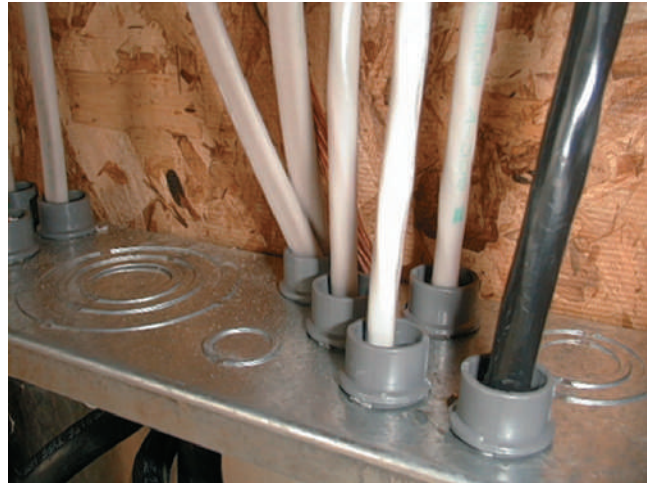
FIGURE 4-21 Individual connectors that are listed for the cable are used to connect the cables to the cabinet.
