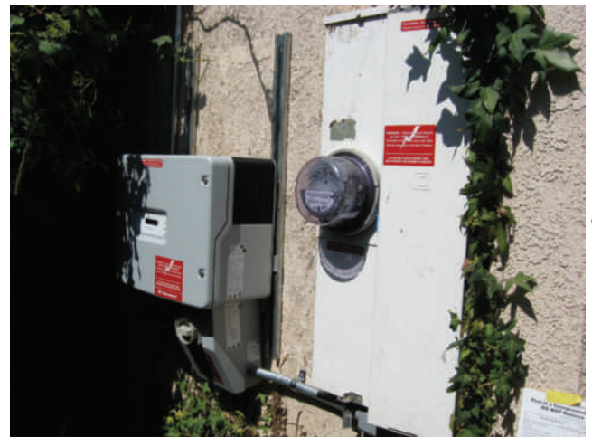
FIGURE 33-4 A residential utility-interactive inverter.
