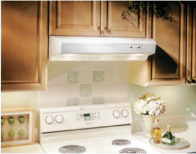
FIGURE 12-6 Typical range hood exhaust fan. Speed control and light are integral parts of the unit.
