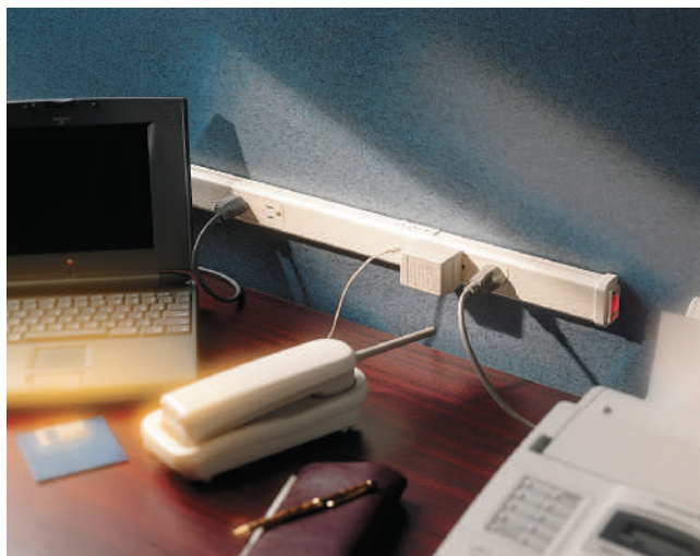
FIGURE 18-16 A typical metal multioutlet assembly. Multioutlet assemblies are permitted to be run through (not within) a dry partition when no outlets are located within the partition, and all exposed portions of the assembly can have the cover removed. Nonmetallic multioutlet assemblies are also available.
