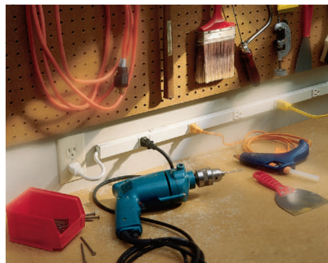
FIGURE 18-18 A cord-connected, prewired multioutlet assembly installed above a workbench.
