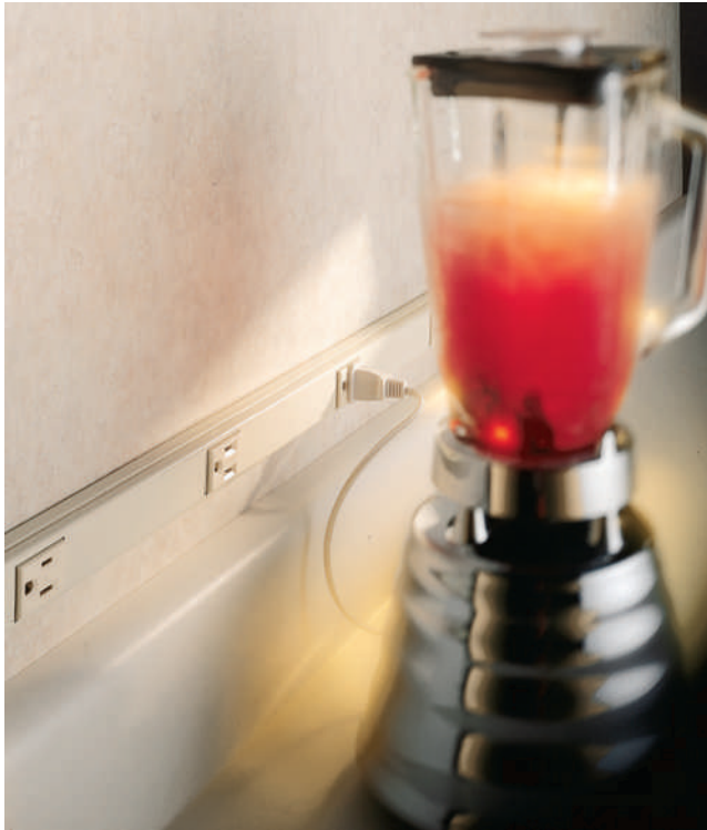
FIGURE 18-19 A multioutlet assembly installed above the backsplash of a kitchen countertop.
