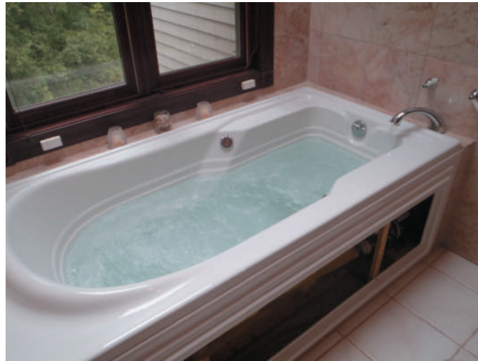
FIGURE 22-12 A typical hydromassage bathtub, sometimes referred to as a whirlpool.
