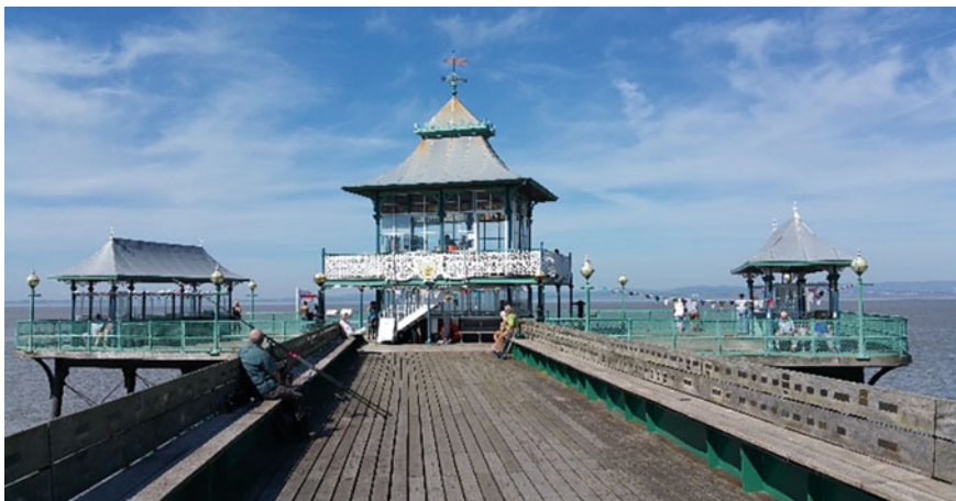
Fig. 6 New central pavilion in the end of the wharf (González-García de Velasco, Agudo Martínez y González Vilchez 2016)
