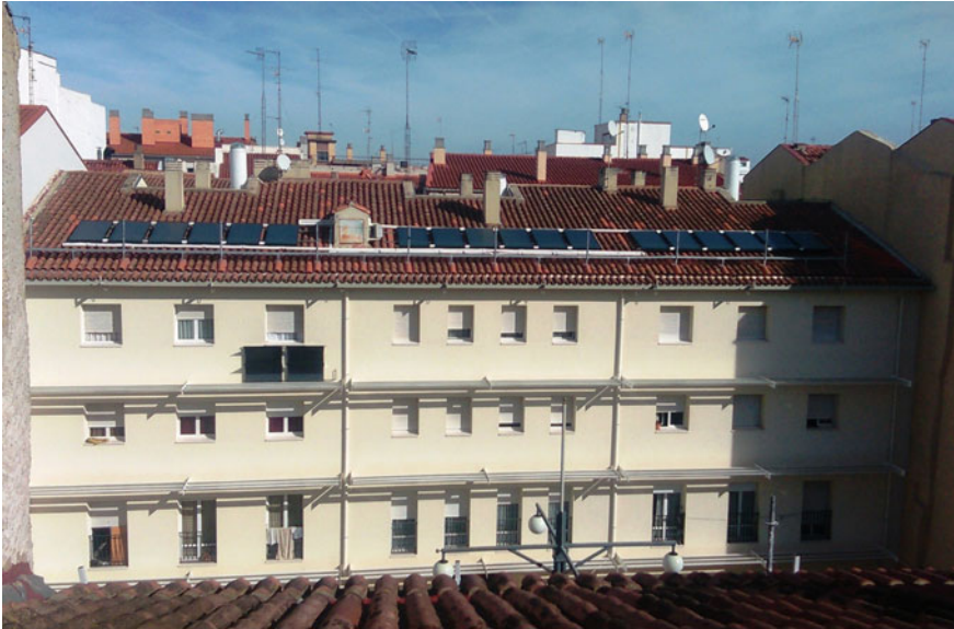
Fig. 7 Building A after intervention facade insulation, incorporation of sunscreen, hybrid solar panels for hot water and electricity, solar lighting conduits for patios and prototype passive solar heating
