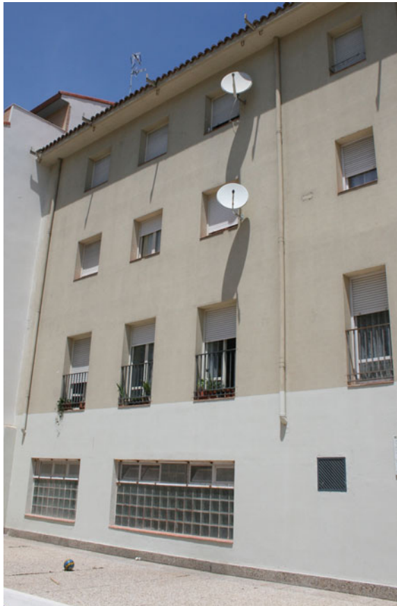
Fig. 3 South facade before renovation. October noon
