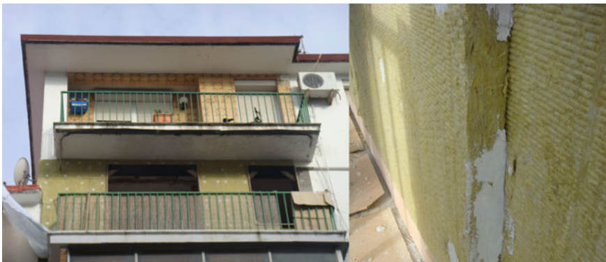
Fig. 1 Image of the facade of the house during construction
