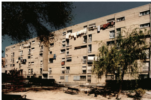
Fig. 1 Caño Roto social housing project. Original (1994) and rehabilitated conditions (2015). Sources CREA Arquitectos file and author’s photograph
