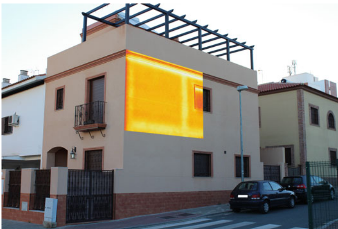
Fig. 1 Building for Model 2 with thermogram overlap
