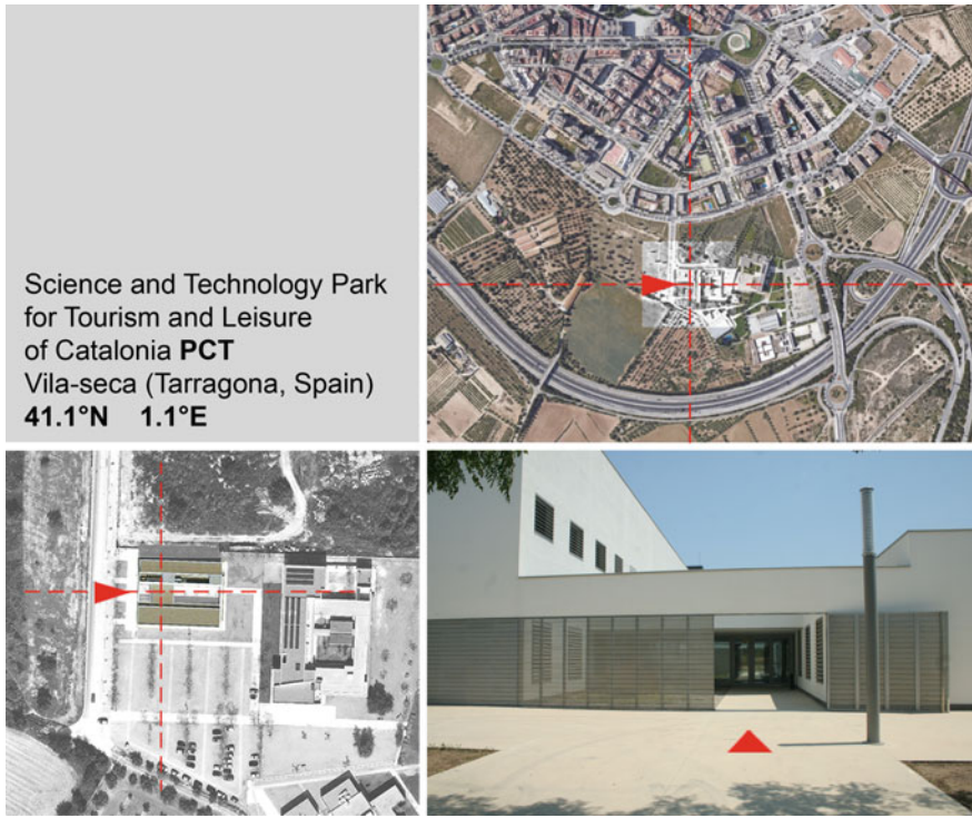
Fig. 1 Situation of the building and entrance view
