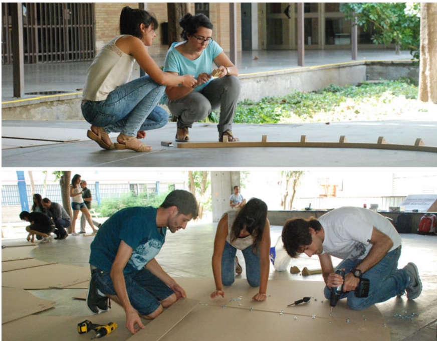
Fig. 3 SSFS Pavilion-Fablab Sevilla assembly test in ETSIE building, and Fablab Sevilla
