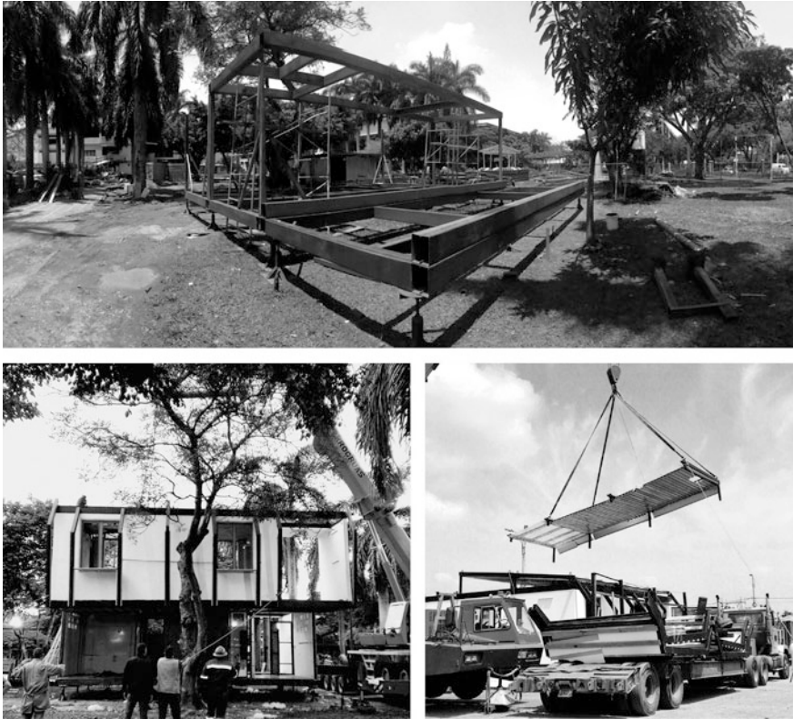
Fig. 7 Module room-cell building, relocation and assembly in Villa Solar
