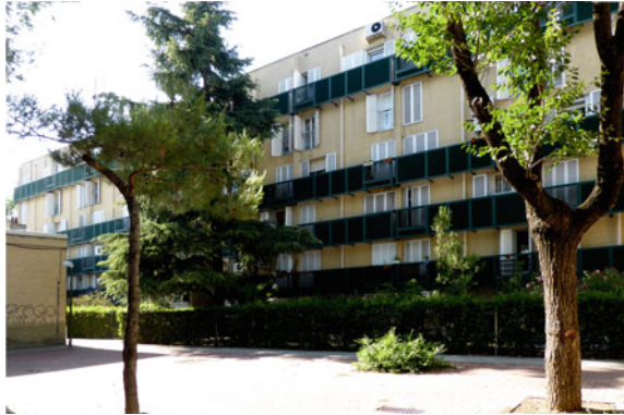
Fig. 2 Caño Roto social housing project. Original (1994) and rehabilitated conditions (2015). Sources CREA Arquitectos file and author's photograph
