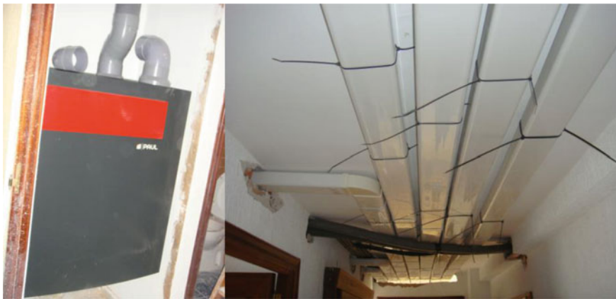
Fig. 3 Air heat recovery and duct system
