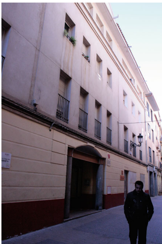
Fig. 2 North facade of the building in San Pablo St.
