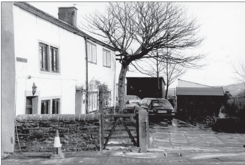
Figure 2.15 The proximity of the tree to the cottage should be of clear concern to any surveyor and a justifiable reason for recommending further investigations.
