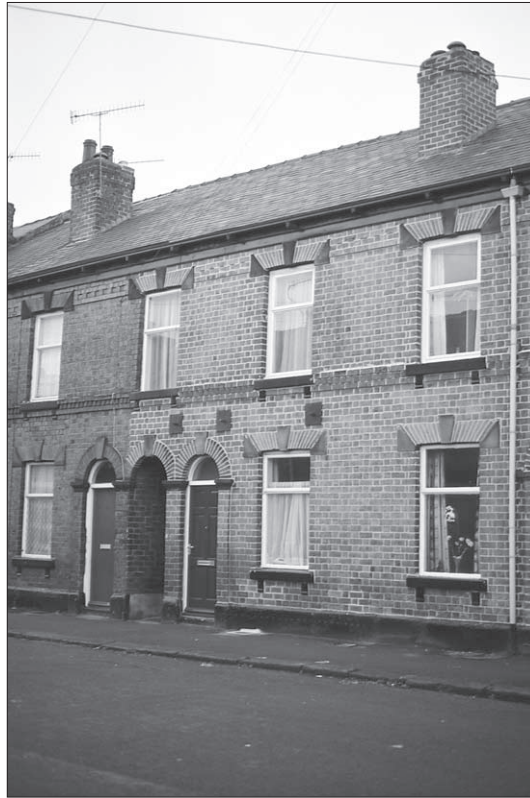
Figure 4.16 External restraint plates to these terrace properties clearly indicates the possibility of lateral instability.
