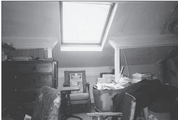
Figure 7.11b An internal view of one of the new roof windows. The purlin has been cut through so the window could be fitted. The vertical posts supporting the ends of the purlins are supported off the existing floorboards and floor structure. Little surprise the roof covering is uneven!
