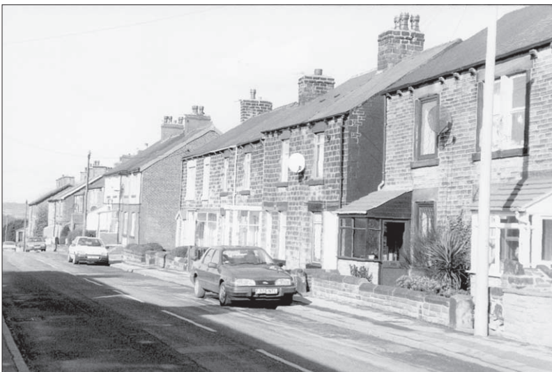
Figure 2.14 Properties in one street in a similar condition.
