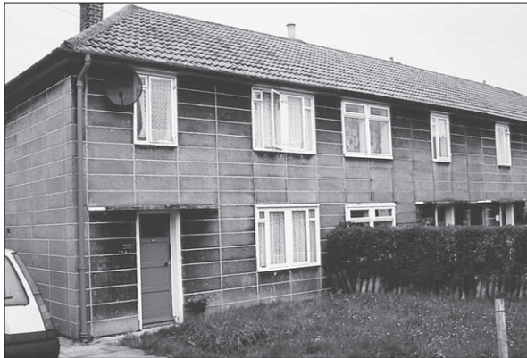
Figure 12.2 Unity house. This type is faced externally with concrete panels.
