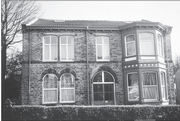
Figure 7.11a The roof to this dwelling has been affected by roof spread. Based on the external visual clues, the likely causes are heavier replacement concrete tiles and the installation of the roof windows.
