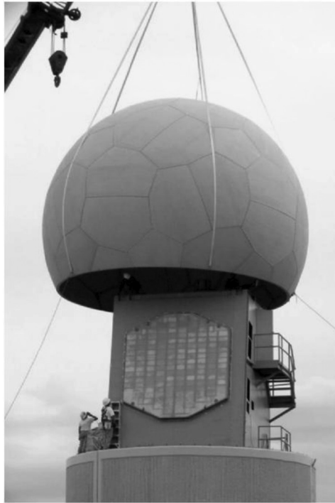
FIGURE 5.5 Phased-array radar antenna of the National Weather Radar Testbed (NWRT) comprising 4352 components used to electronically steer the beam. (Figure courtesy of Zrnić et al. 2007).
