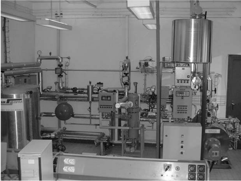
Fig. 6.15 The steam generator installation
