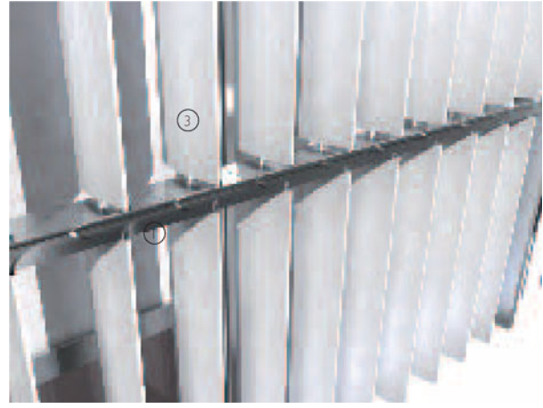
3-D detail view of frame supported metal louvres used as a shading device in front of glazed curtain wall
