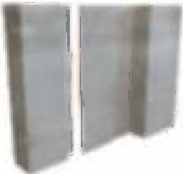
Internal concrete wall
