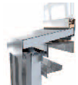
3-D view and exploded axonometric of window head detail
