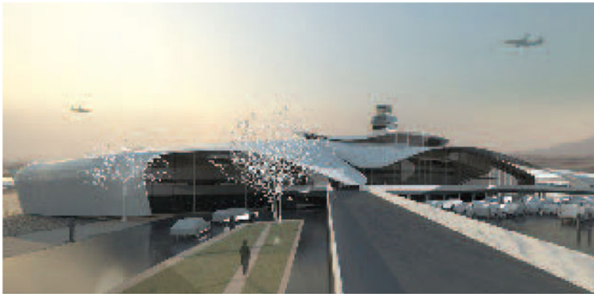
Envelope option of rainscreen cladding panels on a continuous waterproof metal deck. The design is based on prevailing wind movement across the site.
