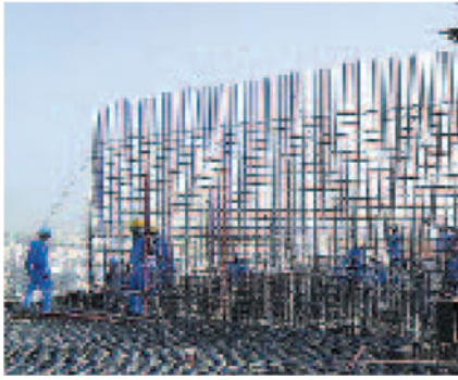
Setting reinforcement
