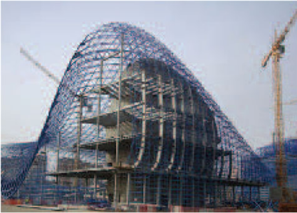
Triangulated roof structure to which envelope system is fixed
