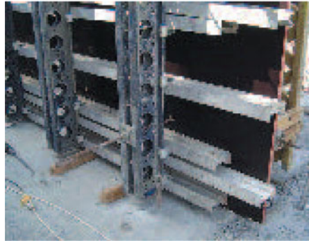
Securing formwork
