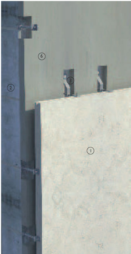
3-D view of stone carrier system made from individual fixings
