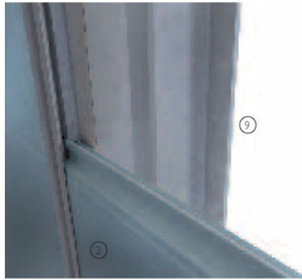
3-D view of framework supporting composite panels interlocking horizontally with vertical capping piece
