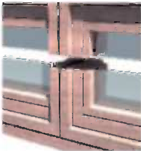
3-D view of vertical sliding sash window
