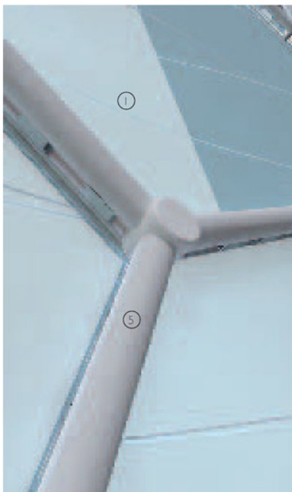
3-D detail of junction between ETFE cushions
