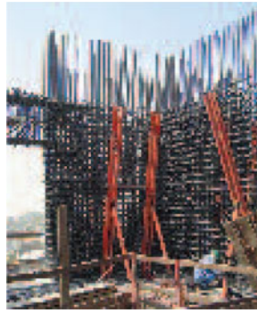
Setting up formwork
