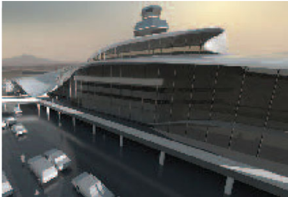
Envelope option of rainscreen cladding panels on a continuous waterproof metal deck. The design is based on prevailing wind movement across the site.
