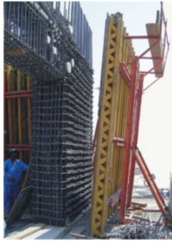
Setting up formwork
