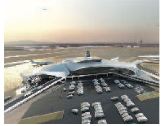
Envelope option of rainscreen cladding panels on a continuous waterproof metal deck. The design is based on prevailing wind movement across the site.
