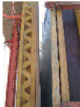
Setting up formwork
