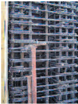
Setting up plywood formwork
