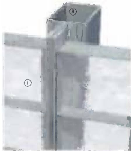
3-D view of connection between glass blocks supported by steel box frame
